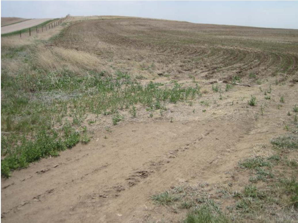
Figure 3: View to the south from the north end of the project corridor (Image 5).
