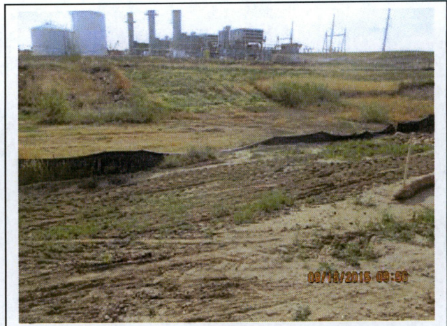
2. West of pond, silt fence overwhelmed and knocked down.
