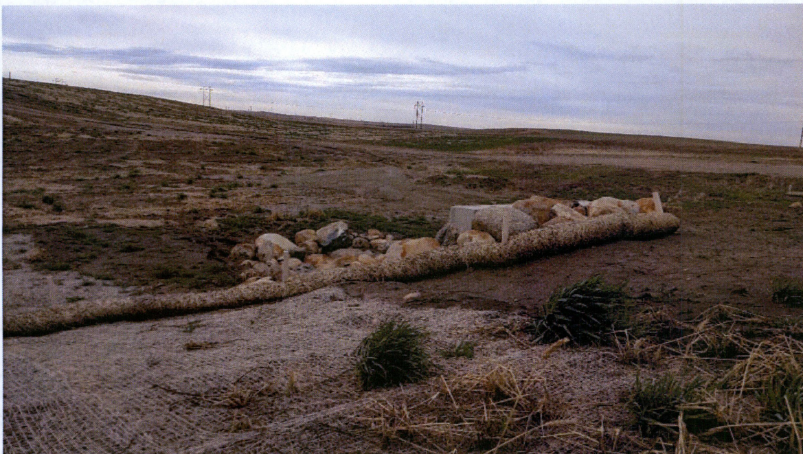
Photo 4. A wetland armored by riprap, a culvert, erosion mats, and waddles.
