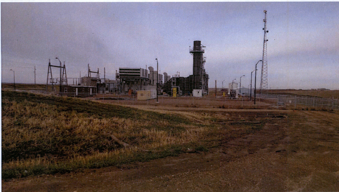
Photo 3. Lonesome Creek Station with partially-reclaimed sideslope and properly-installed waddles.
