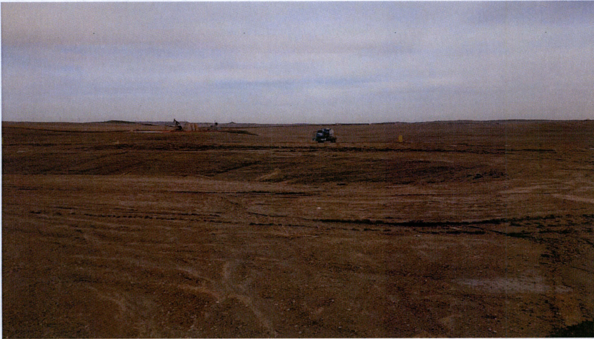
Photo 1. Unseeded/reclaimed portion of Project site with equipment sitting on level ground.
