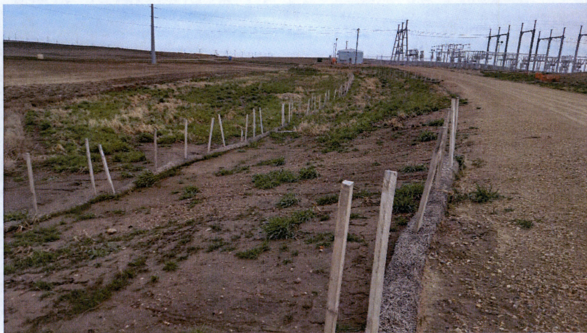
Photo 6. Waddles beginning to load up with sediment from recent rain event.
