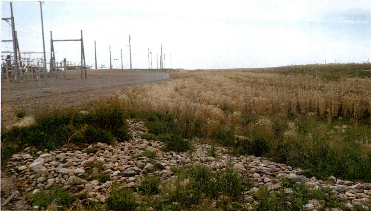
Photo 3. Lonesome Creek Station perimeter with partially-reclaimed side-slope and riprap.
