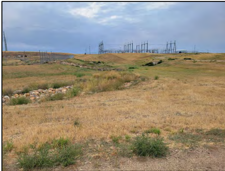
Photo 6. View looking south towards the Switchyard. Annual weeds should be sprayed along drainage ditches.
