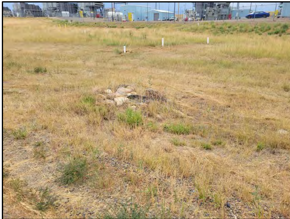
Photo 4. Culvert with rip-rap and revegetated.
