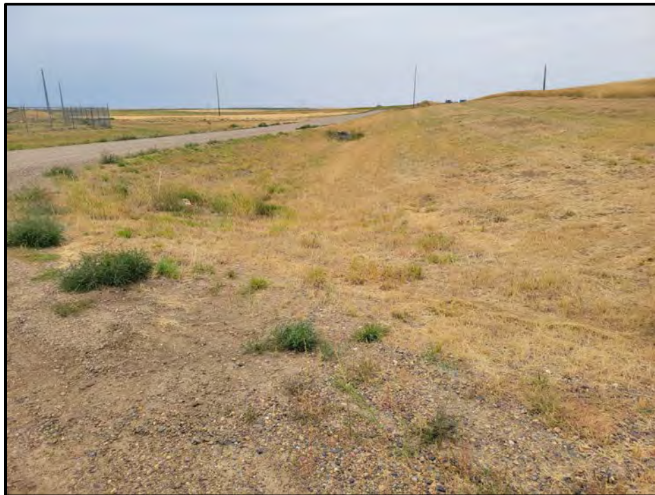
Photo 2. Drainage ditches are well-vegetated and free of erosion.
