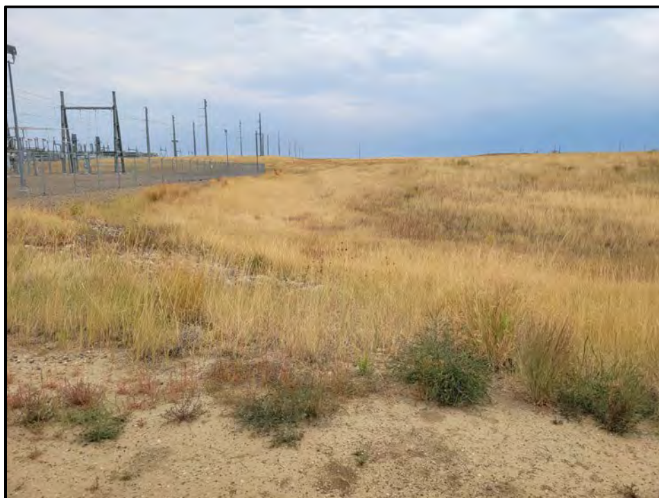
Photo 7. View looking east along the south side of the Switchyard. Grass planting is successful with no erosion observed.
