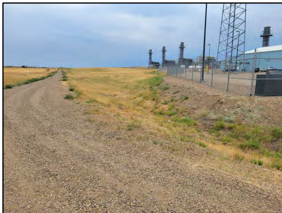
Photo 3. View looking east down the access road on the north side of the Phase III addition.
