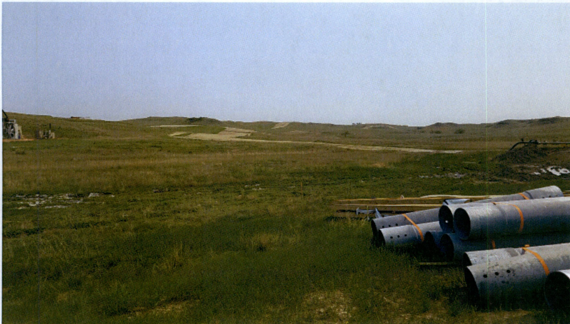
Photo 5. A wetland north of the electrical substation within Parcel 3. Recommend ECDs be placed along project areas edge to protect wetland.
