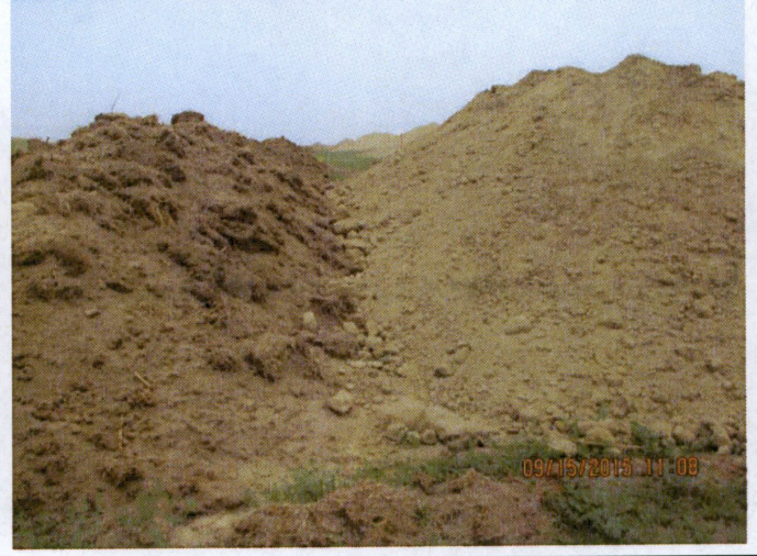
Photograph 2: Station # 986+00, spoil stored up onto stored top soil, top soil is also outside of staked project limits.
