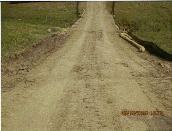
Photograph 7: Station # 29+40, wetland armored up with proper ECDs.
