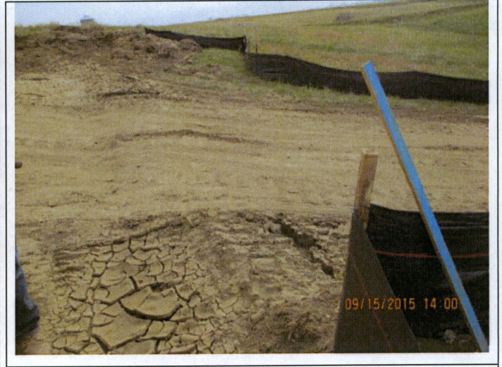
Photograph 8: Station # 29+40, pic 2 of water bars at wetland.
