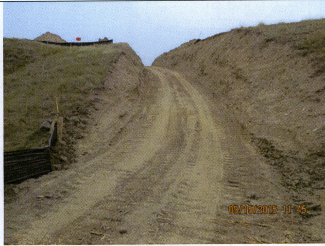
Photograph 5: Station # 643+50, wetland without ECDs in travel lane on slopes.
