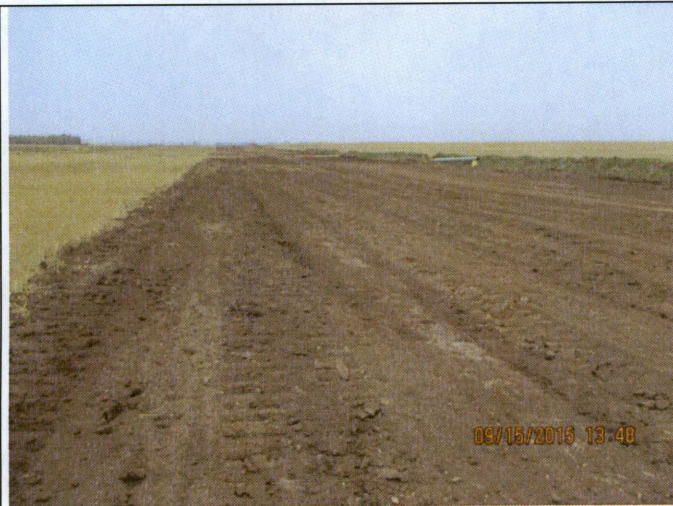
Photograph 11: Station # 7+50 viewing to the north of ROW after backfill.
