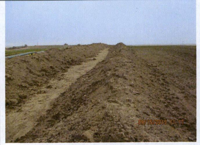
Photograph 4: Station # 966+00, spoil and top soil with proper separation.
