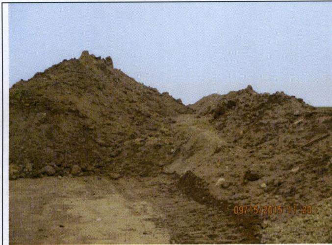
Photograph 3: Station # 968+00, spoil stored up onto stored top soil.
