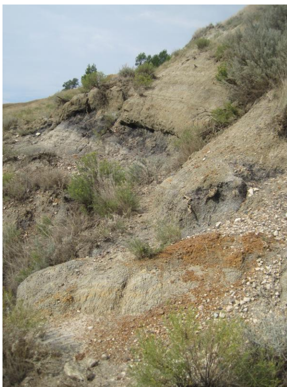
Figure 4. View of large slumped area of outcrop, Segment A-USFS-old (at point P5-120822-03). Photo Direction- Southwest
