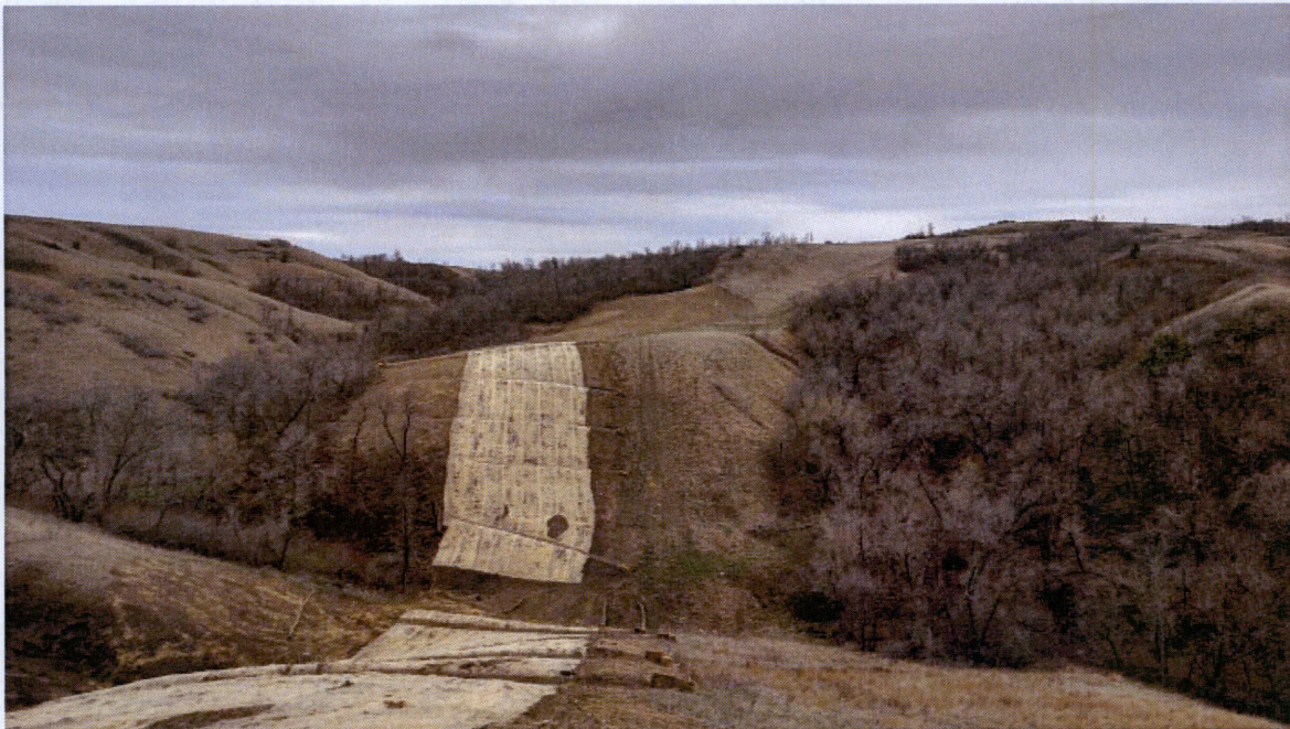
Photo 6. Clear-cut coulee crossing, showing ECDs including matting and waddles.
