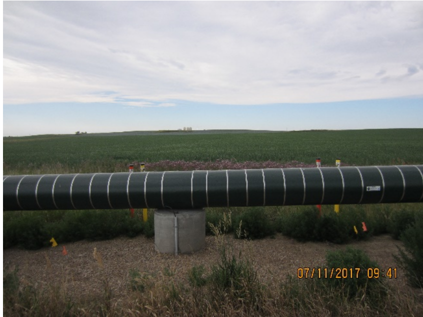
Photo 1: Looking south from Silurian Compressor Station, reclamation complete, no concerns.
