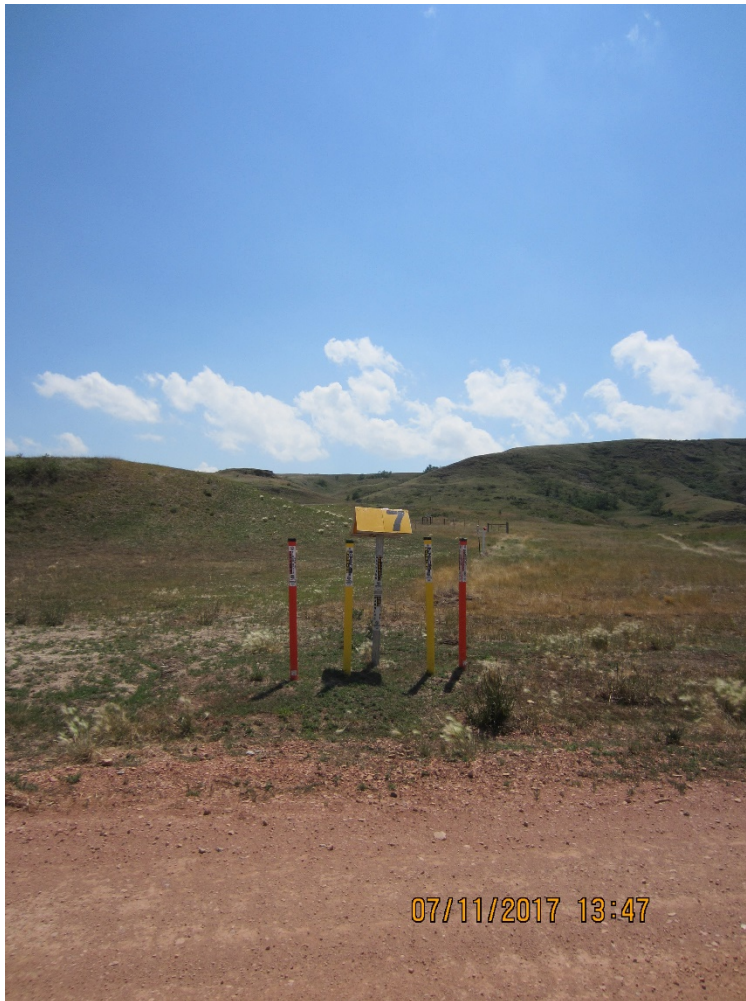
Photo 13: Federal land looking at pipeline marker 7, restoration complete, no concerns.
