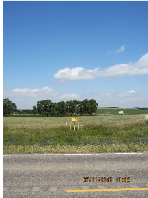
Photo 9: Looking north from Hwy. 1806 at pipeline marker 3, restoration complete.
