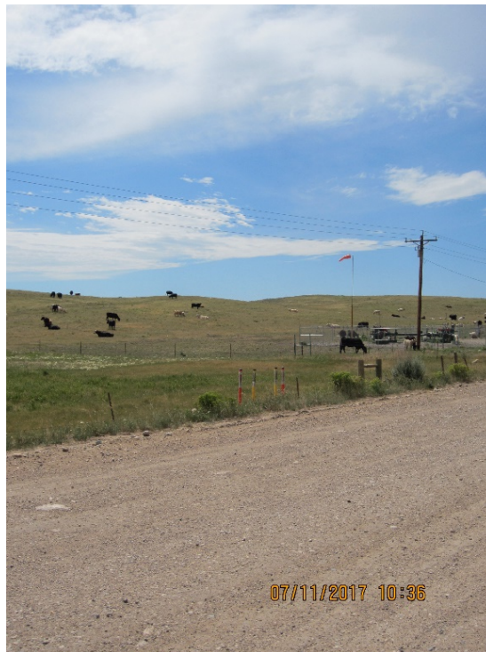
Photo 7: Looking south from the North Hofflund Valve Station, restoration complete.
