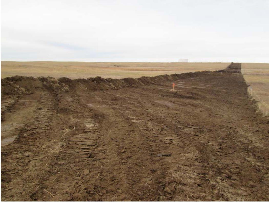
Above: Photo 5 (pt. 202) – Direction looking north towards Skunk Hill. Topsoil stripped.
