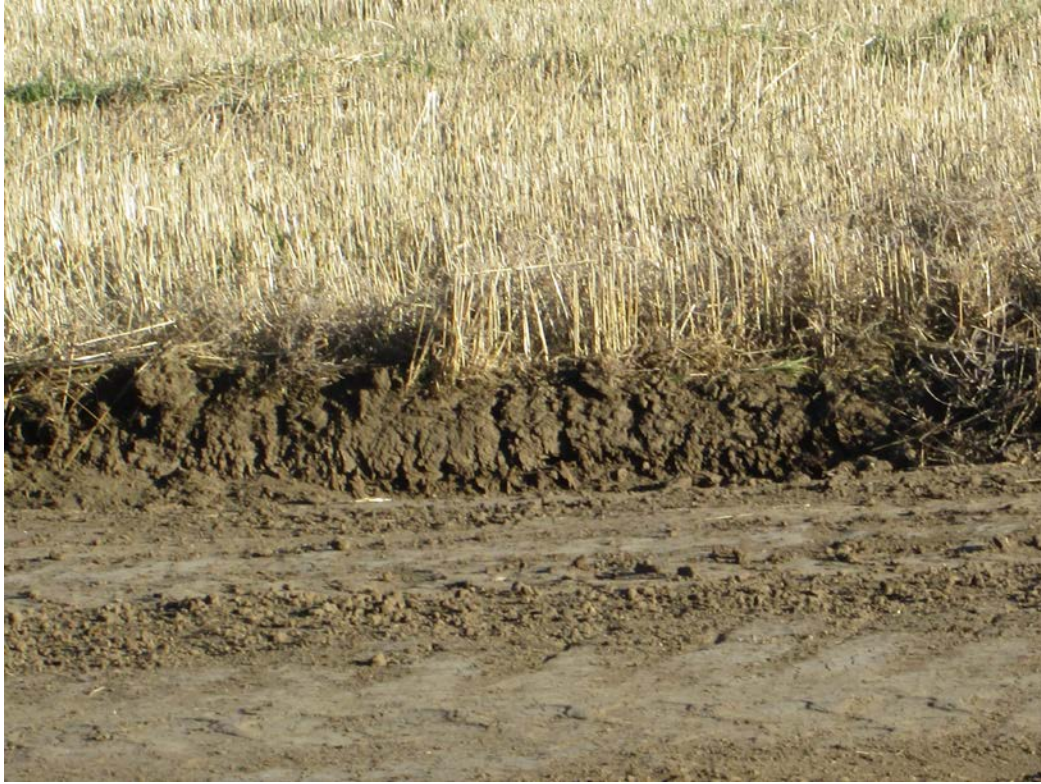
Above: Photo 17 (pt. 212) – ROW topsoil has been removed, area in crop land.
