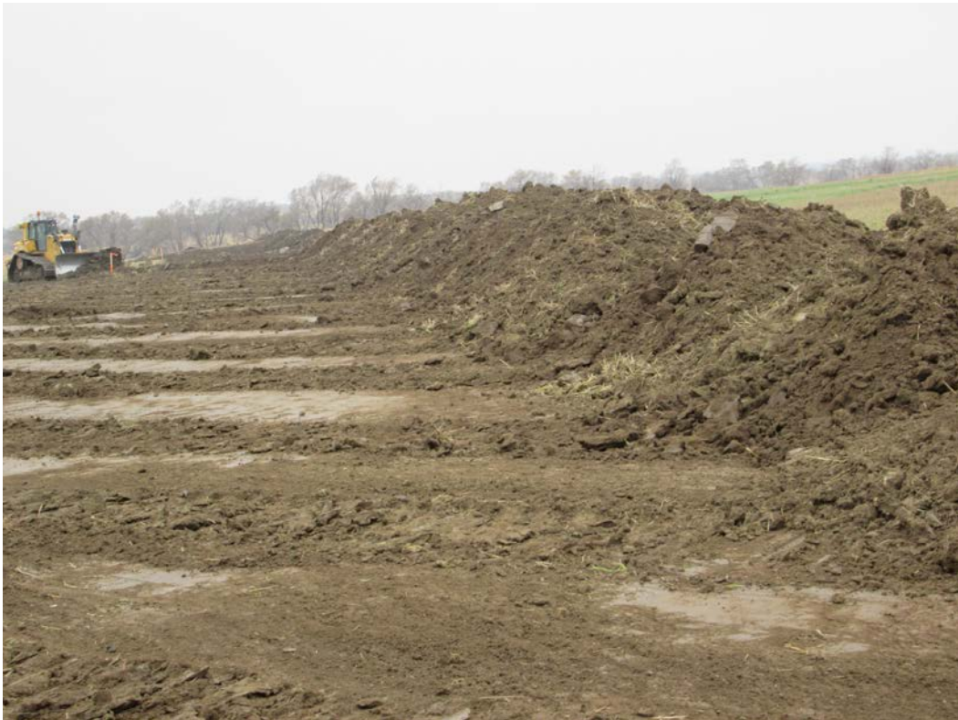
Below: Photo 8 (pt. 206) – Dozer stripping topsoil. Looking S-SW.
