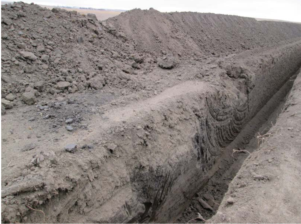
Above: Photo 19 (pt. 213) – Trench. Subsoil pile to the left.
