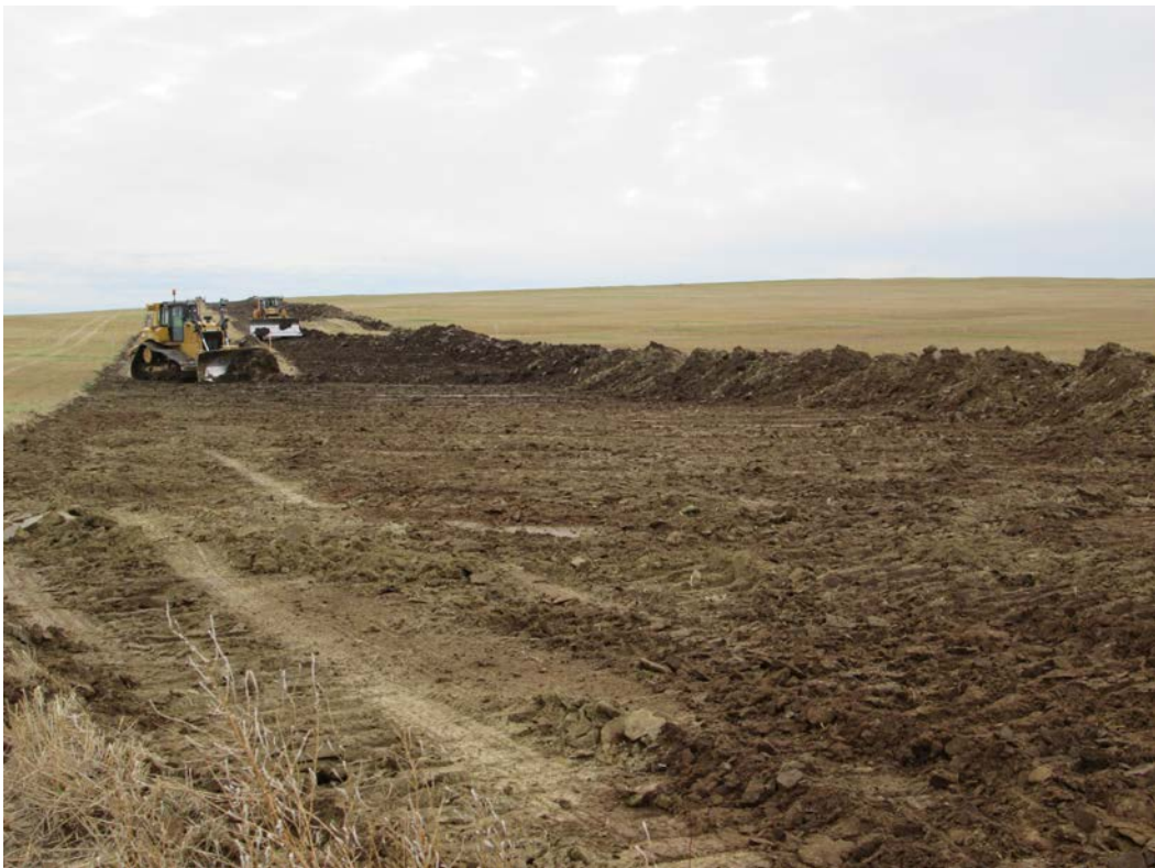
Below: Photo 6 (pt. 202) – Direction looking south. Topsoil being stripped.
