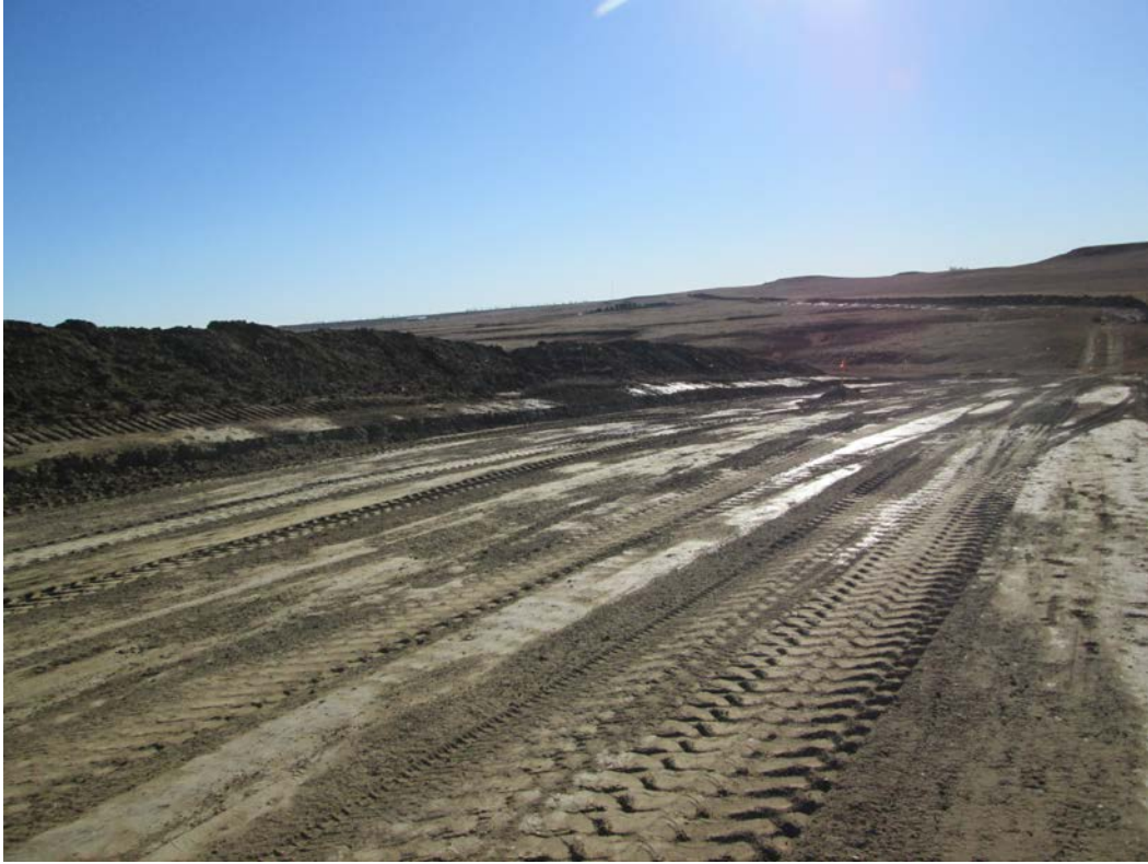
Above: Photo 11 (pt. 208) – Side-sloping/two-toning area, used to level hill slope. Moved topsoil to opposite side. Looking southwest.
