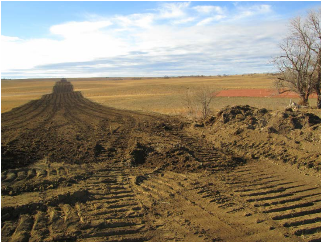
Above: Photo 25 (pt. 216) – Topsoil replaced. Lighter colored subsoil at very bottom of photo where topsoil has not been replaced yet. Looking southwest.
