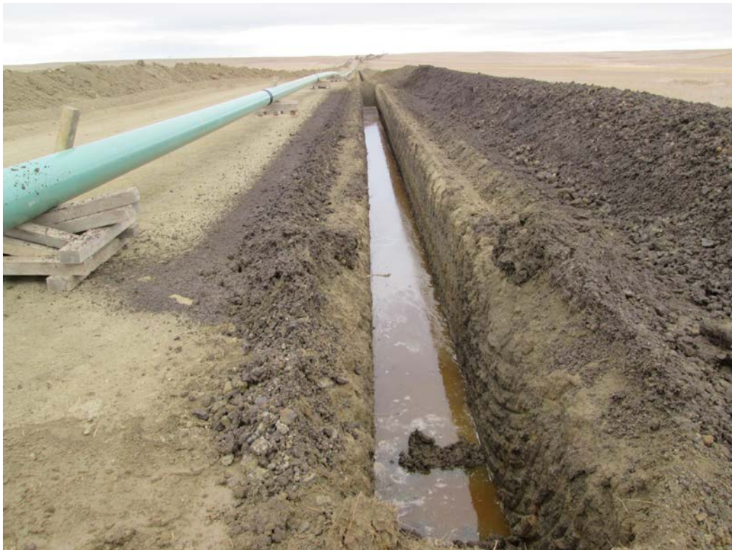
Below: Photo 20 (pt. 214) – Trenching machine removed subsoil. Subsoil pile to the right. Wet area, sediment plug towards the top of photo to help stop water. Looking northeast.
