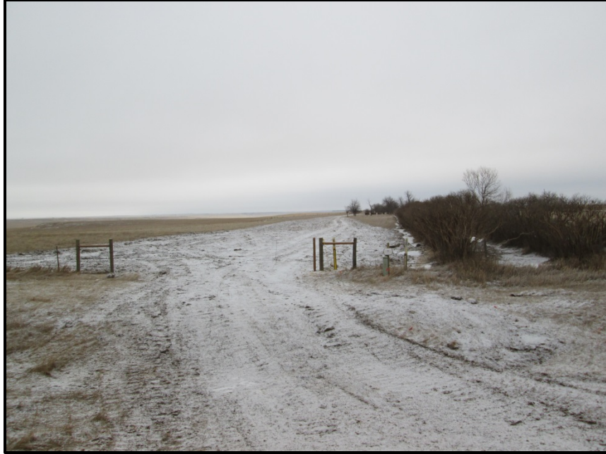
Photo 11. Direction: East (GPS Point #230). Road bore work area of 134 th Ave. Pipeline continuities along tree rows, bottlenecks (smaller ROW area) as to not disturb two trees visible in distance. No trees were removed.
