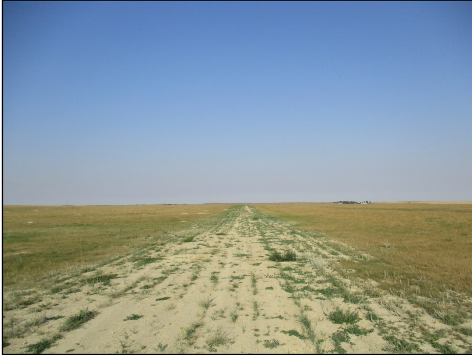
Photo 3. (GPS Point #461) – Notice the very narrow ROW, far less than the typical 100 or 75ft ROW. This area was double ditched, not top-soiled, as requested by the U.S. Forest Service. There are a few prairie dog holes along this area. Direction: West.
