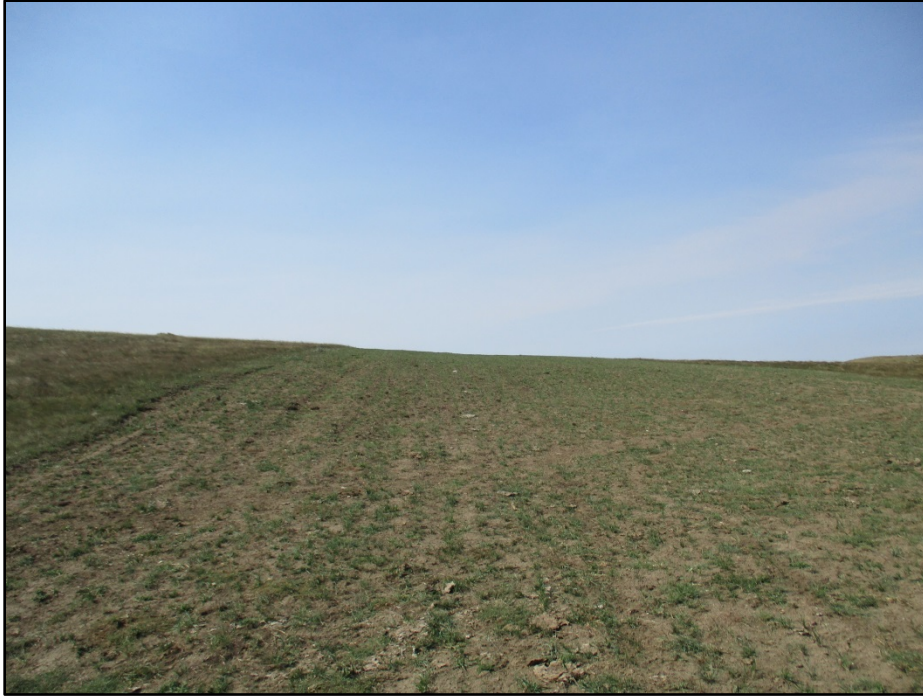
Photo 13. (GPS Point #472) – Pipeline ROW in pasture/rangeland; this area has been grazed. Some grasses were growing. Contours appeared to match up well on sloping hills. Direction: Northeast.
