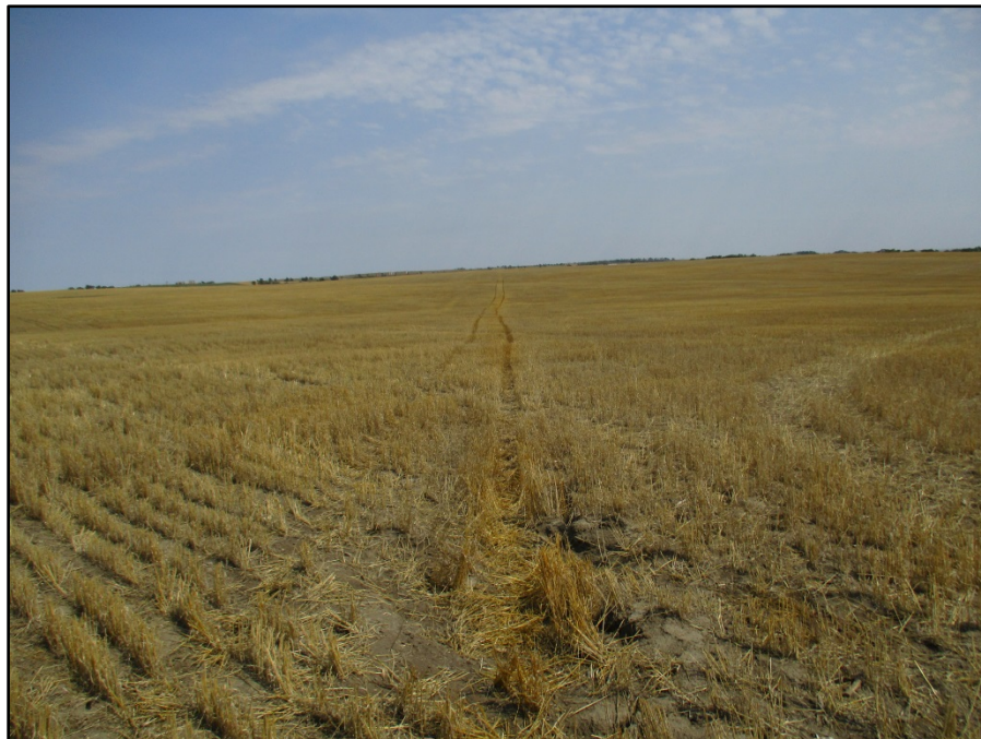
Photo 20. (GPS Point #478) – Pipeline ROW through a wheat field that had some soil subsidence. Inspector stated this will be fixed when all crops have been harvested from project area. Direction: Northeast.
