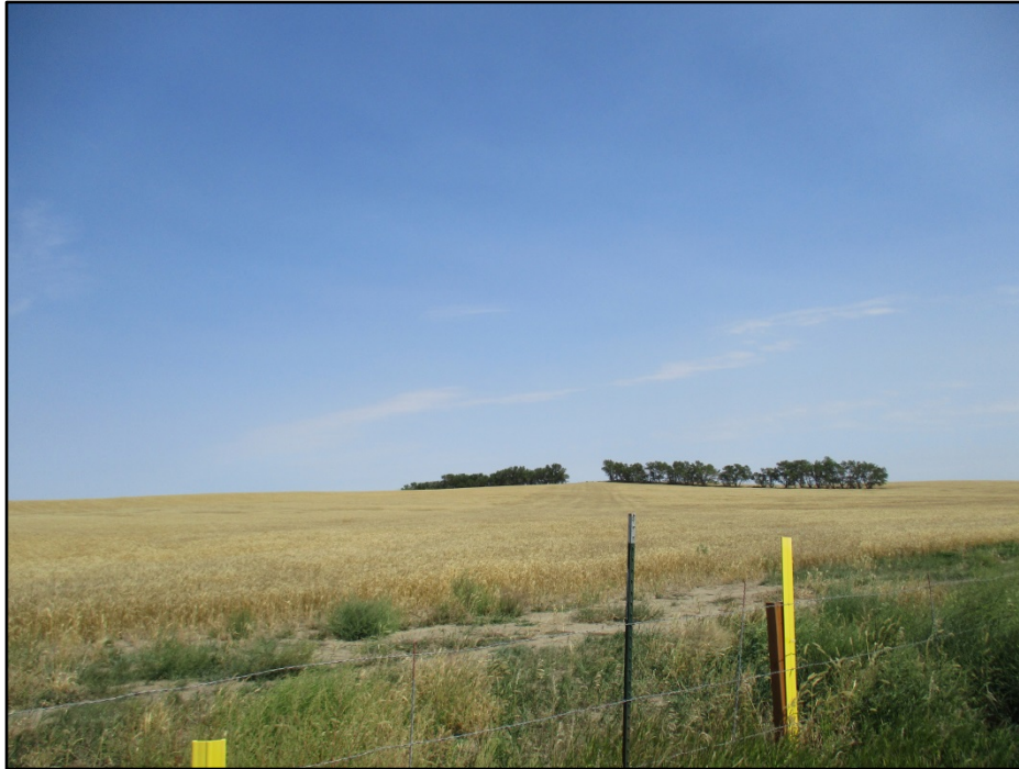
Photo 21. (GPS Point #479) – Pipeline ROW through wheat field. The crop within the ROW appeared to be growing similarly in size and density to the adjacent part of the field, indicating proper soil replacement and restored function. Direction: Northeast.
