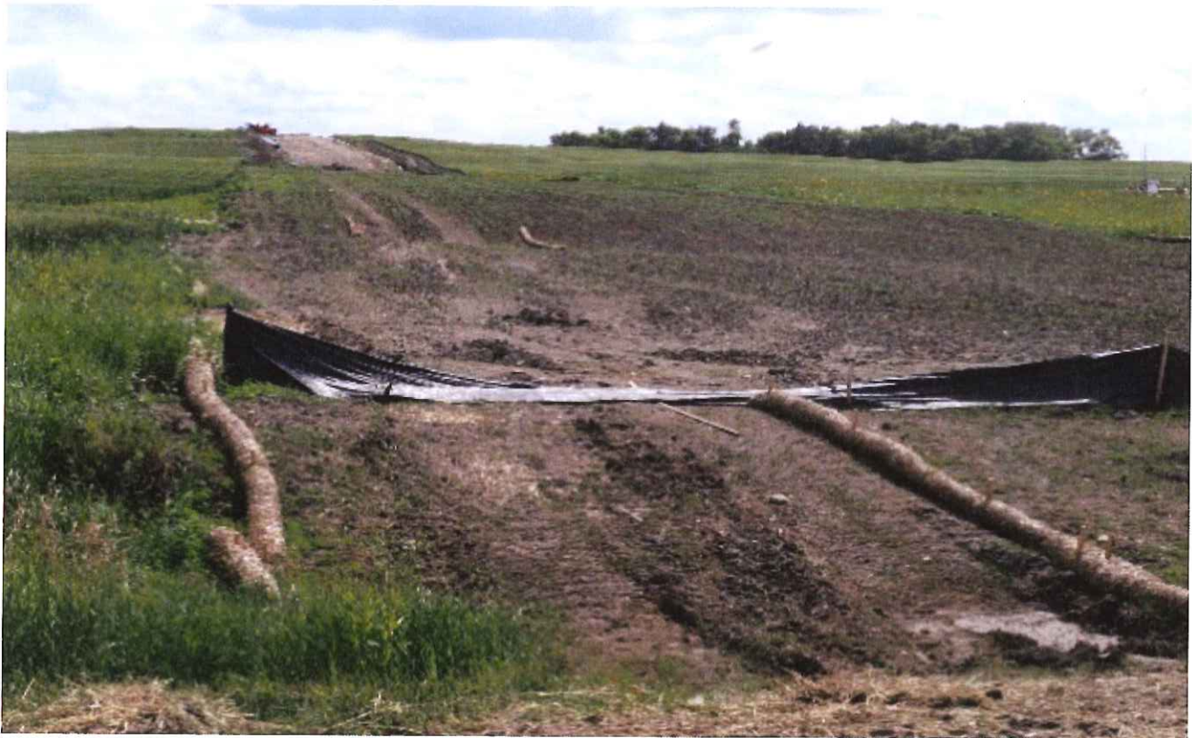
The next two photos, taken at a location east of 87 th Avenue on an unnamed road in Mountrail County, show an area where silt fence was installed but then evidently run over and neglected.
