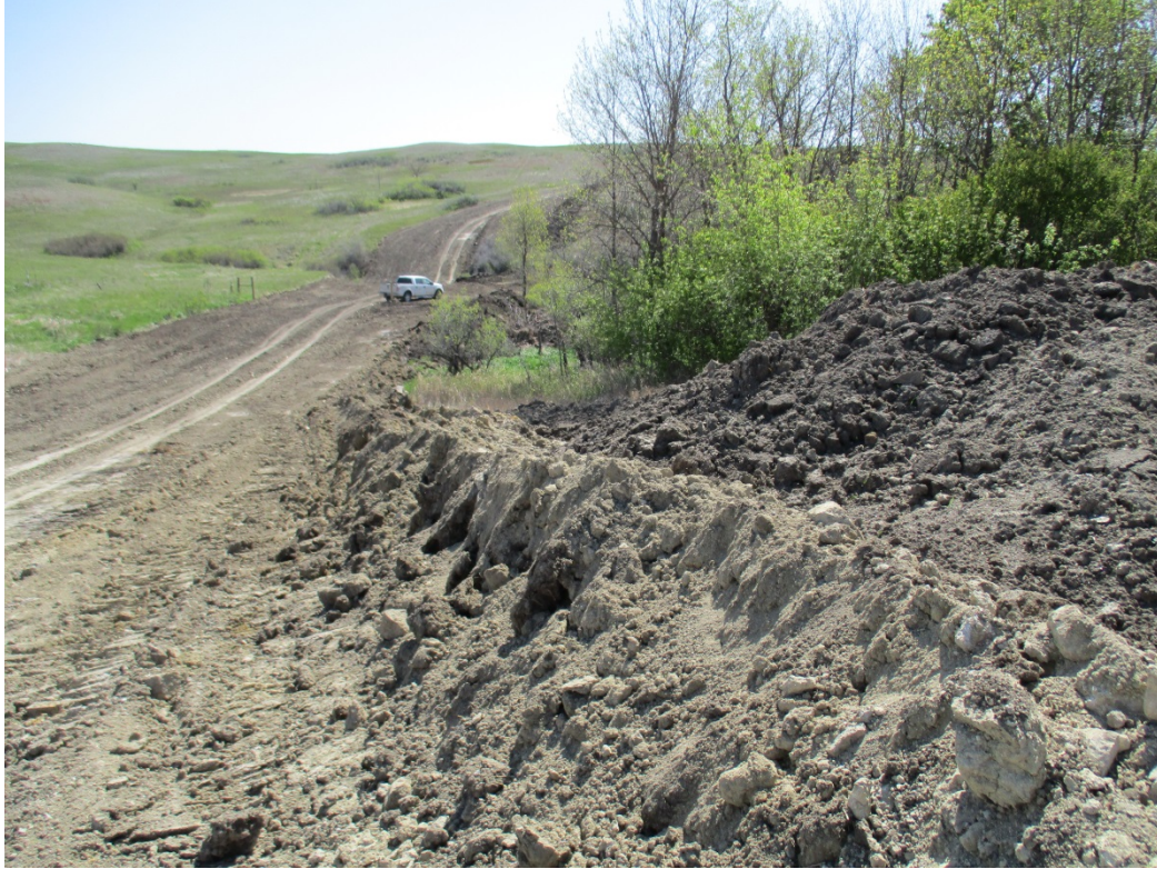
Above: Photo 21 (pt. 290) – Topsoil pile with a small amount of subsoil pushed on top of topsoil pile. Direction looking east.
