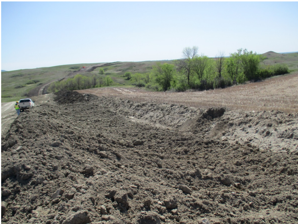
Below: Photo 20 (pt. 289) – Two-tone area. Topsoil pile to the far right, subsoil to the left of photo. Both piles appear to be the same color. Direction looking east.
