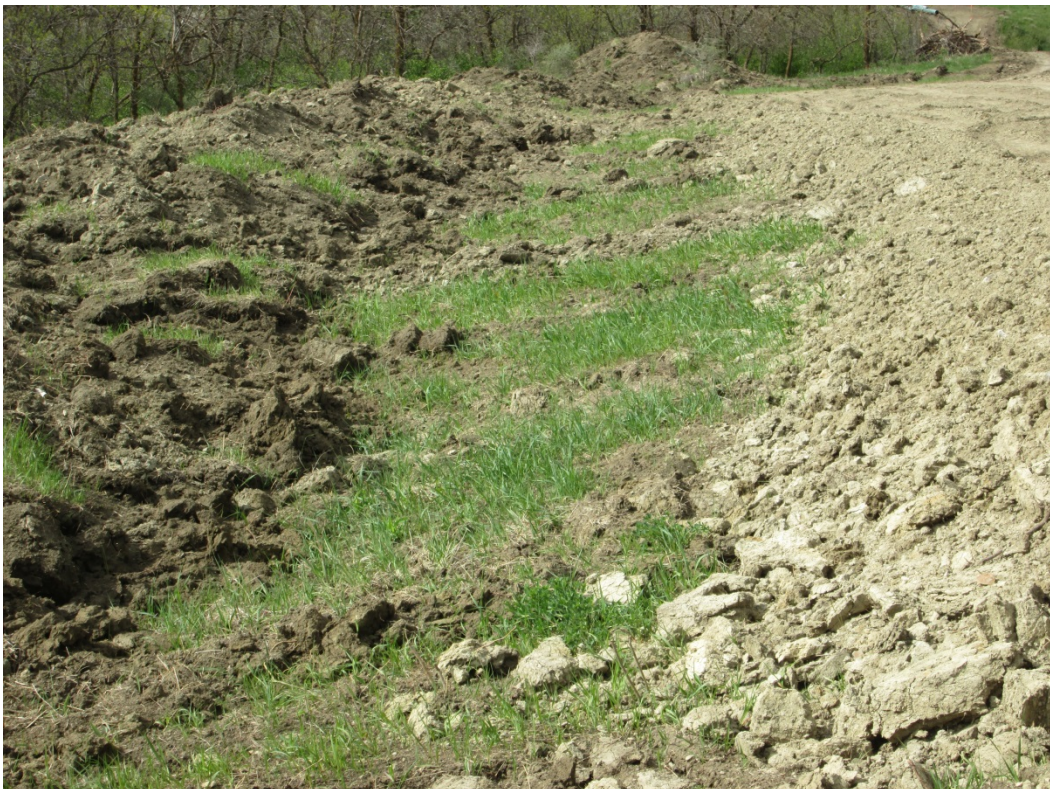
Above: Photo 11 (pt. 280) – Open trench, with pipe strung along side and subsoil pile flattened on the other side of the pipe to create a work space. Topsoil on far ROW edge. Below: Photo 12 (near pt. 281) – Topsoil pile to the far left and subsoil to the right of photo. Grass growing in-between piles. This area may not have been properly stripped of topsoil, potentially may have subsoil on top of topsoil and vegetation.
