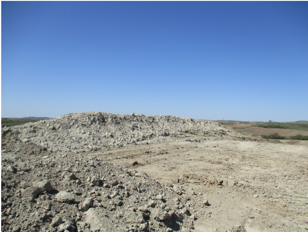
Above: Photo 19 (pt. 289) – Topsoil pile on hilltop area. Pile is very light in color and appears to have a lot of subsoil in pile.
