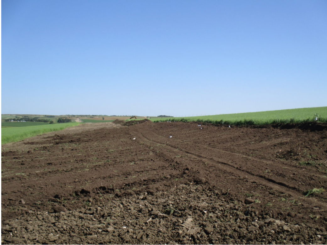
Above: Photo 31 (pt. 445) – Unfinished, started topsoil replacement.
