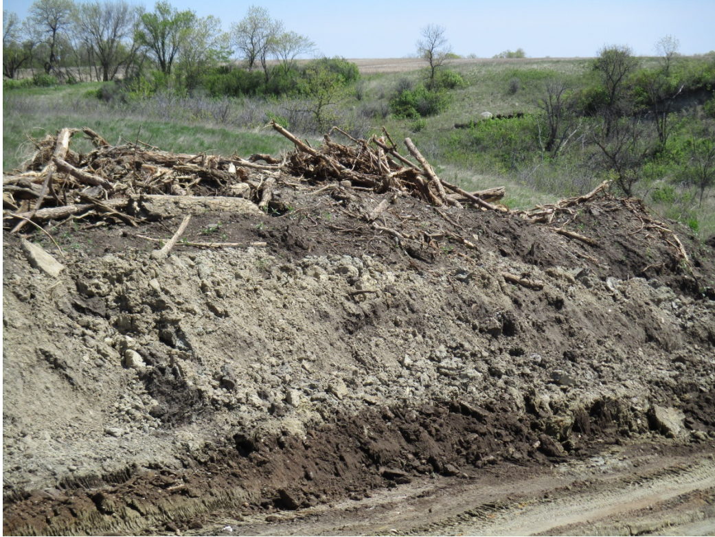
Above: Photo 25 (pt. 295) – Topsoil pile with some subsoil on it, along with woody debris. Unknown what will be done with the woody debris.
