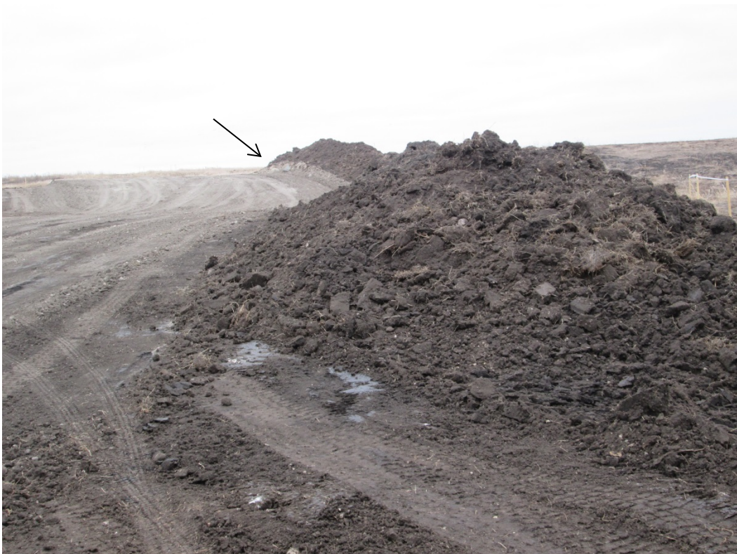
Below: Photo 8 (pt. 234) – Bore location (leveled and smoothed). Notice small amount of subsoil on top of the bottom of the topsoil pile (shown by arrow). Direction looking west.
