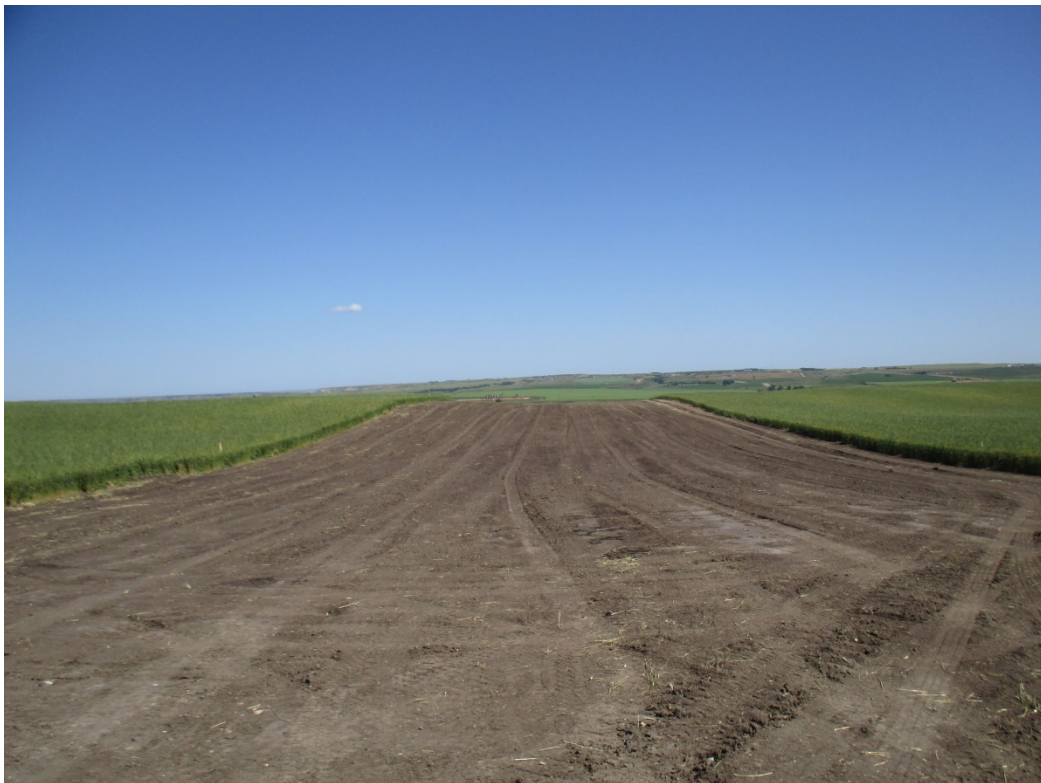
Below: Photo 34 (pt. 446) – Topsoil replaced on ROW area. Contours appear to match up. Direction looking west.
