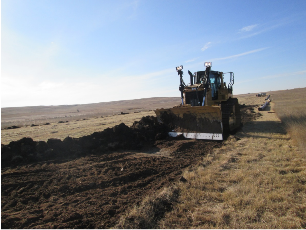
Above: Photo 3 (pt. 232) - Start of topsoil stripping. Direction looking south.
