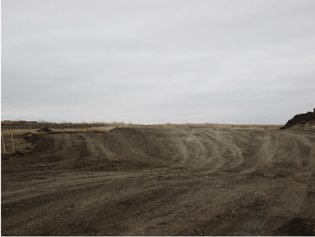
Above: Photo 7 (pt. 234) – Bore location (leveled and smoothed). Notice small amount of subsoil on top of the bottom of the topsoil pile to right of photo. Direction looking west.
