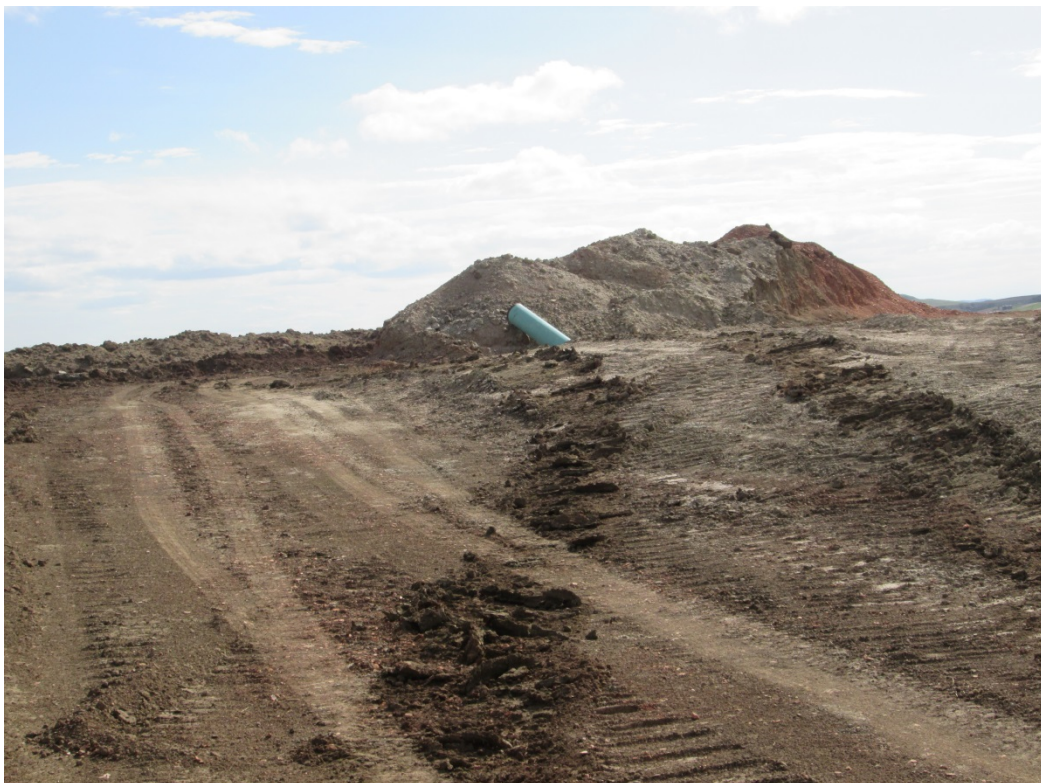
Below: Photo 16 (pt. 285) – Subsoil pile in middle of ROW. Clinker, also called “scoria,” is mixed in the pile which was from an old wellpad site.
