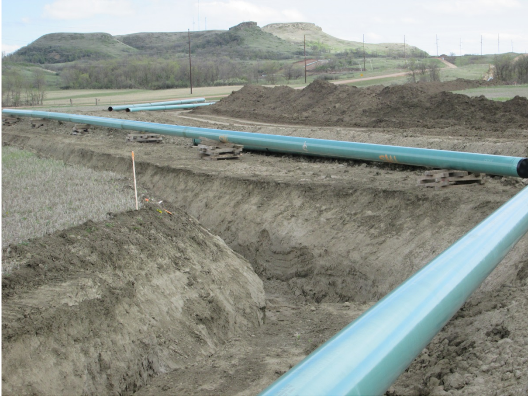
Above: Photo 11 (pt. 280) – Open trench, with pipe strung along side and subsoil pile flattened on the other side of the pipe to create a work space. Topsoil on far ROW edge. Below: Photo 12 (near pt. 281) – Topsoil pile to the far left and subsoil to the right of photo. Grass growing in-between piles. This area may not have been properly stripped of topsoil, potentially may have subsoil on top of topsoil and vegetation.
