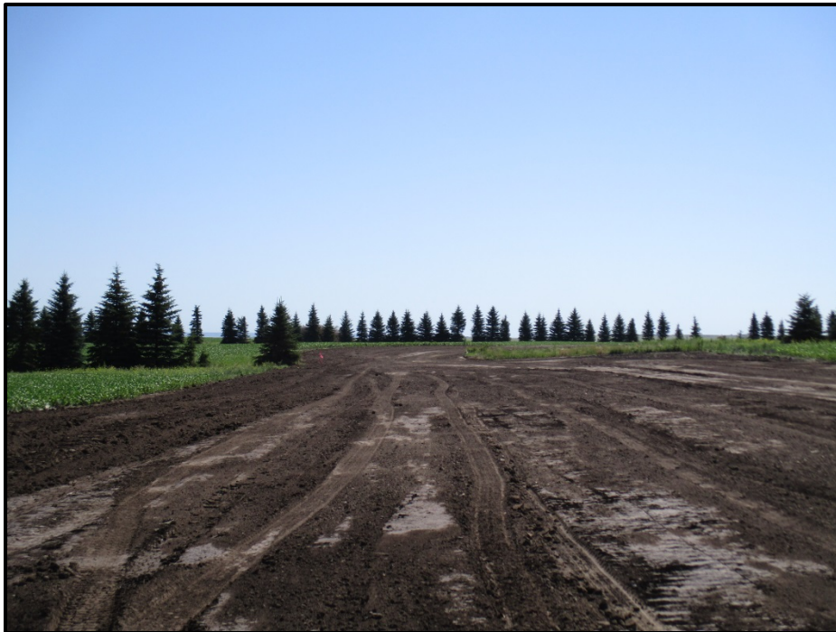
Photo 6. (GPS Point #448) – ROW necked down to 50 ft width through tree rows. Unknown if or how many trees were taken out in this area. Topsoil replaced back on the ROW. Direction: East.
