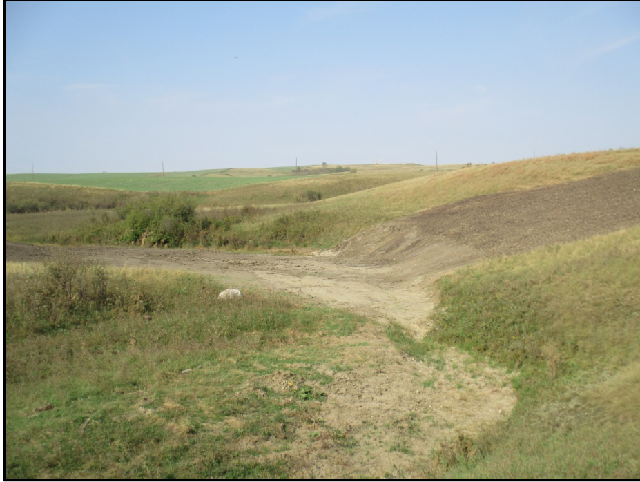
Photo 17. (GPS Point #482) - Drainage area, no erosion control device. Area along the drainage pathway looks light in color, possibly due to topsoil erosion. Direction: West
