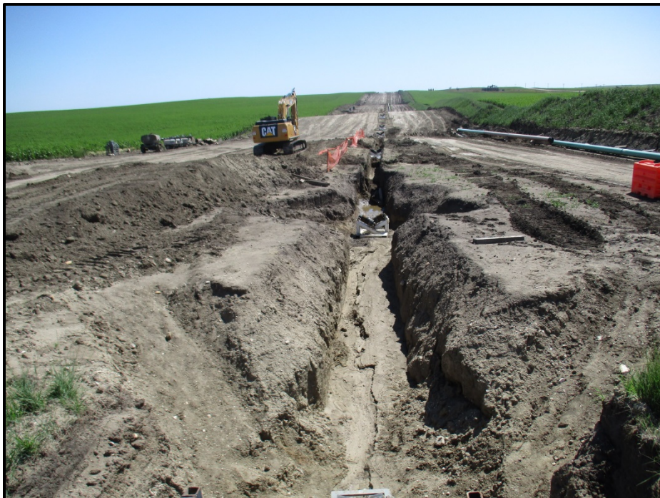
Photo 12. (GPS Point #450) - Open trench with few orange blockades ending to the right of photo, and only partial orange fence to the left of trench. White and black pipe rollers in trench were used to guide bore pipe. Photo taken from bridge shown in photo #11. Direction: East
