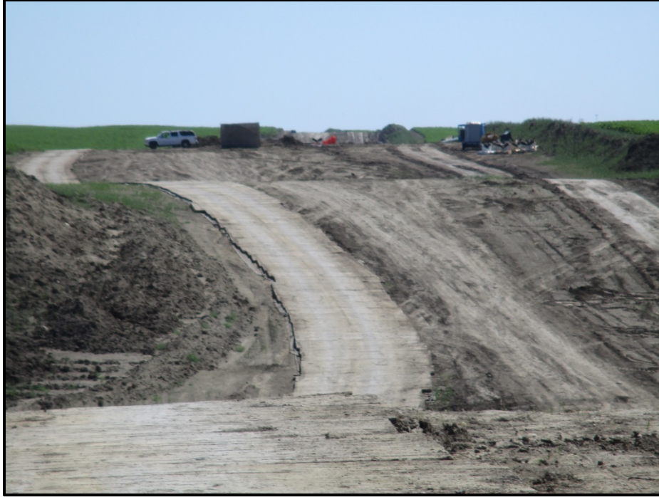
Photo 9. (GPS Point #449) – ROW going up to Lake Sakakawea bore area. The bore contractor wanted mats placed on ROW up to bore area. Mats are observed on the left side of the ROW. Direction: East
