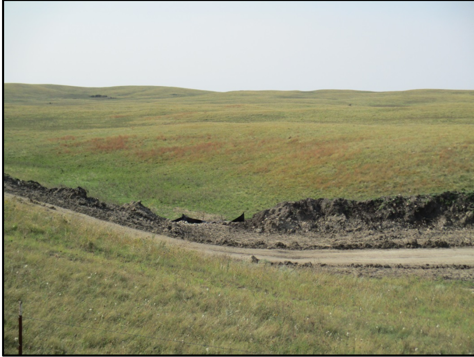
Photo 21. (GPS Point #484) - Silt fence in drainage area, needs maintenance. Direction: South
