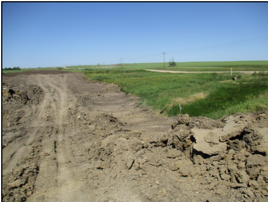
Photo 4. (GPS Point #446) - Drainage area intersected by ROW. Pipe trenched and backfilled along the edge of the ROW. The drainage area appeared to be a potential wetland. Notice the vegetation change. However, the environmental inspector stated it was not a wetland. No erosion control devices were observed. The PSC was informed of this site the day after the inspection.
