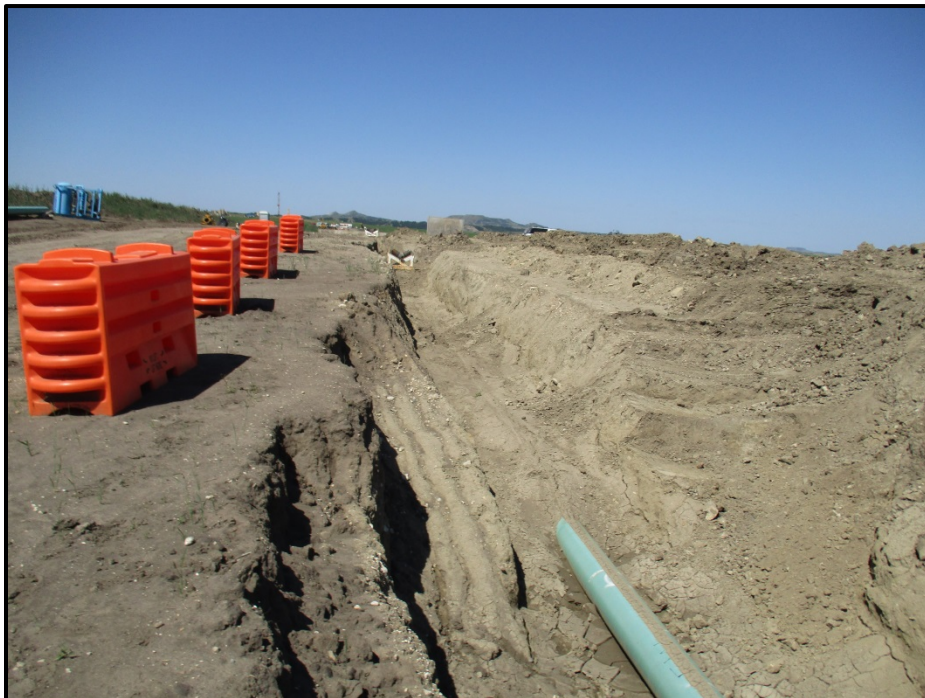
Photo 10. (GPS Point #450) - Open trench with partially covered pipe in trench. Orange safety blockades to the left of photo. White and black pipe rollers (visible in trench in far distance of photo) were used to guide the bore pipe into bore hole. Direction: West
