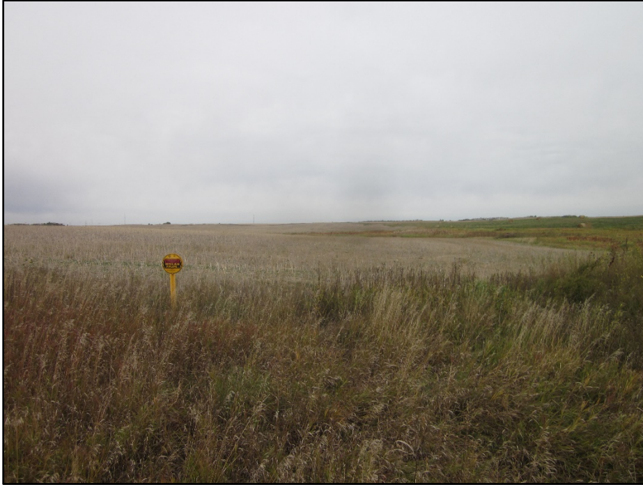
Photo 9. (GPS Point #613) Direction: North. Pipeline ROW through cropland. This segment of the pipeline was bored underneath the gravel road to the south (60 th St NW) and the wetland in the distant right of the photo. The wetland appeared to have naturally-growing vegetation on the margins with no indications of previous disturbance.
