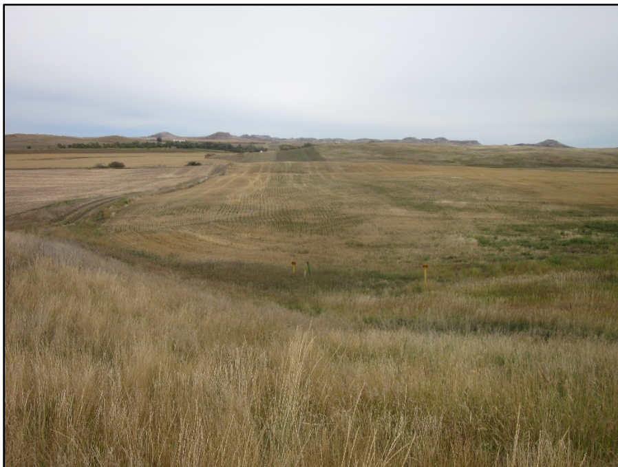
Photo 30. (GPS Point #630) Direction: West. Pipeline ROW through field west of ND Highway 23. Sacagawea line is on north side; a gas line parallels it and was completed in January 2017 and seeded in spring 2017.
