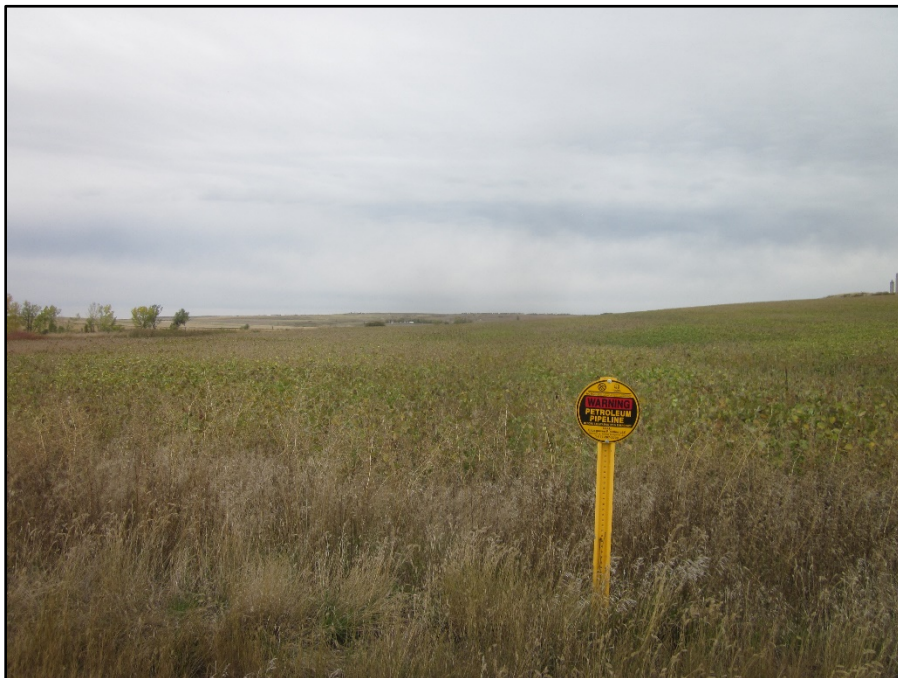
Photo 26. (GPS Point #627) Direction: North. Pipeline ROW through field of soybeans on north side of 32 nd St NW. No visible difference within or outside of ROW.
