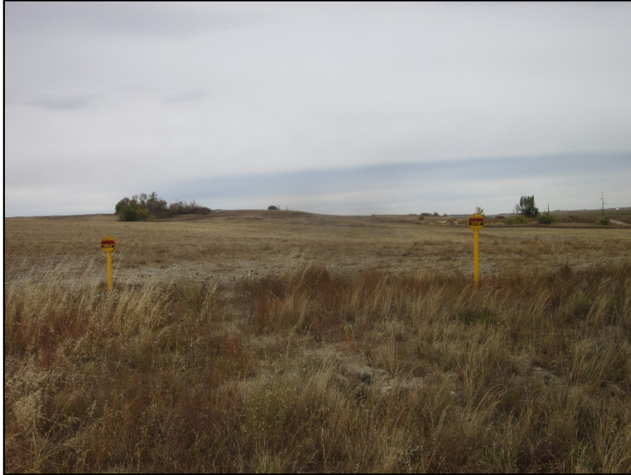
Photo 31. (GPS Point #631) Direction: North. Pipeline ROW through field north of 32 nd St NW. Field had been tilled after harvest.
