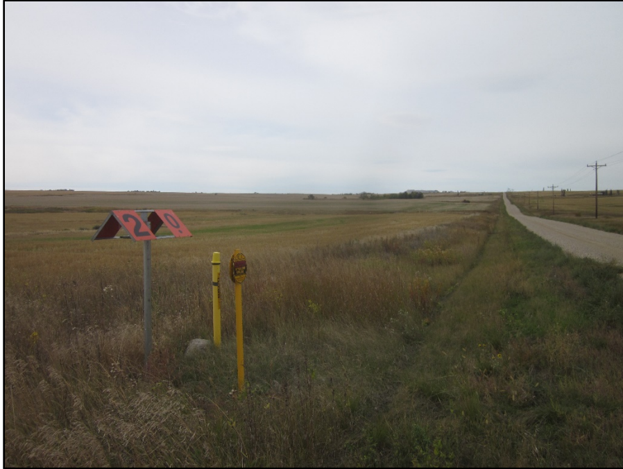
Photo 27. (GPS Point #627) Direction: West. Pipeline ROW parallels south side of 32 nd St NW. Cropland stubble looked comparable in density within and outside ROW. Drainage crossing in distance (not clearly visible in photo) was repaired adequately and revegetated.
