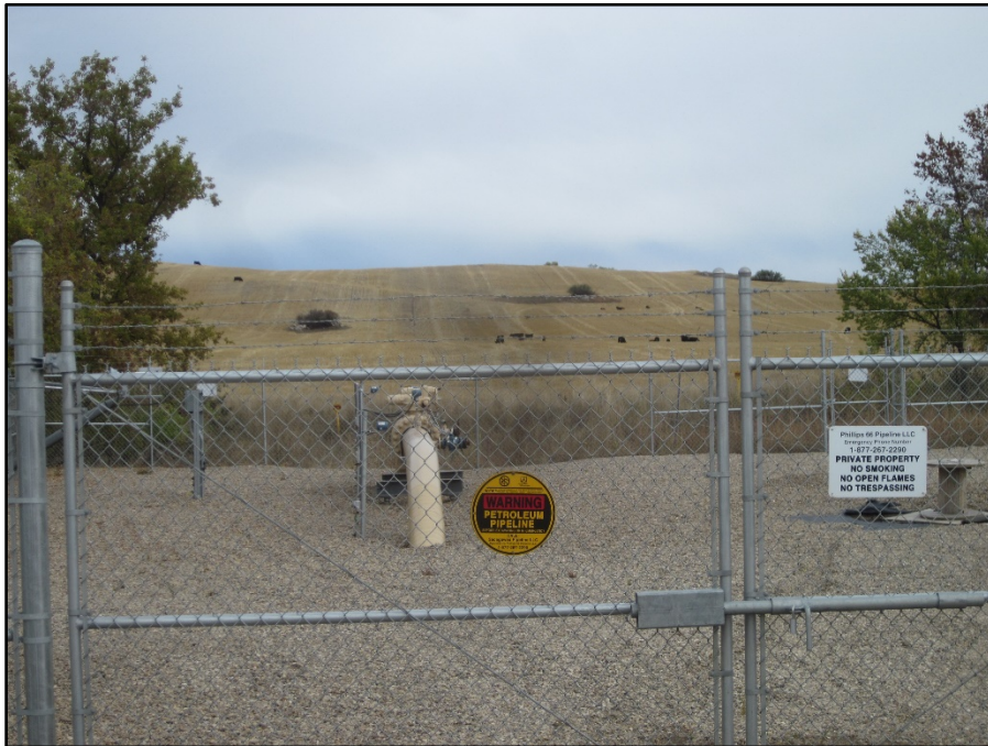
Photo 36. (GPS Point #635) Direction: East. Valve for Sacagawea line. Pipeline ROW continues east through field. Contouring was good. Crop stubble was thinner in ROW.
