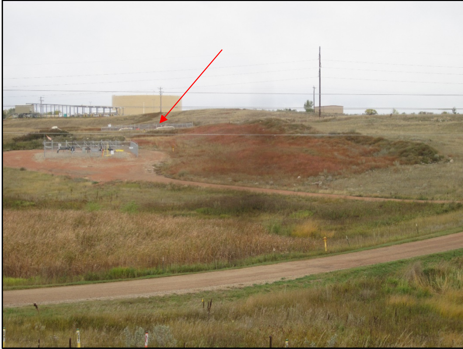
Photo 1. (GPS Point #607) Direction: North. The valve setting in the upper left of the photo (red arrow) is the connection of the Sacagawea pipeline to the Palermo Rail Terminal Facility on the north end of the route. Pipeline marker for the line is visible in the lower right. Wetland in foreground was bored underneath as part of the bore under U.S. Highway 2.
