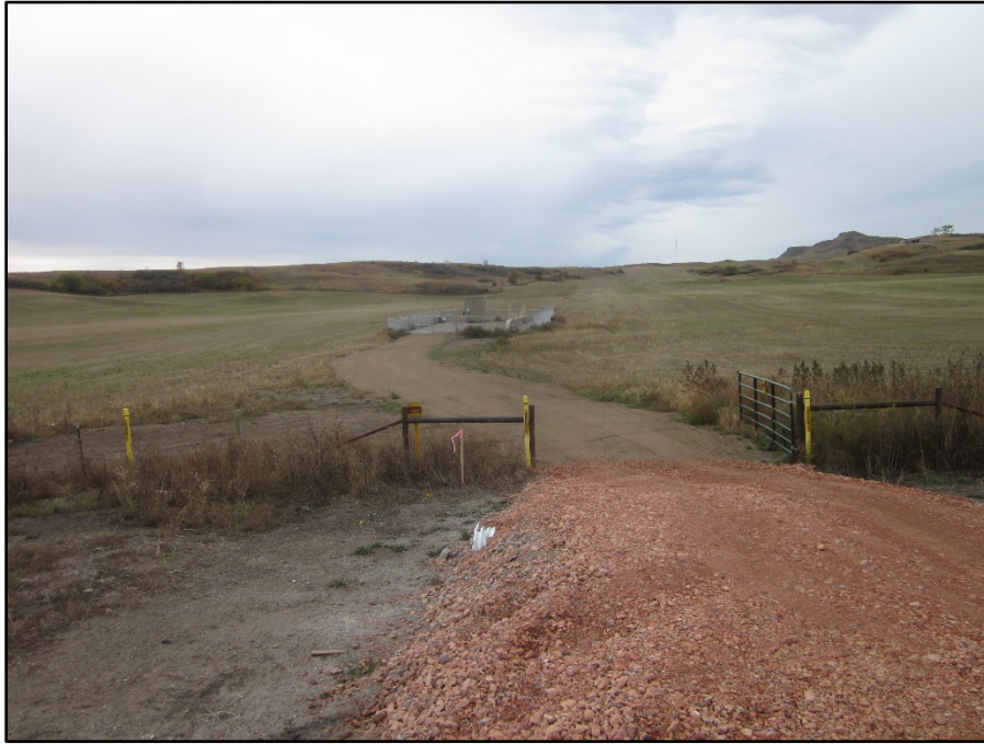
Photo 35. (GPS Point #635) Direction: West. Pipeline ROW through field on the north of the valve setting in the distance. The valve is for the adjacent gas line. Saddle Butte visible in the distance.
