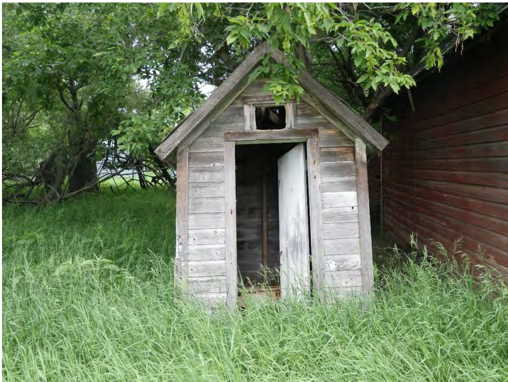
Figure 37: Overview of Feature 3, privy, view to the north.
