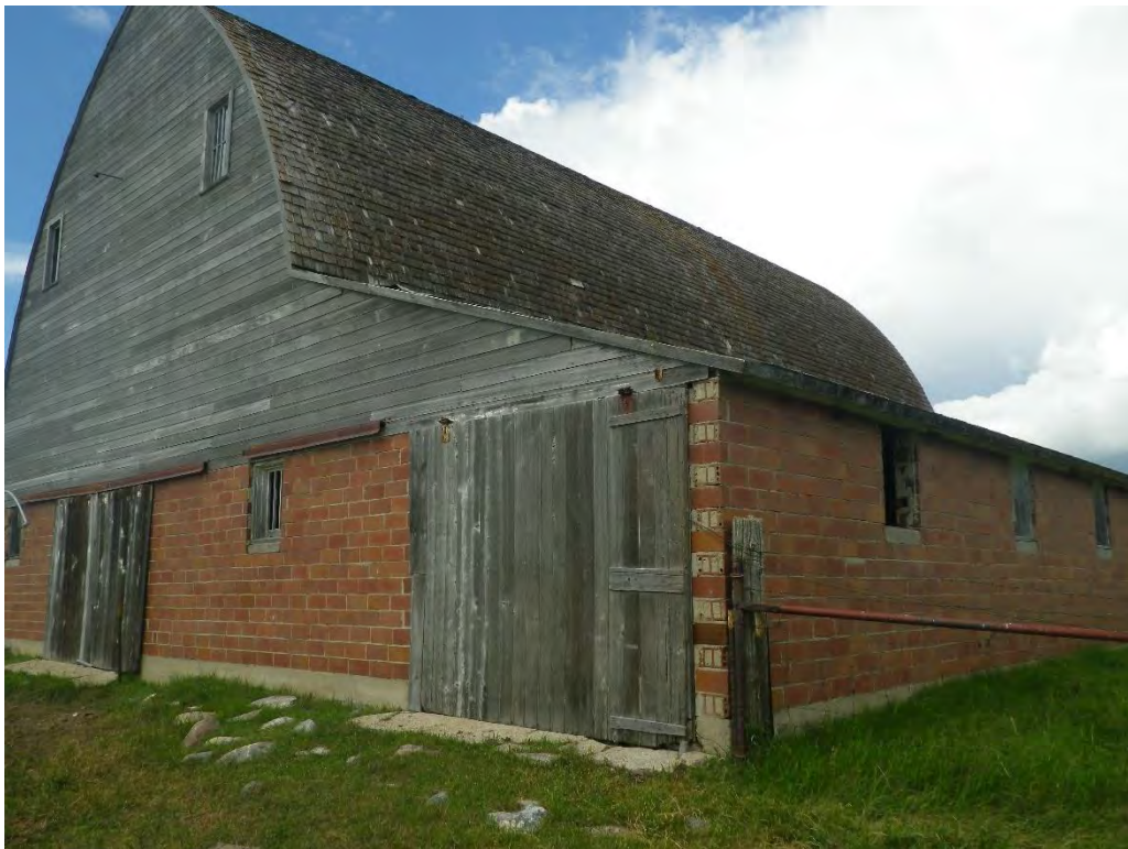
Figure 26: Southeast corner of Feature 2, barn, view to the northwest.
