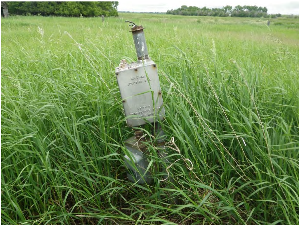
Figure 43: Overview of Feature 9, power box, view to the north.
