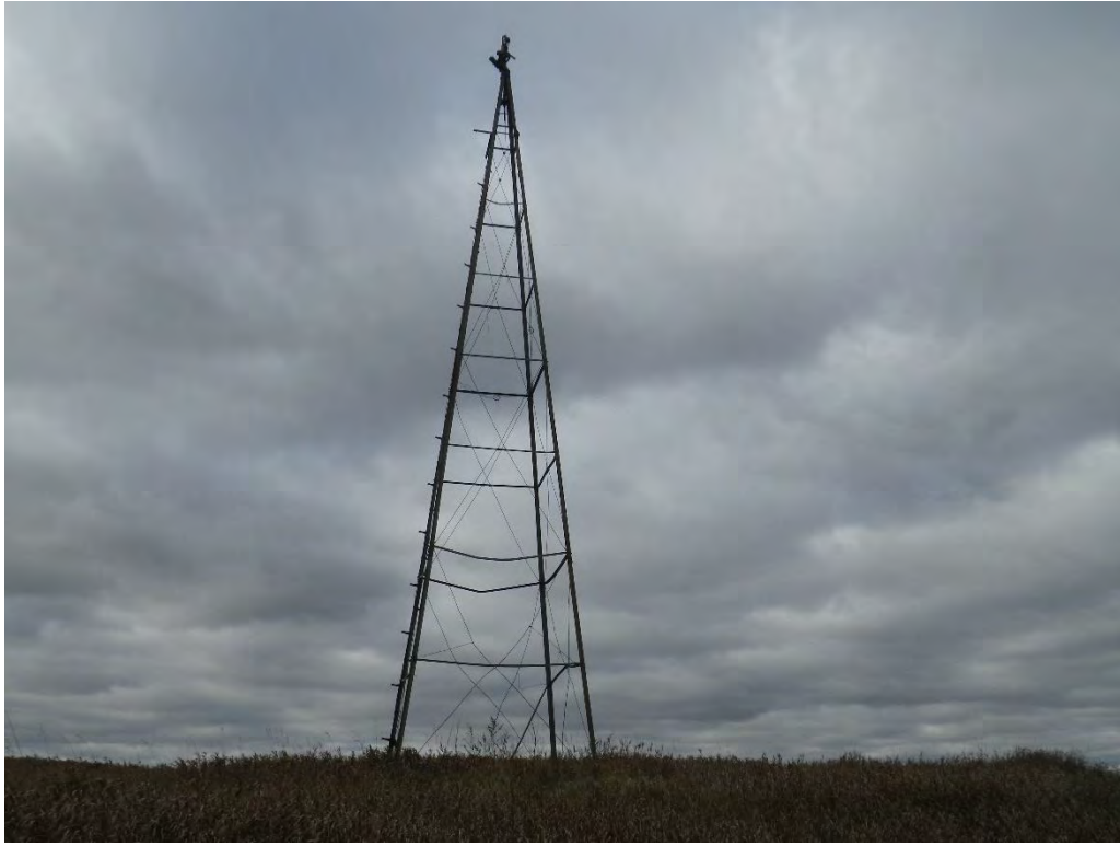
Figure 50: Overview of Feature 1, windpump, view to the west.
