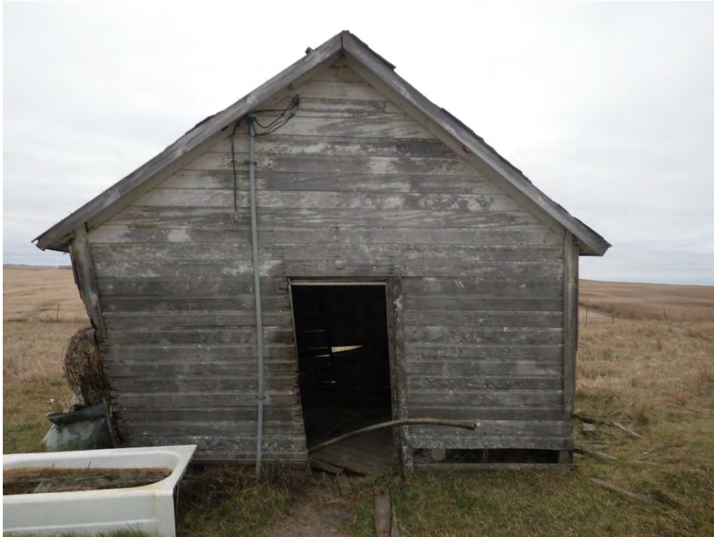
Figure 23: Overview of Feature 1, outbuilding, view to the south.
