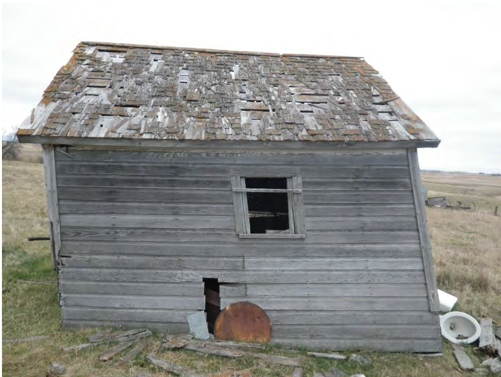
Figure 24: Overview of Feature 1, outbuilding, view to the east.
