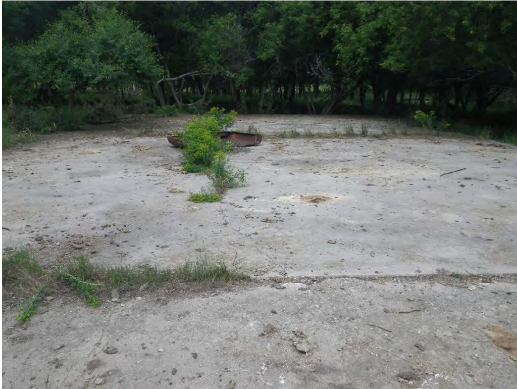
Figure 29: Overview of Feature 5, poured concrete foundation, view to the north.
