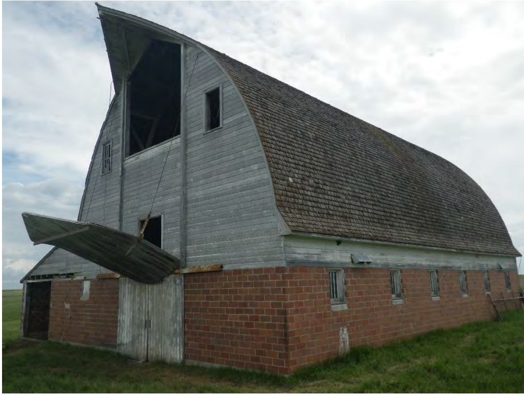
Figure 25: Northwest corner of Feature 2, barn, view to the southeast.
