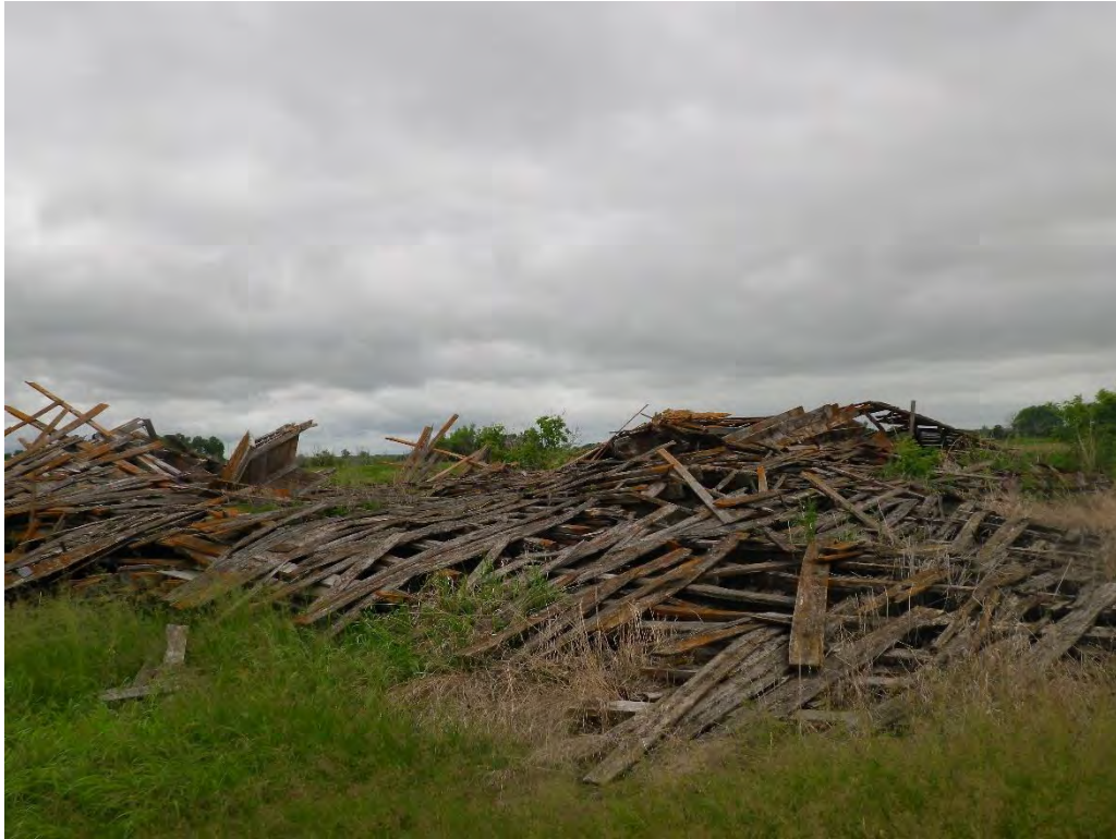
Figure 42: Overview of Feature 8, collapsed barn, view to the northeast.
