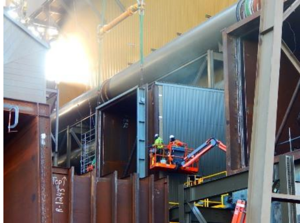
2014-12-09 Insulating ductwork
