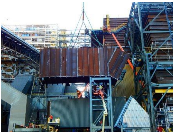
2014-10-07 G26 ID fan 1A discharge ductwork lift
