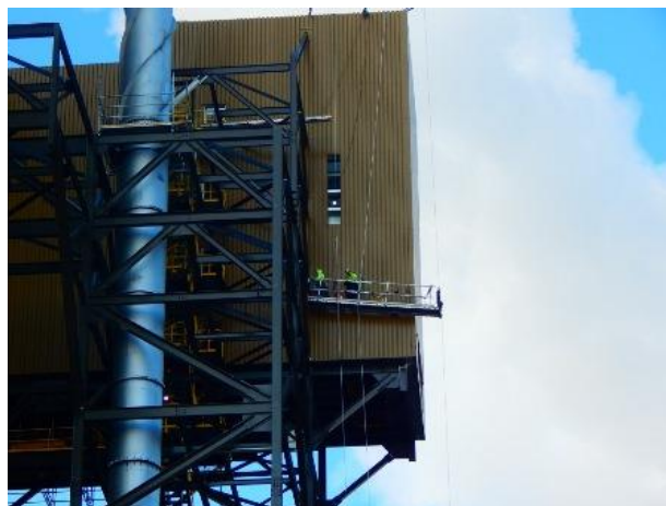
2014-12-09 Siding work continues
