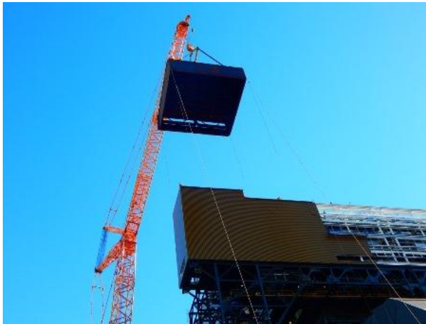
2014-10-14 G3A duct lift
