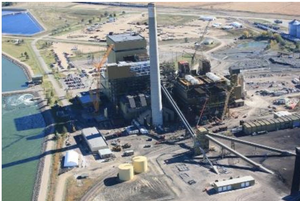
2014-10-15 Aerial view of project
