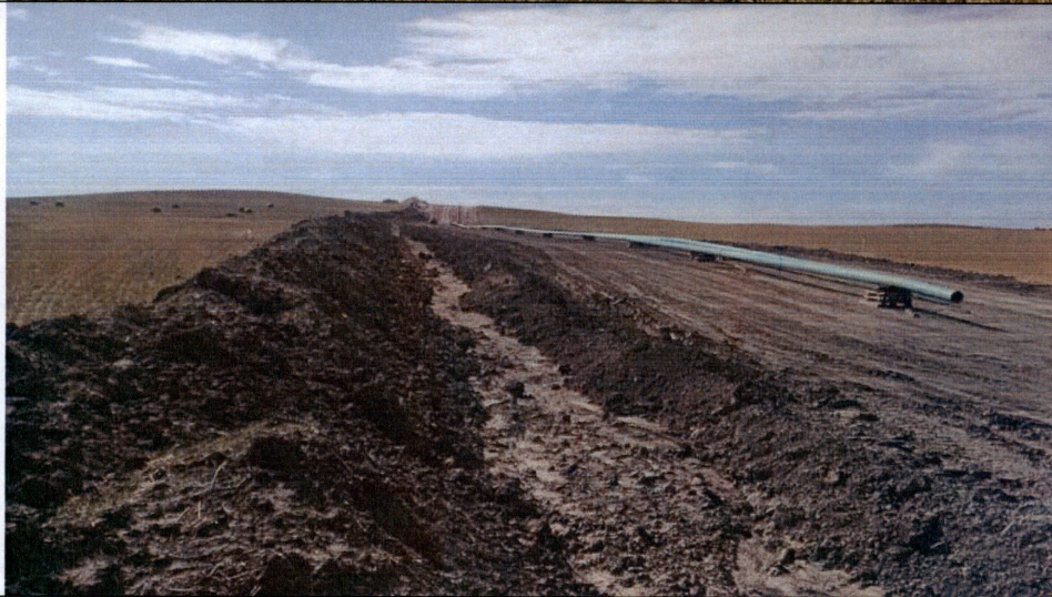
Photo 14: Looking south at Cherry Creek pipe line in Section 8. Topsoil and subsoil windrows are being used to provide a gutter for stormwater control.
