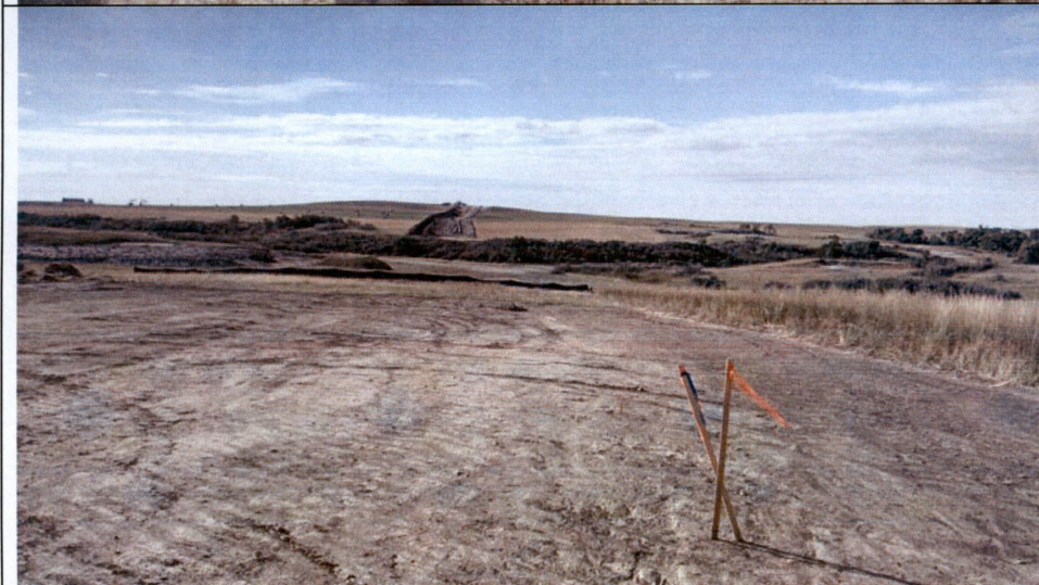
Photo 12: Looking south from the northern end of directional bore, proposed under Wetland 04.
