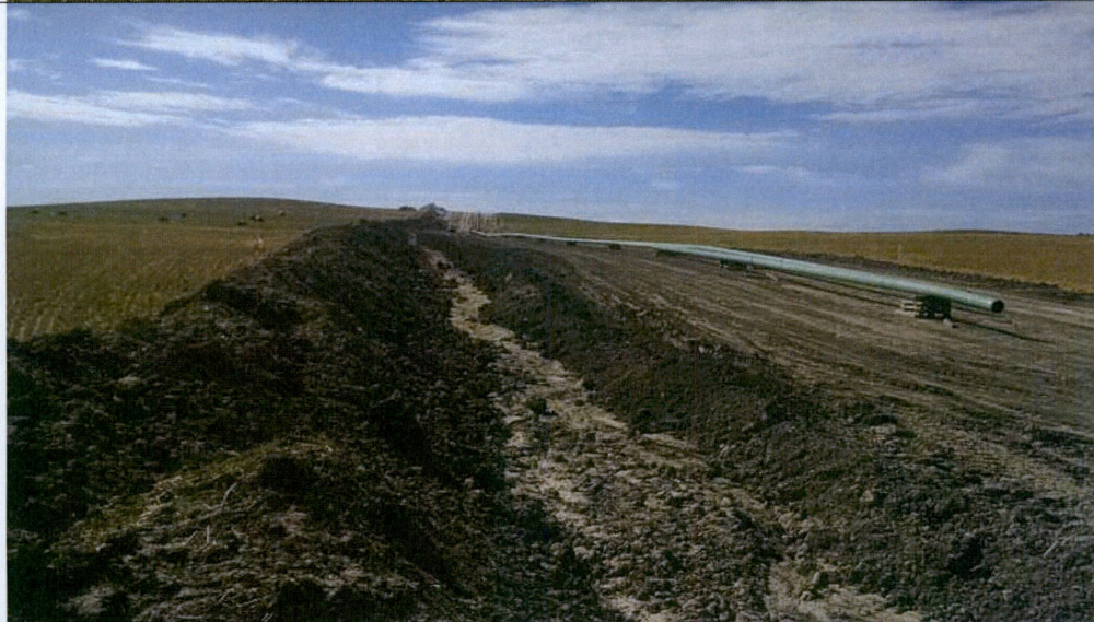
Photo 14: Looking south at Cherry Creek pipe line in Section 8. Topsoil and subsoil windrows are being used to provide a gutter for stormwater control.
