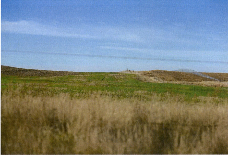
Photo 1: Beginning of pipeline (facing west).
