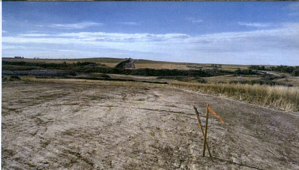
Photo 12: Looking south from the northern end of directional bore, proposed under Wetland 04.
