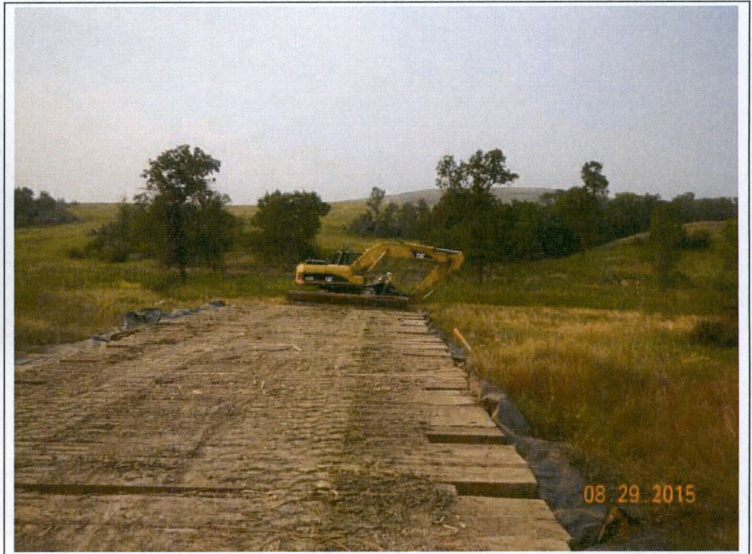
Photograph 4: Viewing southward from Sta. ~118+00 (MP 2.2) at the installation of a travel lane through Wetland 2.
