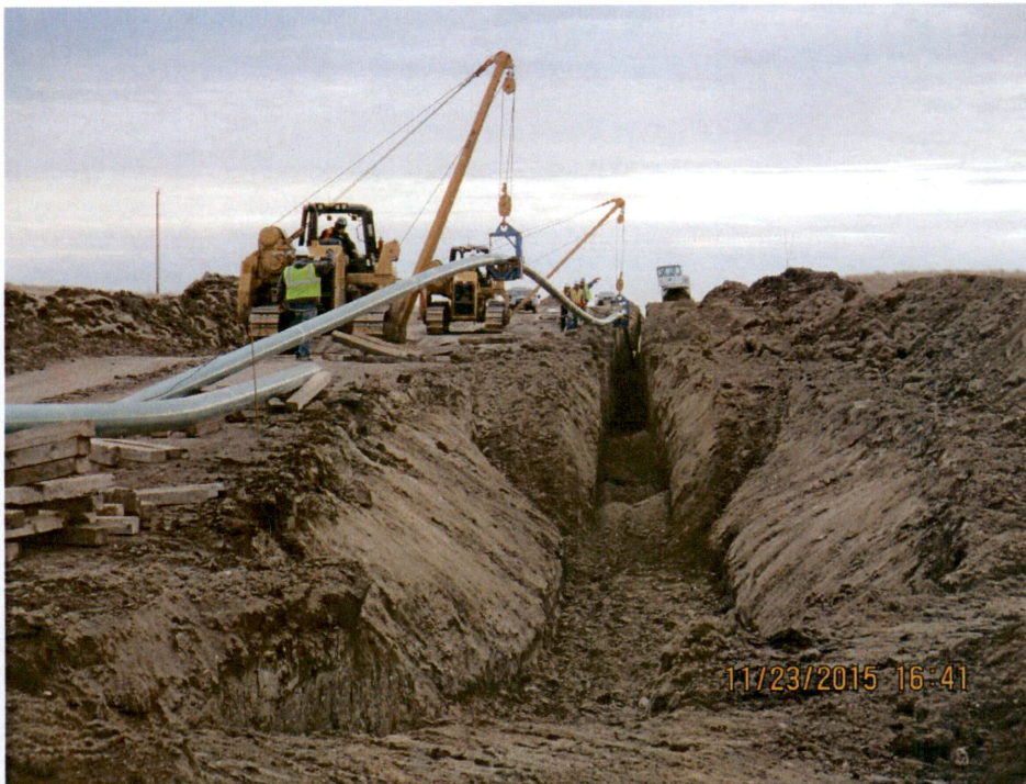
Figure 9. Photo of pipe being lowered into the trench.
