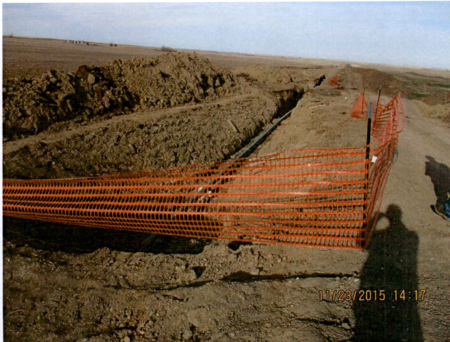
Figure 5. Open trench fenced off. Final coatings on the welds still needed after the tie-ins are made.
