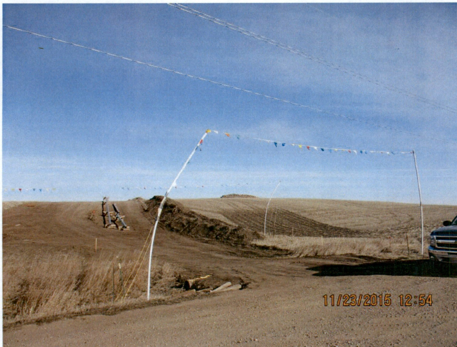
Figure 2. Overhead protection in place while working around the powerlines and preparing to bore under the road.
