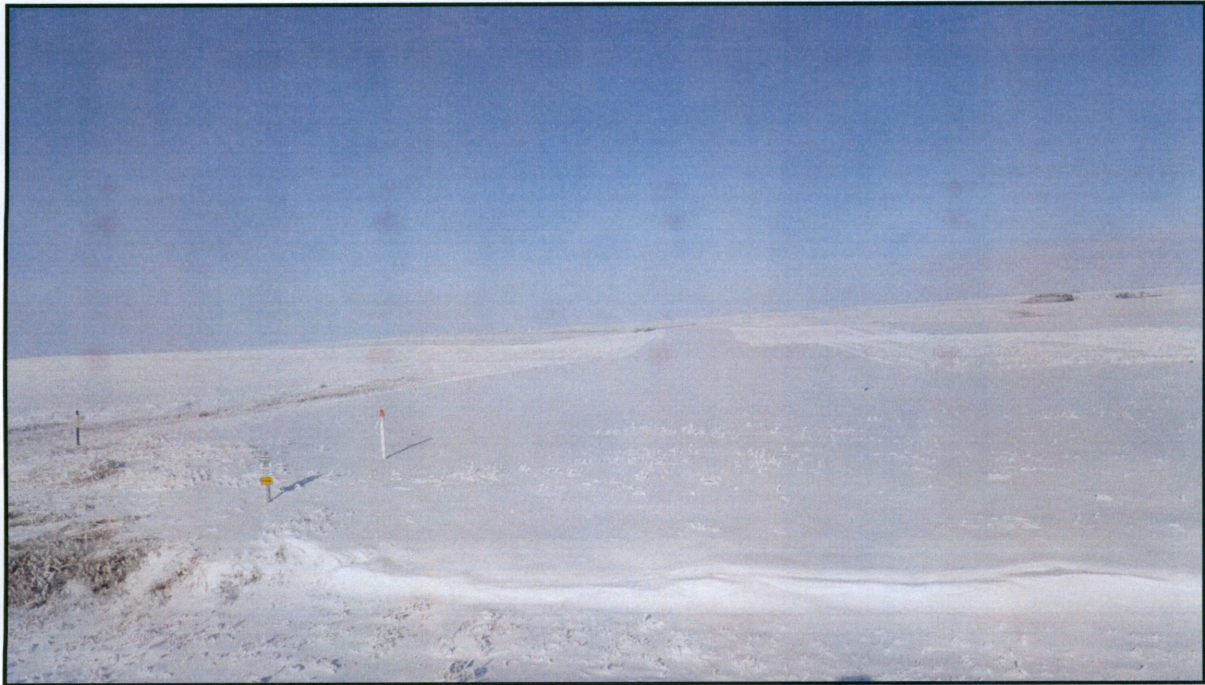
Figure 1. Photo taken of ROW looking north from 64 th Street NW. Test lead for cathode protection and reclamation are visible.
