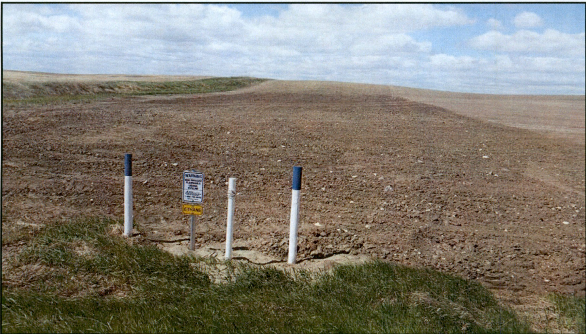
Figure 2. Photo taken look west across Section 15, T160N, R101W from 140 th Ave NW. Reclamation has been complete with pipeline markers in place.
