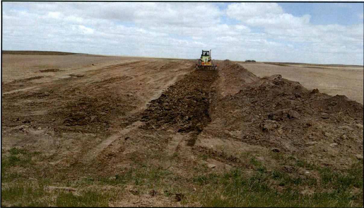
Figure 7. Photo taken facing north from County Highway 12. The ROW is being disced before topsoil is spread.
