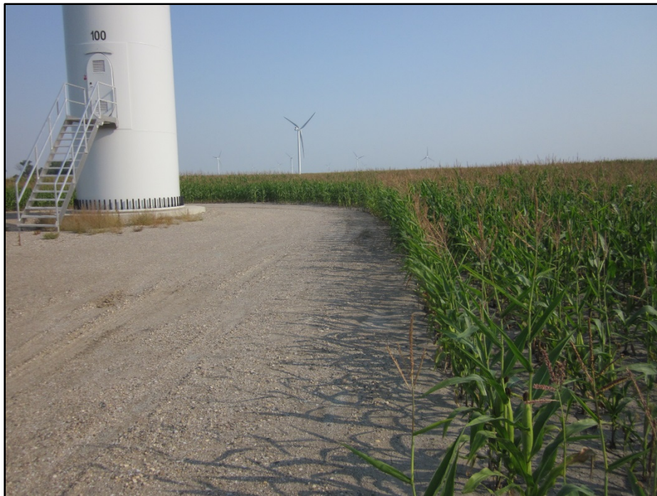
Photo 1. (GPS Point #548) – View of base of Turbine 100. Gravel pad/access road surrounds turbine, there is a 16-ft radius around the turbine for the road/gravel pad. Weeds (brown in color) next to the turbine base by stairs have been sprayed, they will be sprayed in the spring and fall for this project. The corn next to the access road, where it has been reclaimed, is somewhat stunted. Direction: North.
