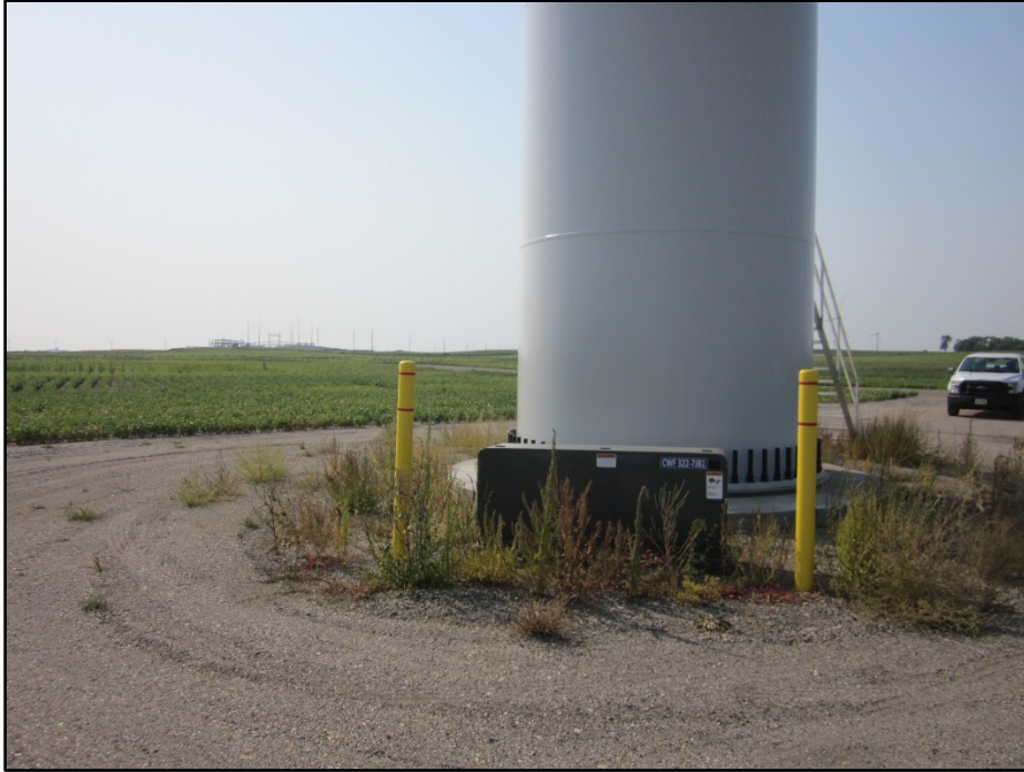
Photo 7. (GPS Point #551) – View of base of Turbine 59. Safety warning signs were in place. Box has two cement bollards and gravel around it. Weeds have been recently sprayed. Direction: Southeast.
