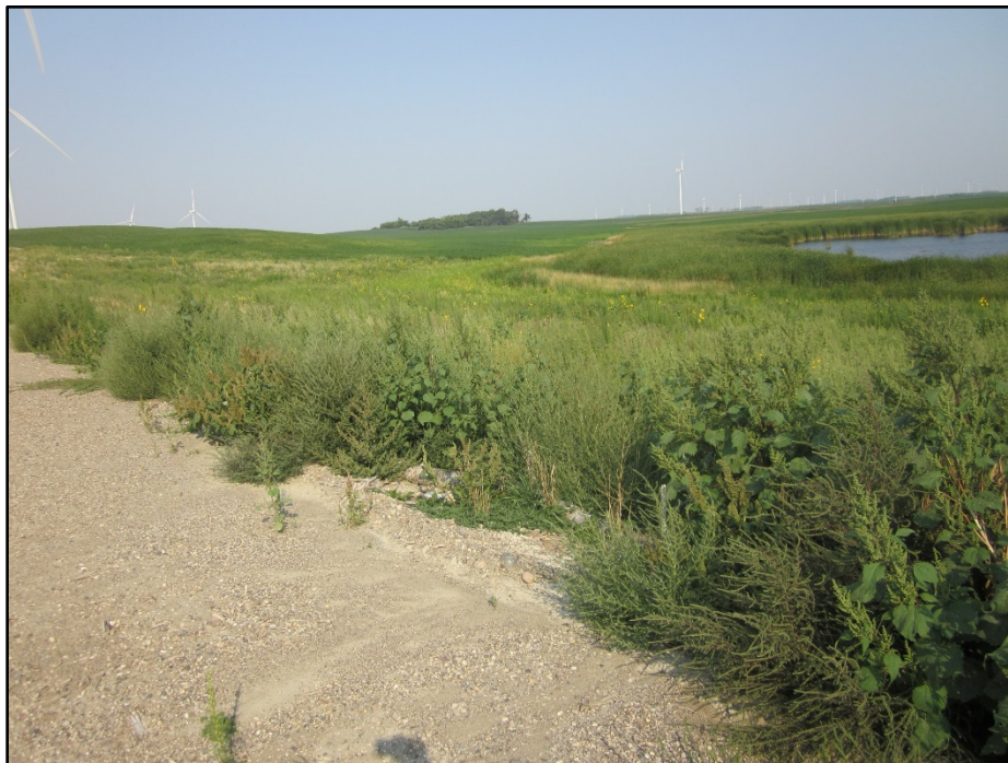
Photo 4. (GPS Point #549) – Access road to Turbines 95-98 (same area as photo above). The access road was cut into side of the hill and this area was reclaimed, it has annual weeds growing which is typical for the 1 st growing season after re-seeding. Note straw wattle by edge of road (weed growth is covering most of the wattle), wetland to the right of photo. Canada thistle (not shown) was observed near the reclaimed area in the county road ditch. Direction: West-northwest.
