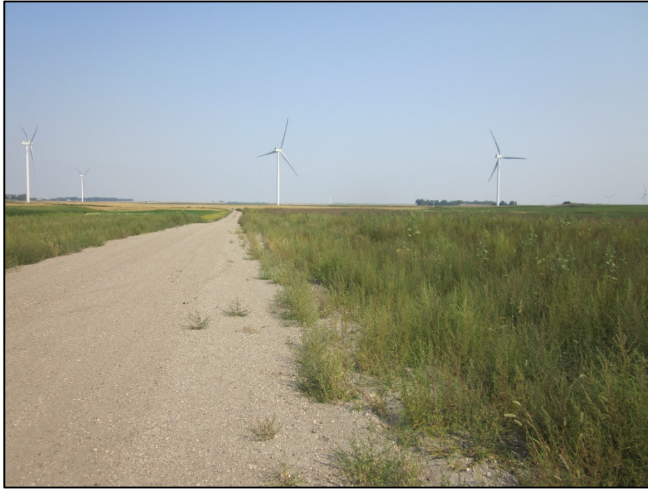
Photo 17. (GPS Point #556) – Access road Near Turbine 31 in CRP land. Direction: South.
