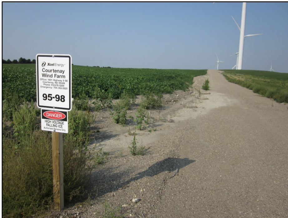
Photo 3. (GPS Point #549) – Access road to Turbines 95-98. Warning sign shown. Straw wattles shown to the left of the access road. This access road was cut into the side of the hill. Direction: West.
