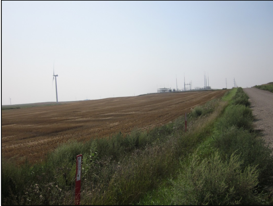
Photo 13. (near GPS Point #553) – View of line markers. Underground line connects to substation. There looks to be a slight unevenness in field, unsure if it is from underground lines, natural topography, or something else. Direction: South.
