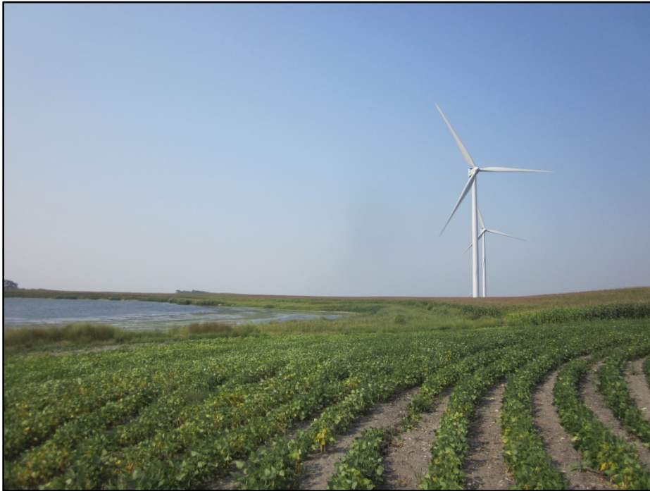
Photo 16. (GPS Point #555) – Near Turbine 49. This area has been reclaimed back to cropland (soybeans). Crops were somewhat thinner or stunted in the reclaimed area. There was previously a silt fence near the wetland. Direction: West.
