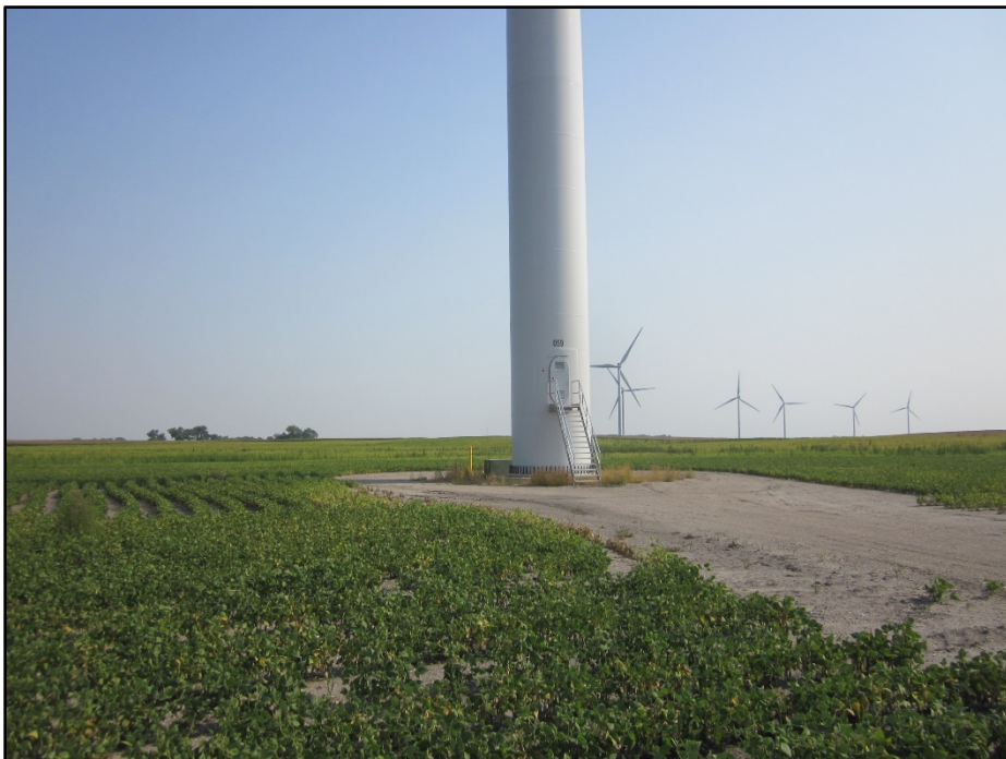
Photo 6. (GPS Point #551) – View of Turbine 59, in soybean field. Crops were coming along well but still somewhat thinner in reclaimed areas. Direction: North.
