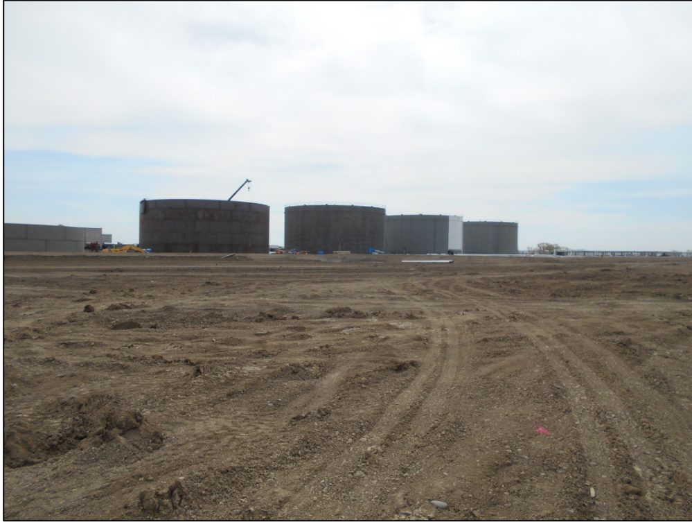
Figure C.11. Overview of proposed Fairview rail facility expansion area, facing southeast (photo taken May 1, 2015).
