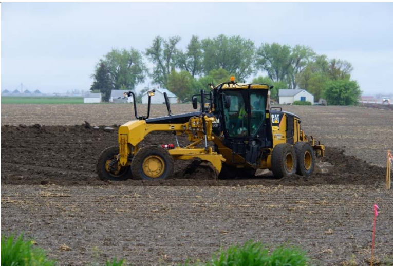
Photo 5: Grader removal depth, Facing south.
