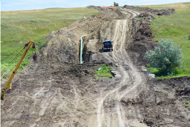
Photo 22: Wetland crossing construction (facing Northeast).
