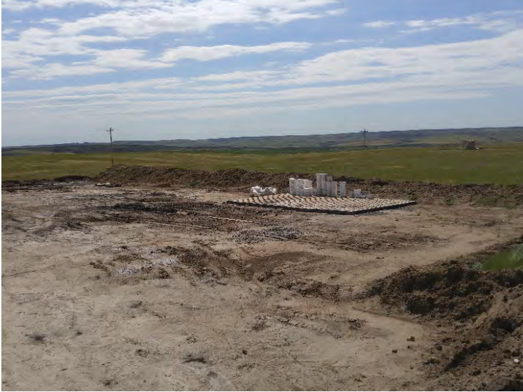
Photo 12: Material staging area (facing Southeast).
