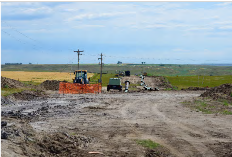
Photo 11: Pipe laydown (facing East).
