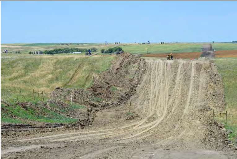
Photo 23: Topsoil pile and corridor preparation (facing West).
