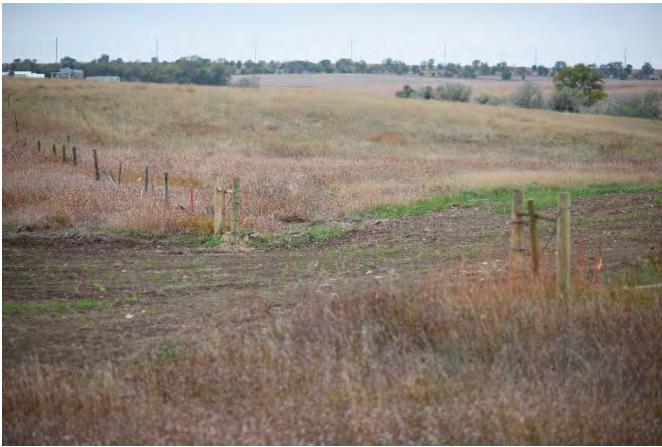
Photo 13: Fence repair facing northwest
