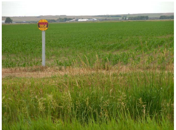
Photo 14: Pipeline corridor and signage facing west at 159 th Avenue NW.
