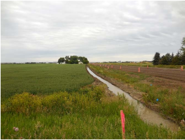
Photo 1: Corridor facing south near Highway 58, on far west side of project.
