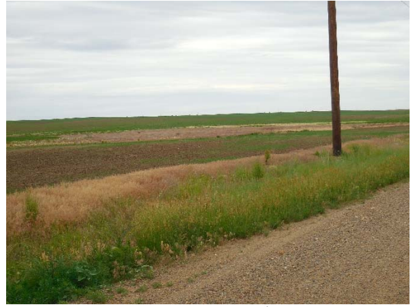
Photo 29: Pipeline corridor from 34 th Street NW, facing east northeast. Grading footprint is visible.
