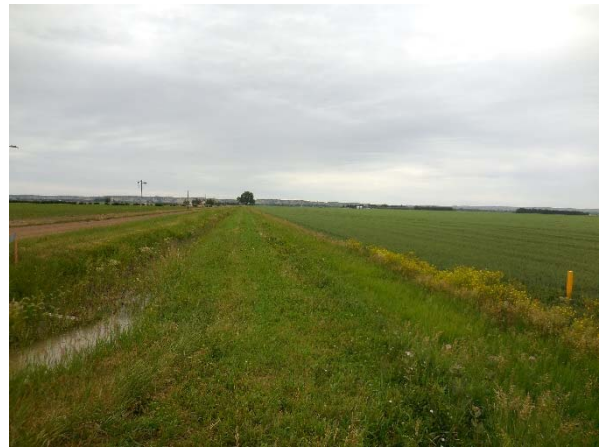
Photo 2/3: Pipeline corridor facing east, at 32 nd Street NW, near far west side of project.
