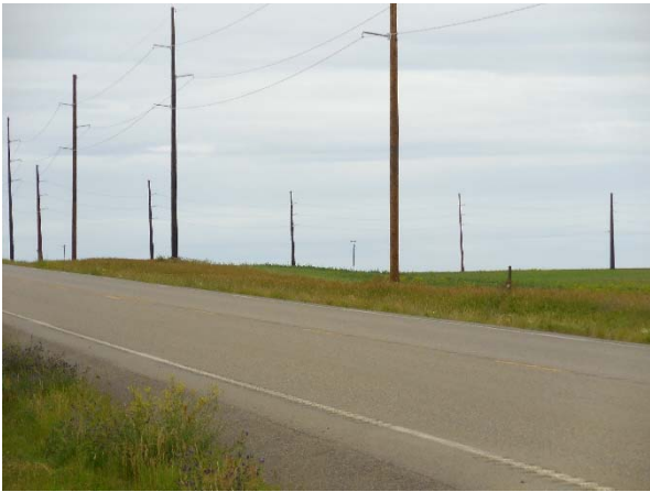
Photo 20: Pipeline corridor on the east side of Highway 16.
