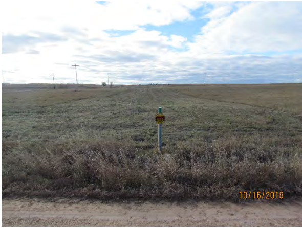
Photo 65: Fence repair facing west
