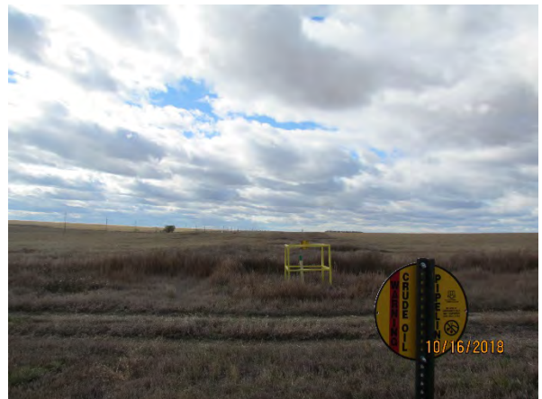
Photo 34: Reclamation facing west
