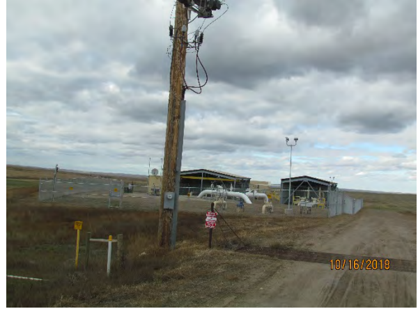
Photo 42: Reclamation facing north/northwest.
