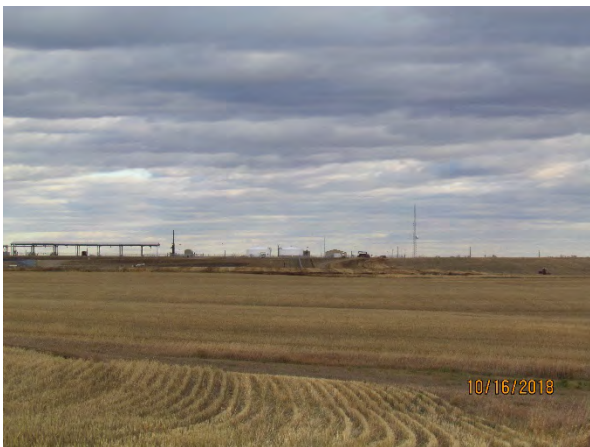
Photo 69: Reclamation facing east towards eastern project termini.
