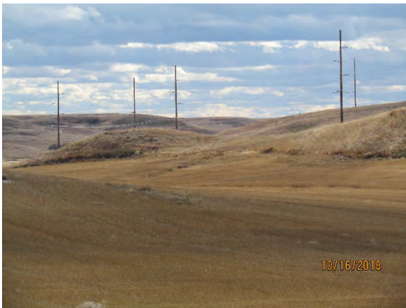
Photo 31: Reclamation facing southwest.
