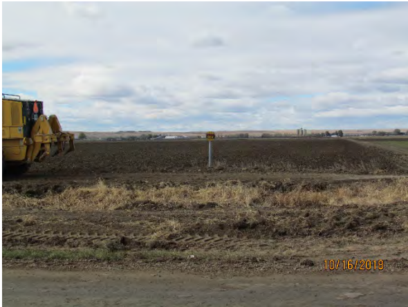
Photo 13: Reclamation facing west.
