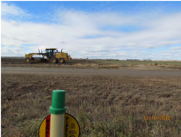
Photo 15: Reclamation facing west.
