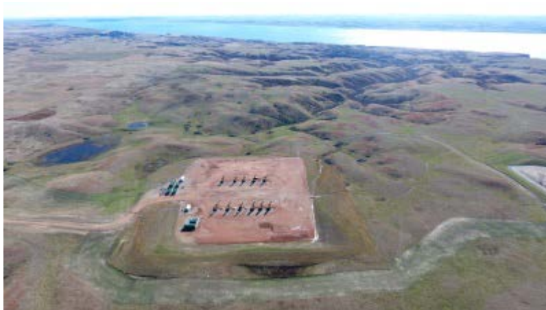
Picture 47: Station 705+50.00; Latitude: 48° 8'38.37"N Longitude: 102°41'16.04"W Looking south, pipeline crosses near center of picture
