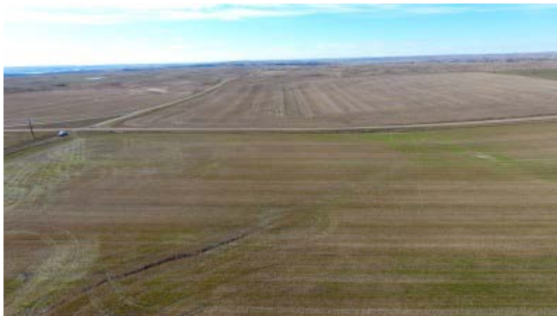
Picture 35: Station 430+40.00; Latitude: 48°11'1.56"N Longitude: 102°41'46.31"W Picture looking west, pipeline at left side of field
