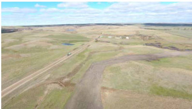
Picture 59: Station 1809+00.00; Latitude: 48° 0'9.62"N Longitude: 102°26'18.13"W Looking north, pipeline is the less visible scar to the left, some weed growth present
