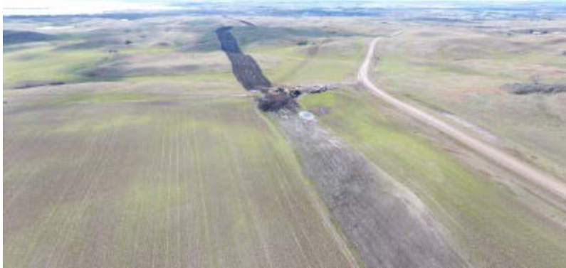
Picture 60: Station 1813+10.00; Latitude: 48° 0'5.53"N Longitude: 102°26'16.17"W Looking south, pipeline between road and pipeline currently being reclaimed
