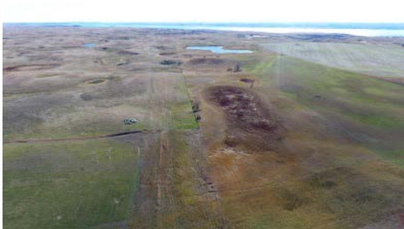
Picture 42: Station 670+70.00; Latitude: 48° 9'12.83"N Longitude: 102°41'17.19"W Looking south, pipeline in center, then to the turning to the right side of picture
