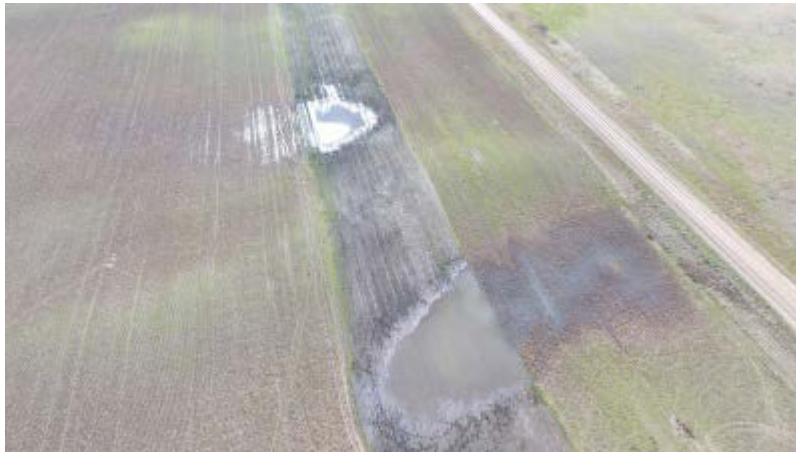
Picture 58: Station 1806+15.00; Latitude: 48° 0'12.47"N Longitude: 102°26'18.09"W Picture looking to the south, pipeline near road (prominent scar from a different pipeline)
