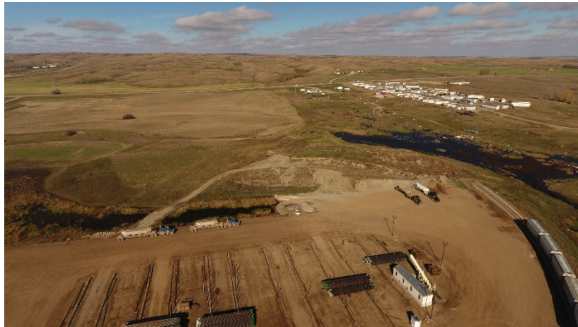
Picture 74: Station 2050+00 Latitude: 47°58'19.1244" N, Longitude: 102°26'35.8800" W Looking north, pipeline in center of picture
