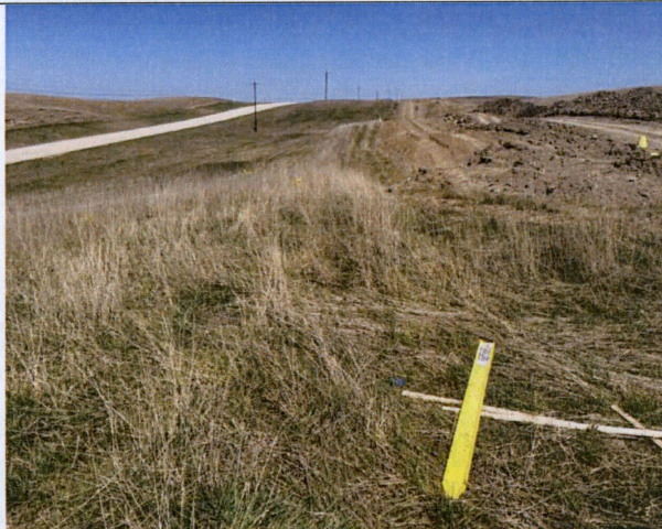
Photo 3- Site 75 (pipeline on left side of active construction)
