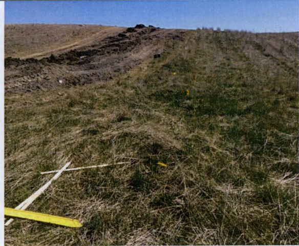
Photo 4- Site 75 (pipeline on right side of active construction)
