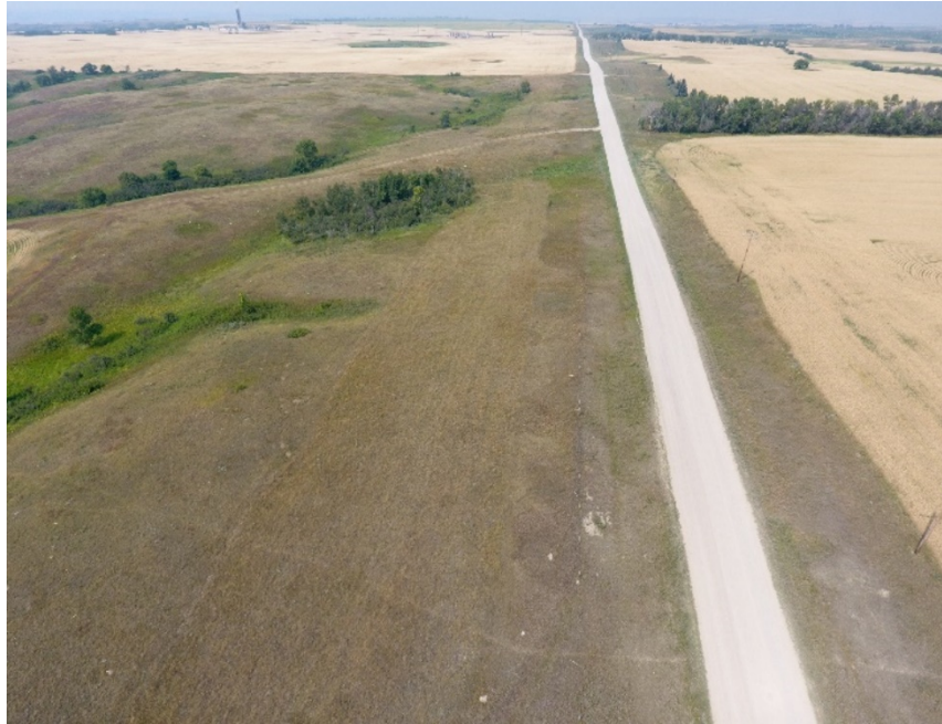
Location 85, looking North (48.214714, -102.699112) Scar visible on West side of road, well established, matching existing conditions
