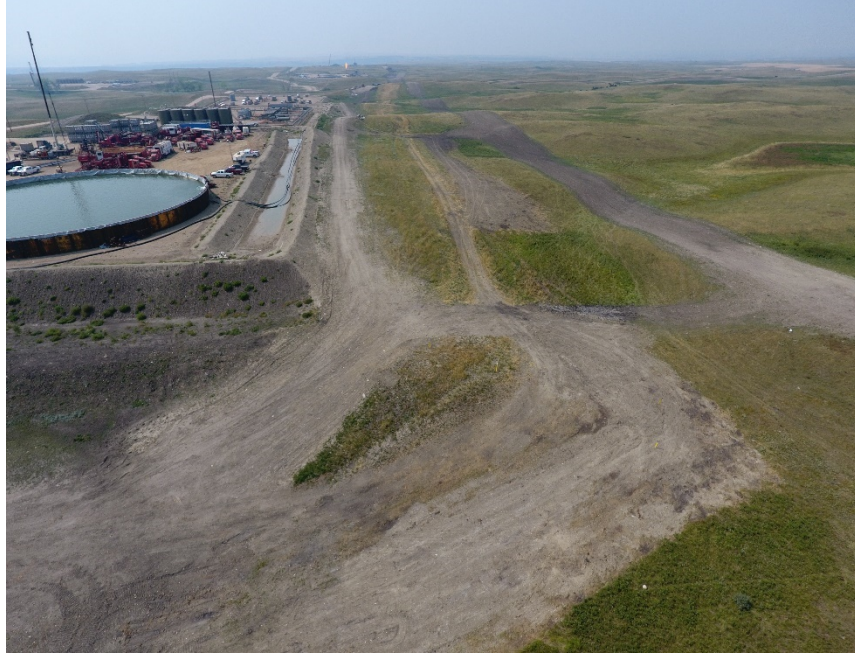
Location 71, looking North (48.169628, -102.687805) Scars showing recent work adjacent to pipeline
