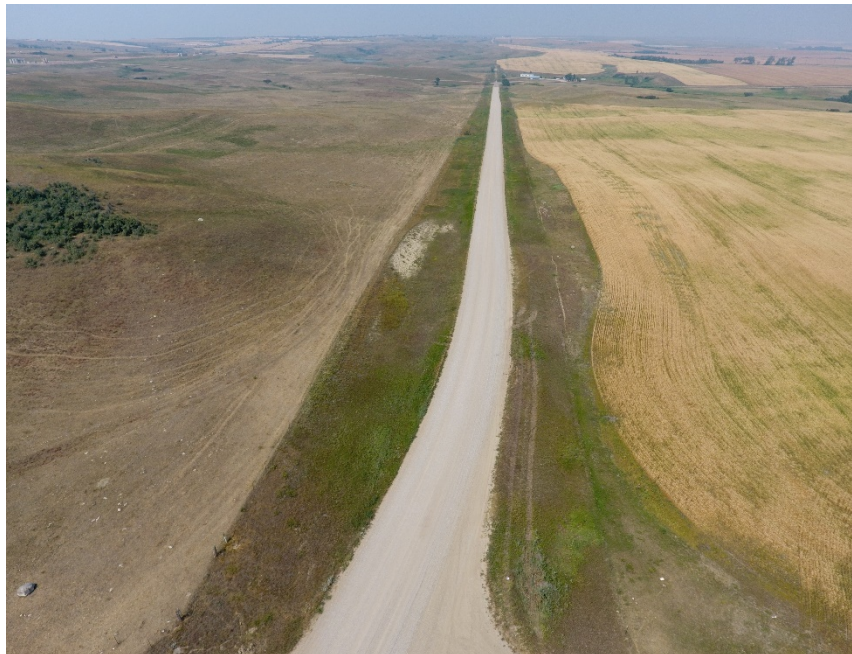
Location 4, looking North (47.999111, -102.439659) Pipeline at right, not detectable
