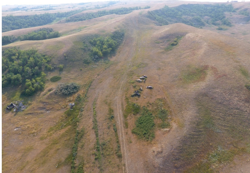
Location 29, looking West (48.049789, -102.566978) Grass well established and blending with existing conditions
