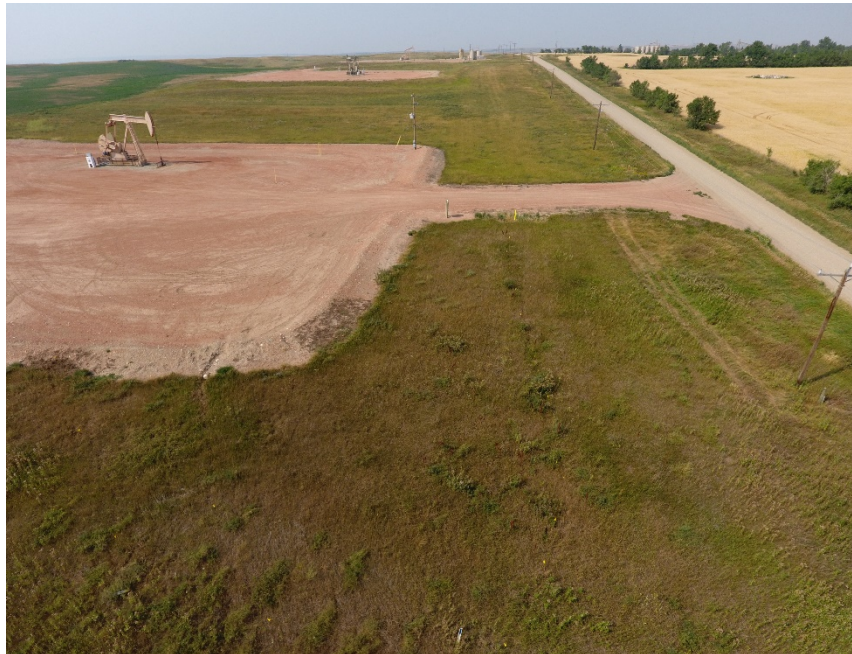
Location 16, looking North (48.03051, -102.461983) Little or no evidence of pipeline work after reclamation
