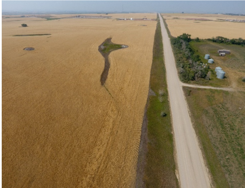
Location 97, looking North (48.29163, -102.656204) Pipeline at West side of road. No reclamation issues in farmland
