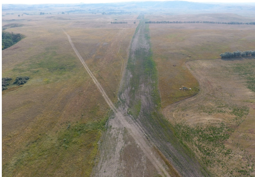
Location 26, looking West (48.055264, -102.54528) Visible scar from adjacent pipeline noted at Location 25
