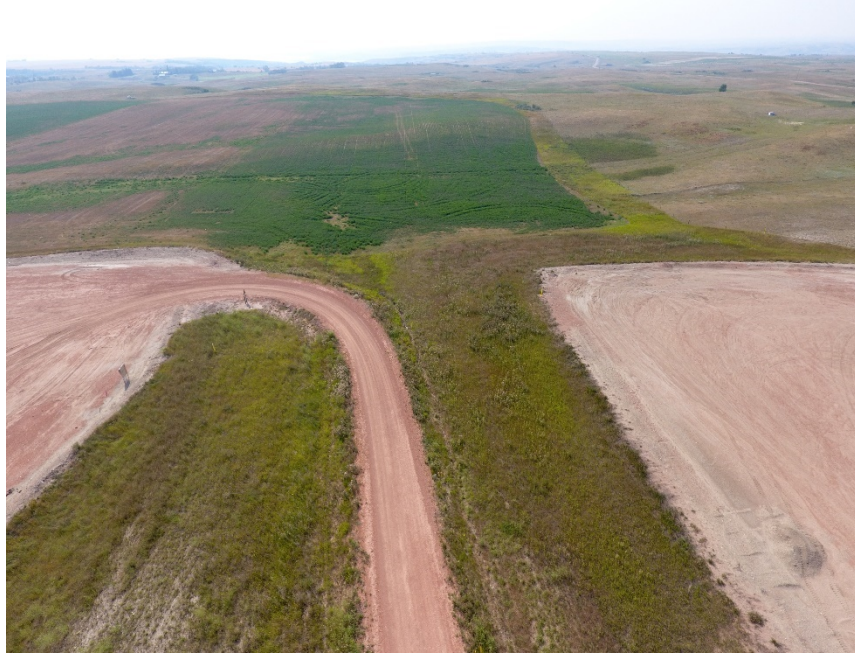
Location 17, looking West (48.034012, -102.462486) Pipeline marker visible at corner of pad, vegetation well established. Strip of noticeable change in vegetation extending straight west is not on this pipeline alignment
