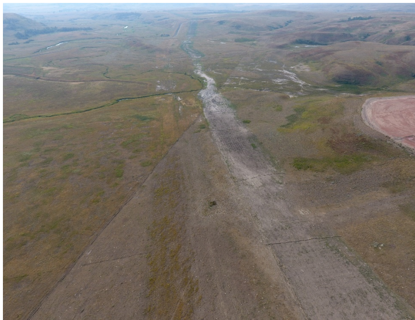
Location 24, looking West (48.053711, -102.525238) Scar at left side in photo
