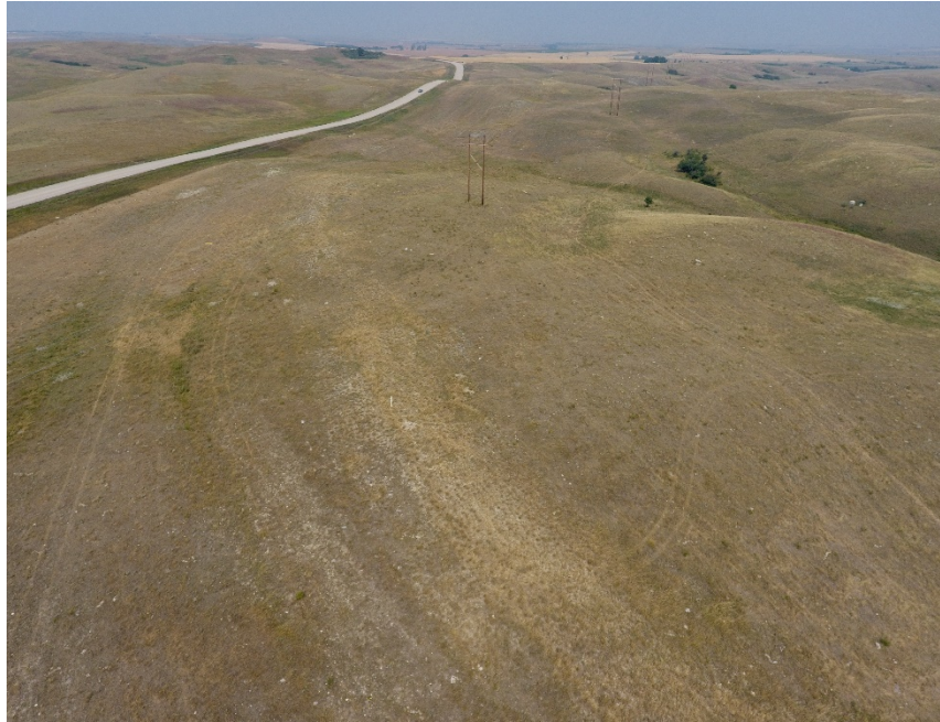
Location 3, looking Northeast (47.993015, -102.445267) Pipe marker visible in center of picture, scar nearly undetectable in distance
