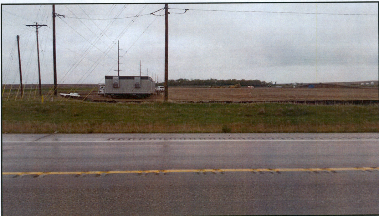
Figure 2. Photo taken looking west from Hwy 40 across the lay down yard in Section 3, T158N, R95W.
