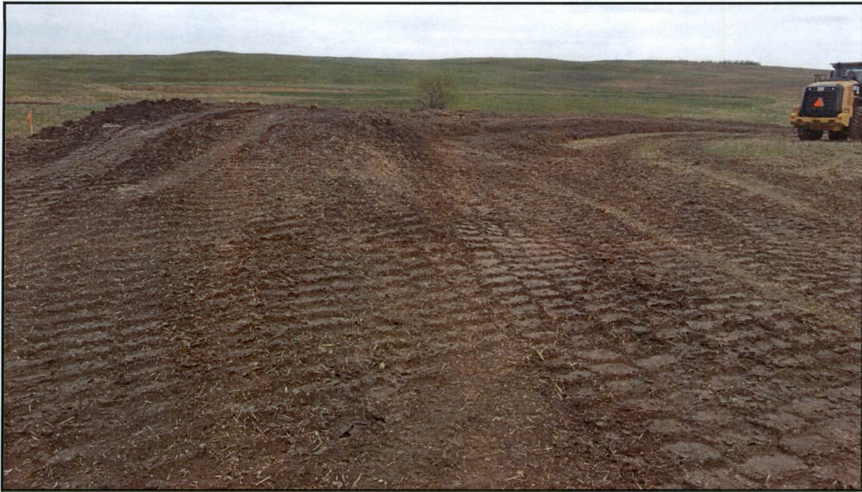
Figure 5. Photo segregated topsoil for Turbine B-10 pad.
