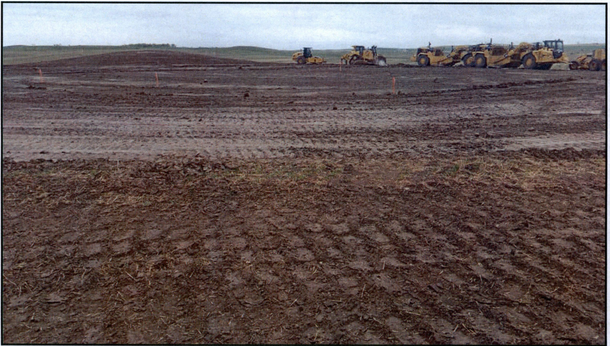
Figure 4. Photo of pad for Turbine B-10.
