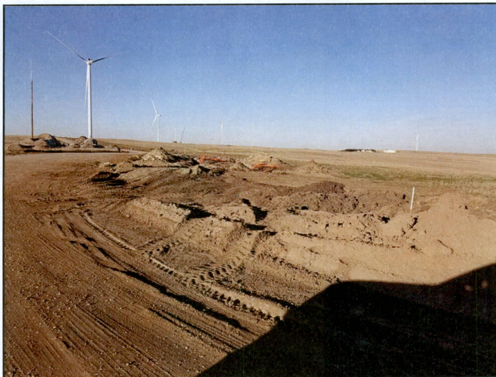
Figure 10. Photo taken facing north along the access road to turbine F7. Electrical cable and junction box installation is underway.
