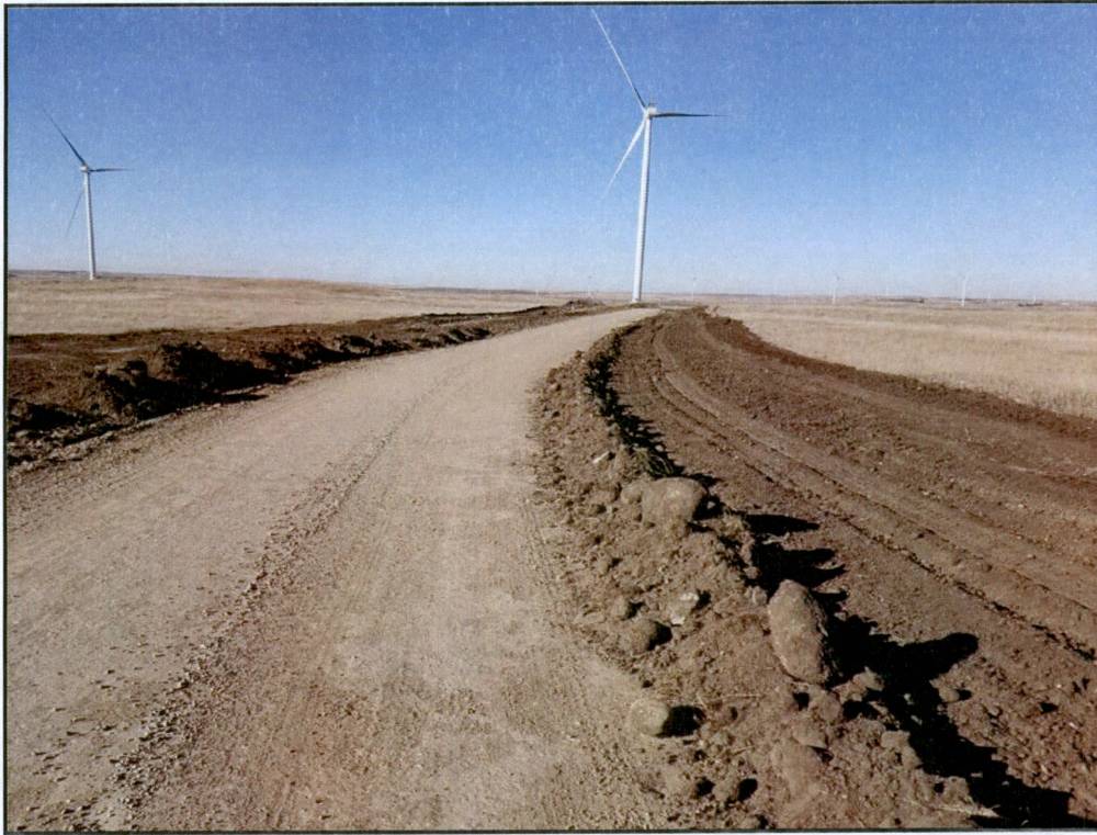
Figure 2. Photo taken facing northwest towards turbine B8. The access road has been surfaced at a width of 16-feet and topsoil redistributed on the shoulders.
