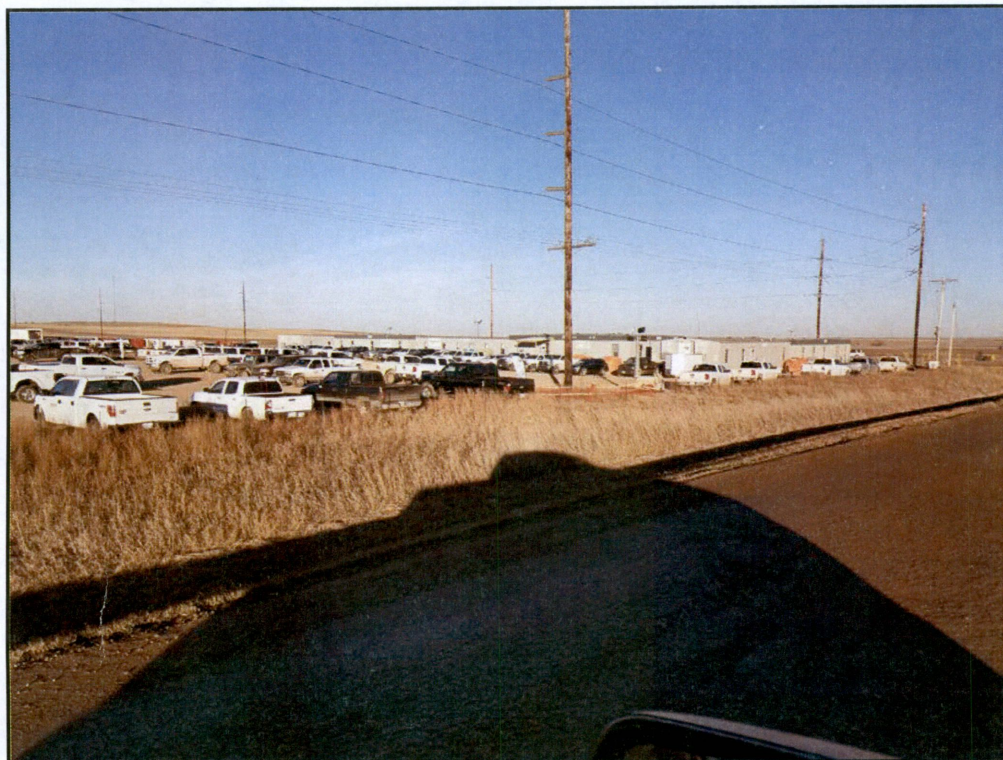
Figure 9. Photo of the completed Laydown Yard.
