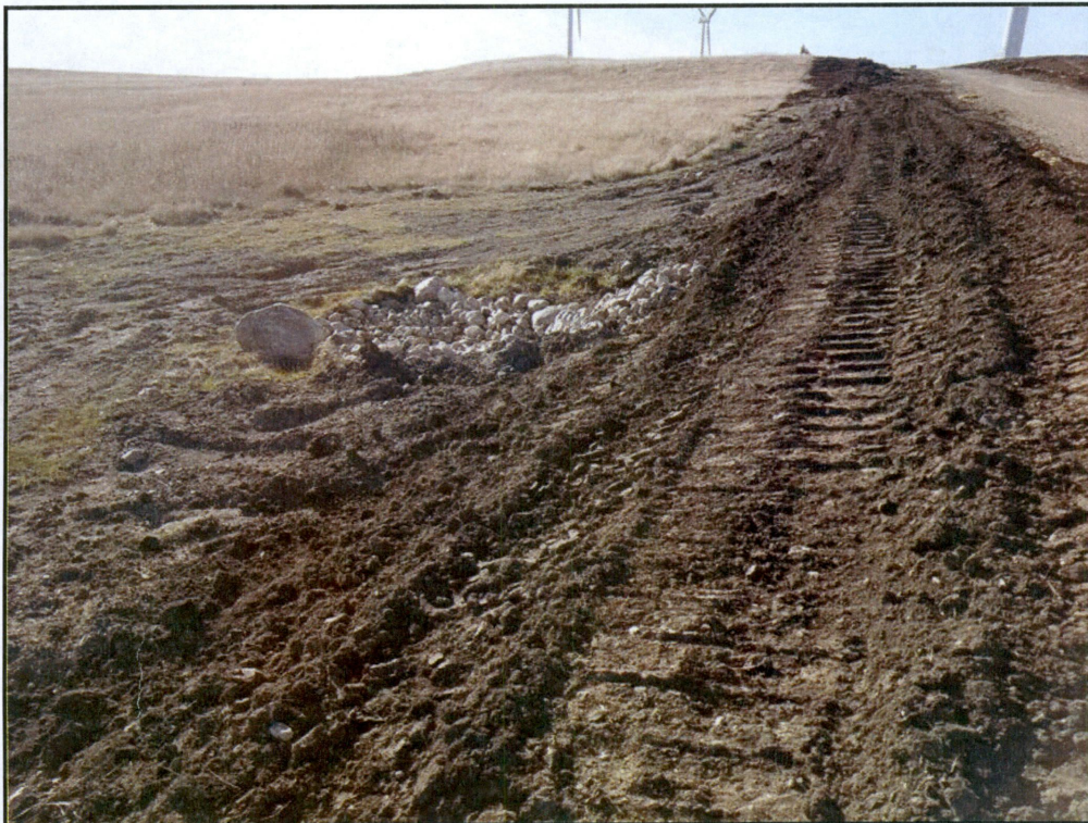
Figure 3. Photo taken east of turbine B6 documenting rock placed around culvert for erosion control.
