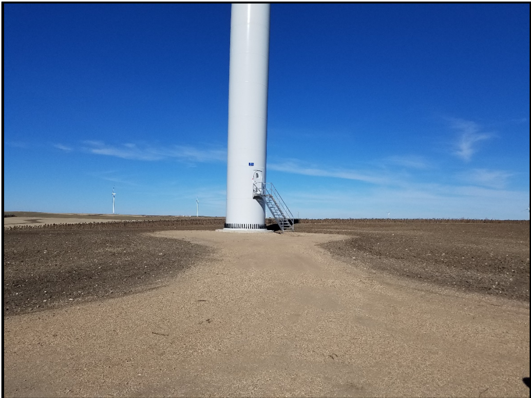
Photograph 6. View the reclaimed pad of Turbine E4 in the N1/2, Section 17, T158N, R95W.
