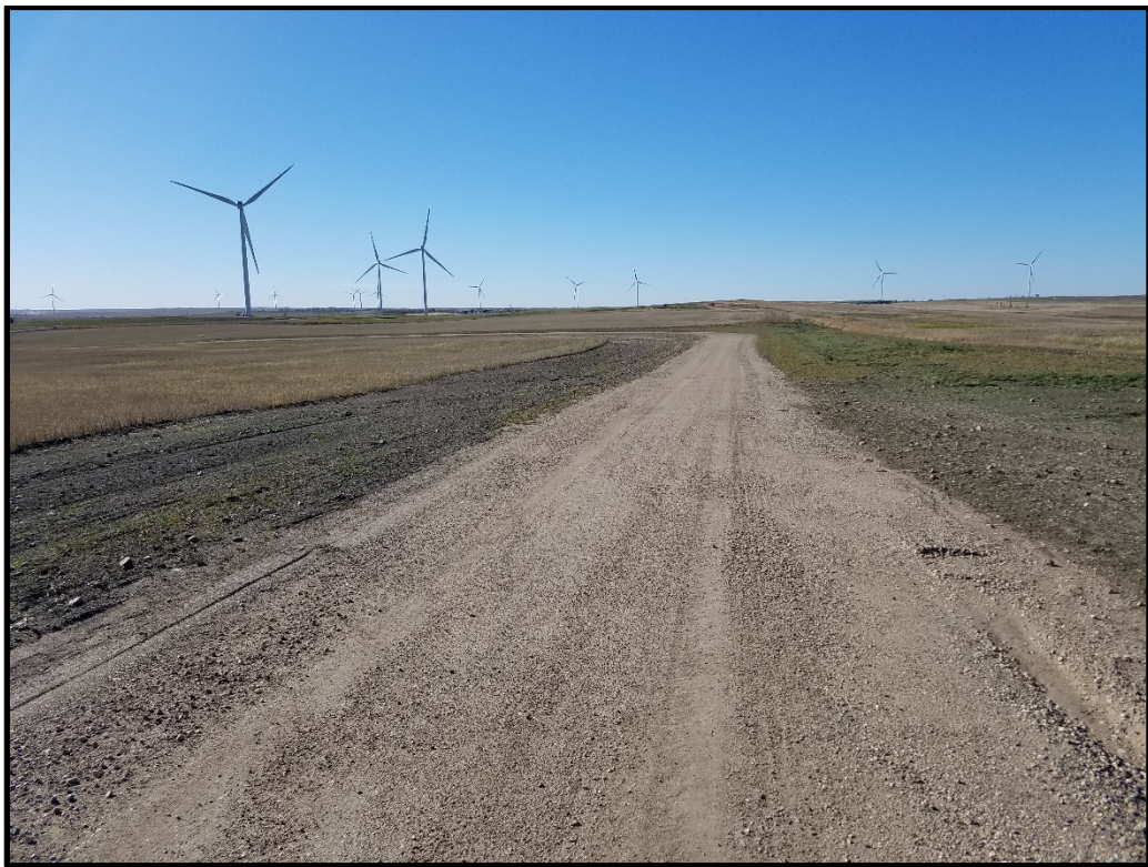
Photograph 2. View looking west along the access road to the "G" string of turbines in Section 3, T158N, R95W. Turbines 09, 10, 11, 12 can be seen.
