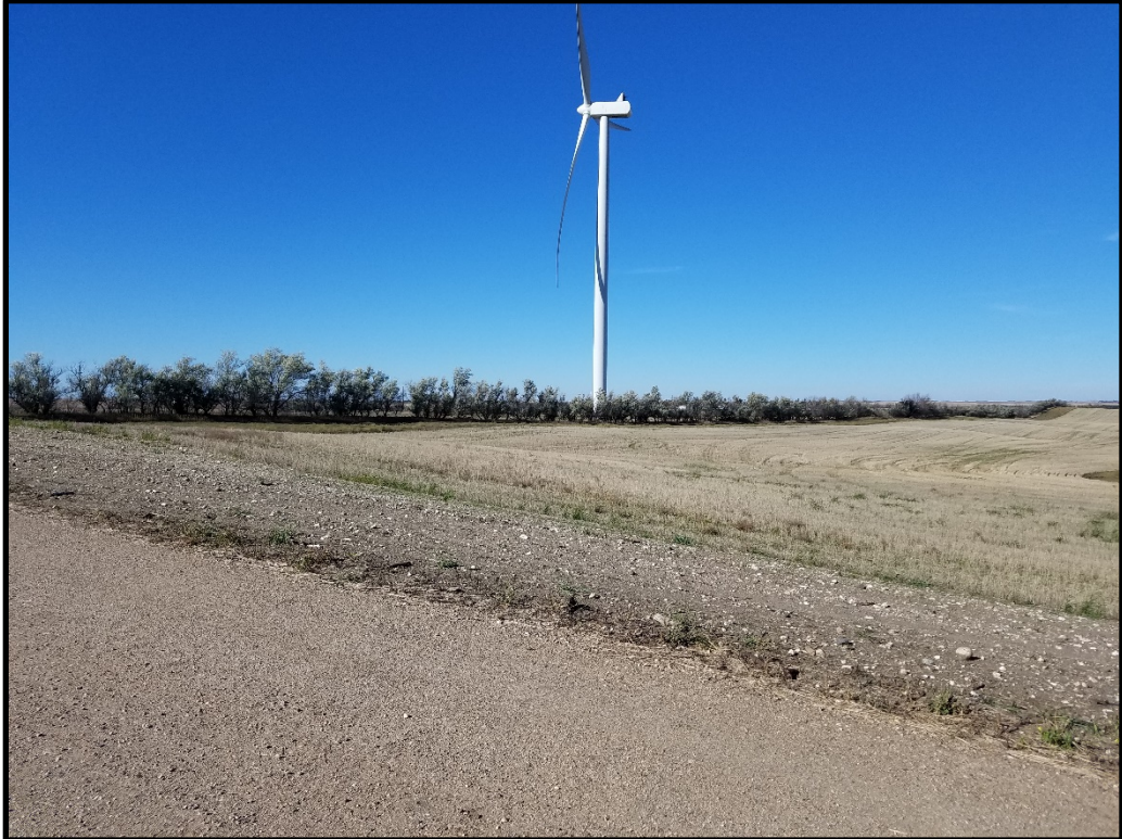
Photograph 10. View looking NW at Turbine D7 in Section 26, T159N, R95W.
