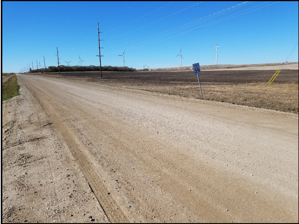
Photograph 3. View looking northwest at the reclaimed laydown yard in Section 3, T158N, R95W.
