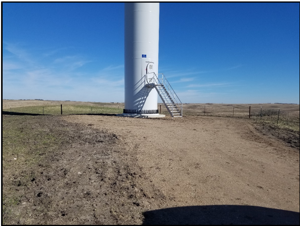
Photograph 8. View of the reclaimed pad and base of Turbine B5 in the SE1/4 of Section 28, T158N, R95W.
