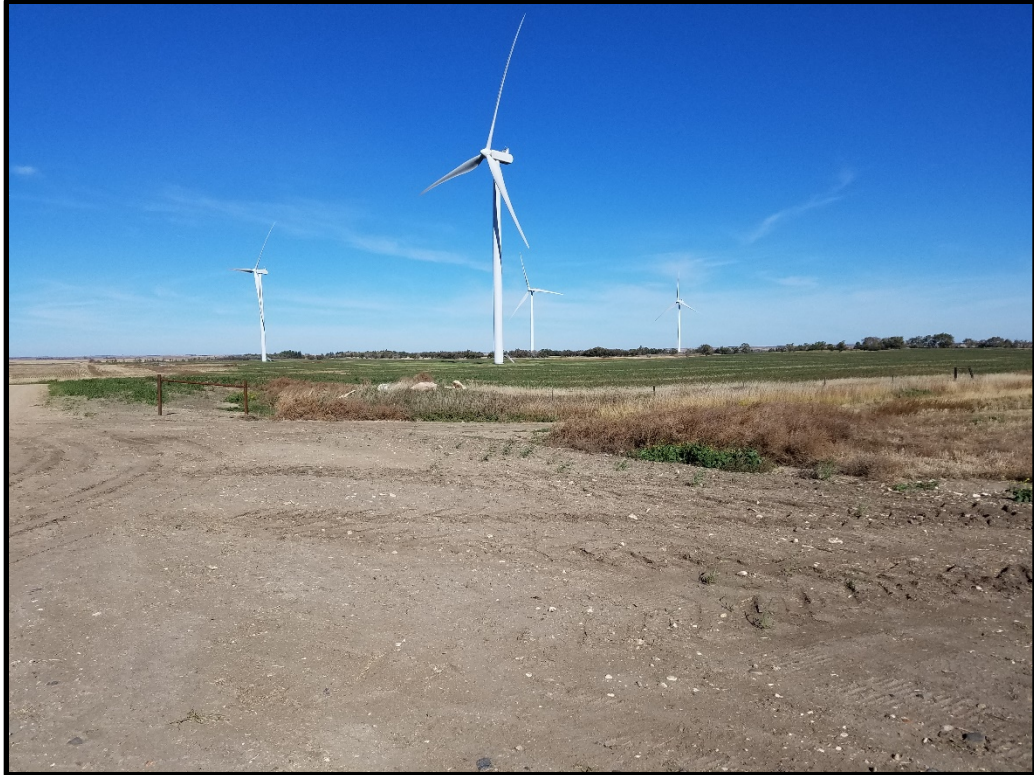
Photograph 1. View looking north at the "C" string of turbines in Section 21, T159N, R95W.
