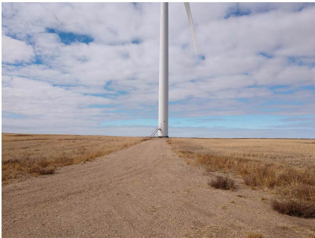
Photo 3. Photo taken looking west towards Turbine C3.
