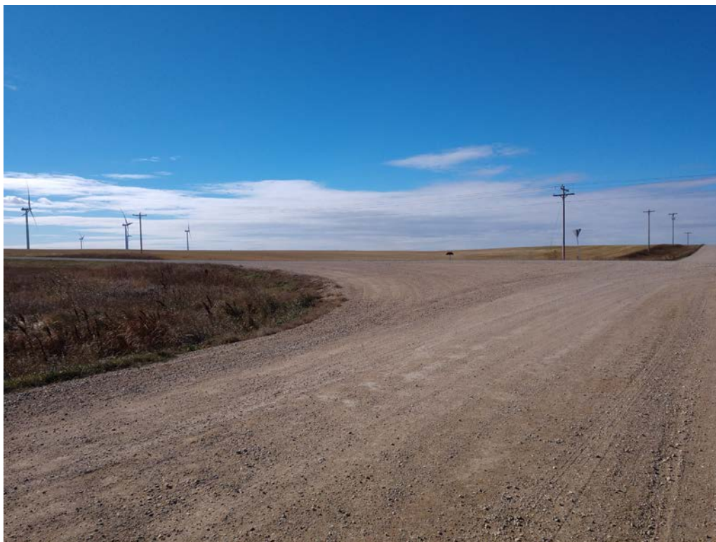
Photo 5. Photo of County Road 21 and 77 th St. NW intersection (facing southwest). Widened turning radius was left in place at request of the County.
