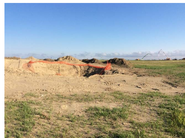
Near station 204+38 pipeline connection and rehabilitation will need to follow
