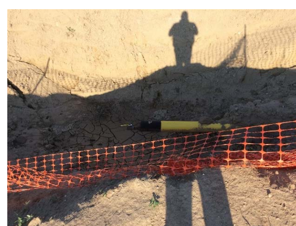
Near station 204+38 pipeline stub.
