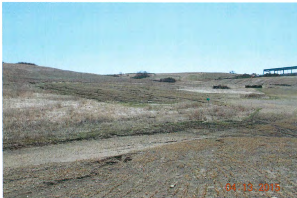
Figure 2. Erosional rilling requiring repair on SPGM stockpiles and the surrounding associated disturbance areas in Section 30 in Permit NACC-1301 - facing southeast toward stockpile TS-3 with the mine office-shop building frame in background – refer to Figure 5 for location
