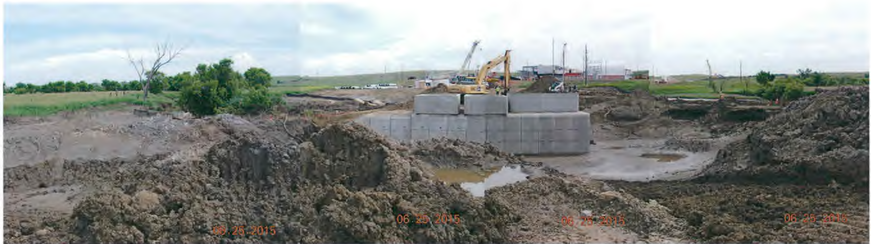
Figure 2. The first of two double box culverts being installed - facing easterly.
