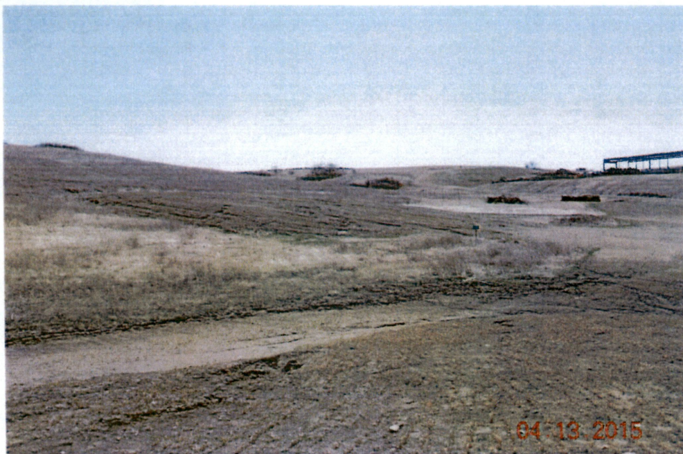
Figure 2. Erosional rilling requiring repair on SPGM stockpiles and the surrounding associated disturbance areas in Section 30 in Permit NACC-1301 - facing southeast toward stockpile TS-3 with the mine office-shop building frame in background – refer to Figure 5 for location
