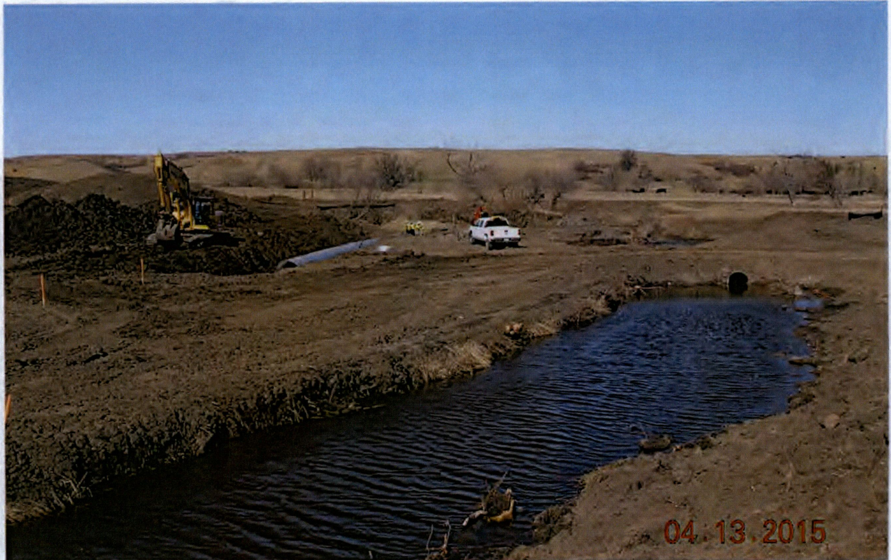
Figure 2 – Low flow culvert installation in progress on Coyote Creek on April 13, 2015
