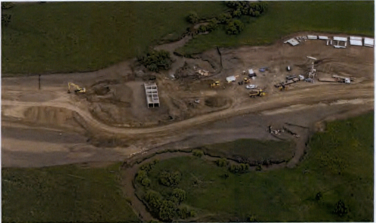
Figure 1- Coyote Creek at access road crossing site taken during June 25, 2015 flyover inspection
