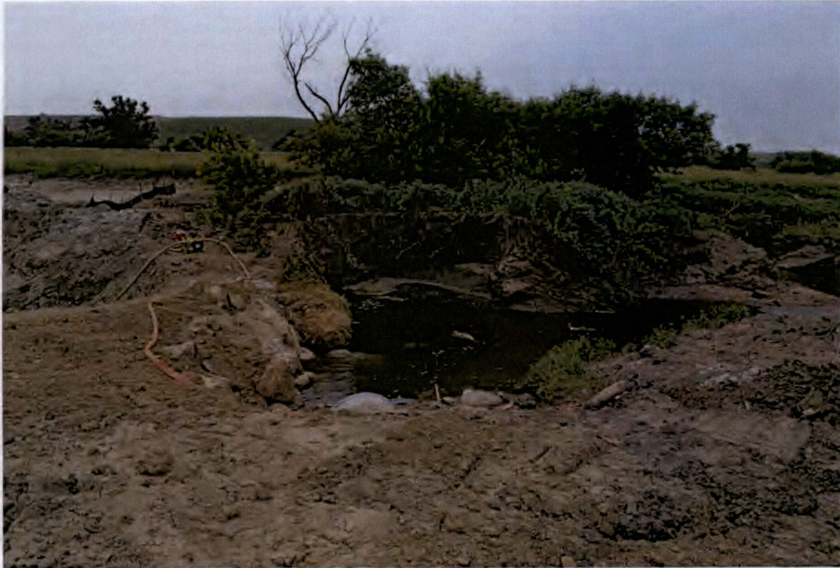
Figure 3- Erosion to stream bank, center. Channel plug and box culvert site to the left.
