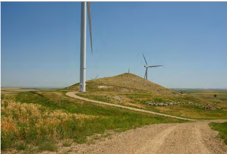
Photo 25: Tower 10 (facing East).
