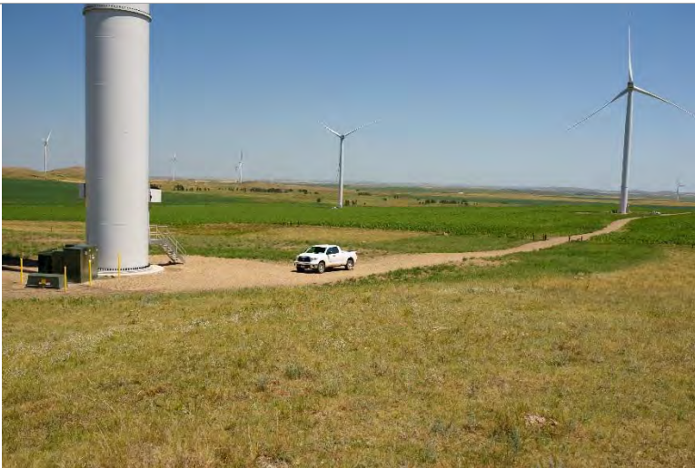
Photo 30: Tower 18 (facing East).
