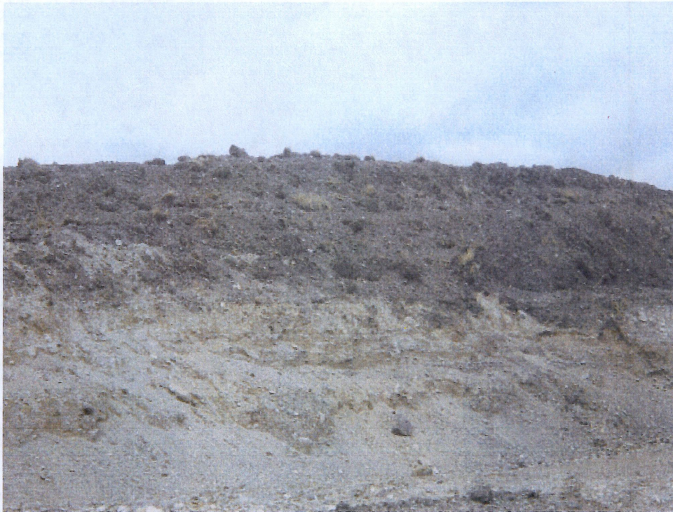
Above: Photo 27- Looking at north side of right of way at station 144+00. Photo shows top soil location with lighter subsoil deposits mixed in with top soil.
