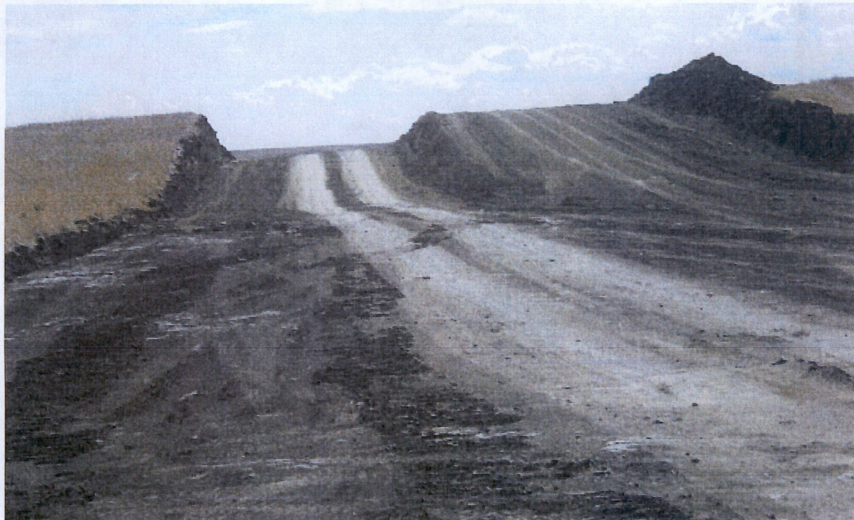
Below: Photo 4- Looking south at hillside located at station 120+00. Right of way has been stripped with top soil located at west side of right of way.
