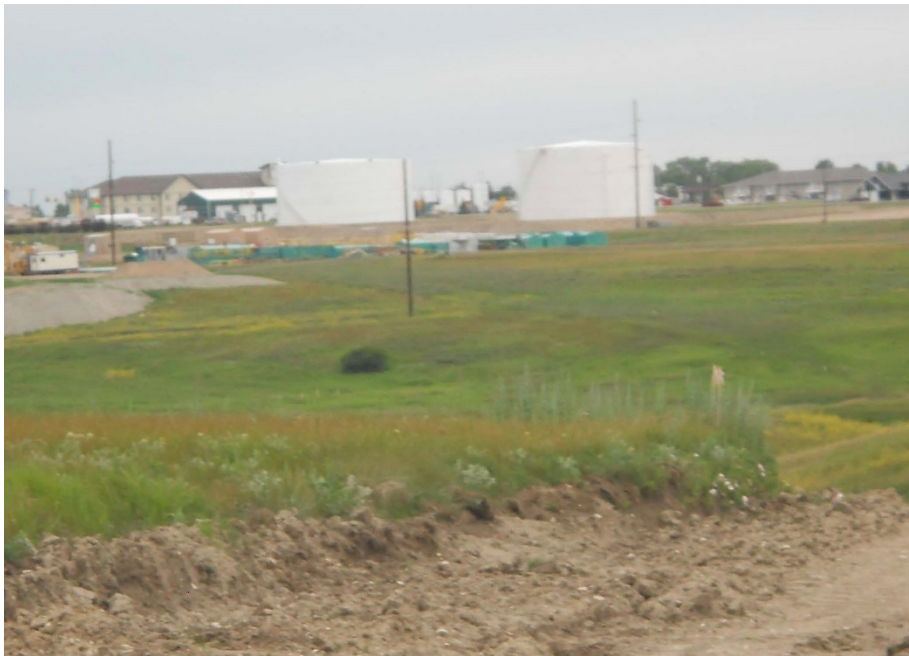
Photo 34 - Located at station 423+56.8, End of Pipeline, photo looking south west at exit bore site across wetland towards tie-in at Enbridge tanks at Stanley, ND.
