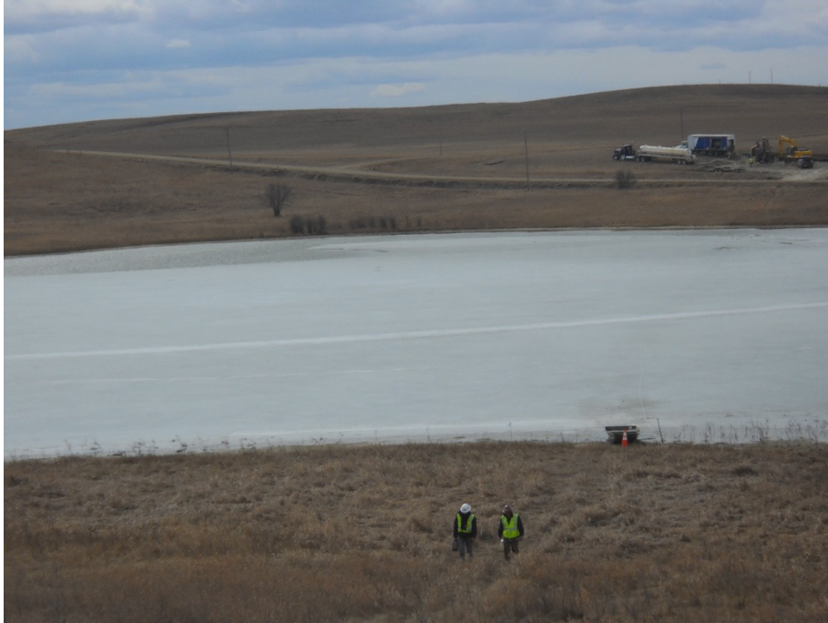
Photo 19 - Located at station 148+00, standing on west hillside, looking across waterway slough to be bored due to nesting habitat.
