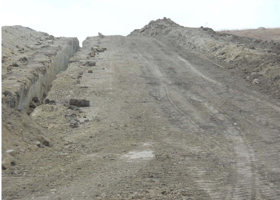
Photo 5: Located at station 34+00, looking east at graded Right of Way, with top and subsoil pushed off edge of Right of Way trenching was underway. No pipe has been stringed out on Right of Way.
