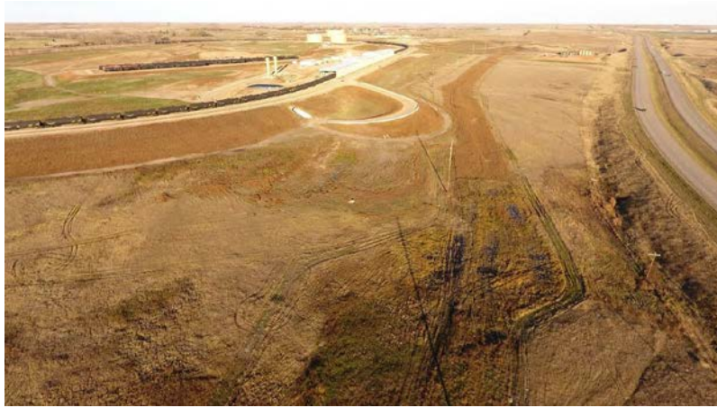
Photo 79: Station 374+85; Latitude: 48.329935889 Longitude: -102.257985111
