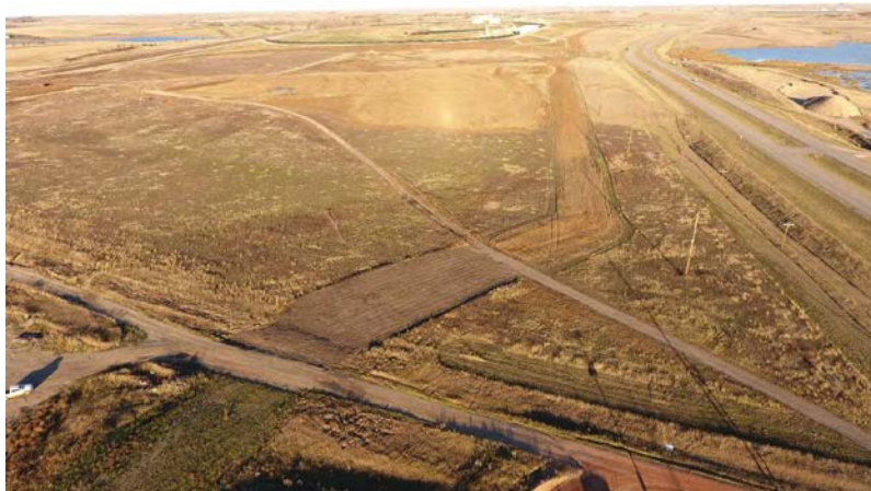
Photo 69: Station 346+95; Latitude: 48.32824925 Longitude: -102.268764722
