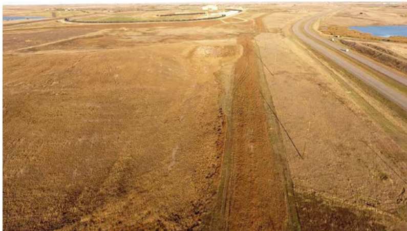
Photo 72: Station 357+40; Latitude: 48.328807944 Longitude: -102.264909083
