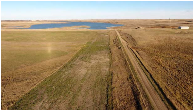
Photo 41: Station 242+80; Latitude: 48.312840083 Longitude: -102.293604889
