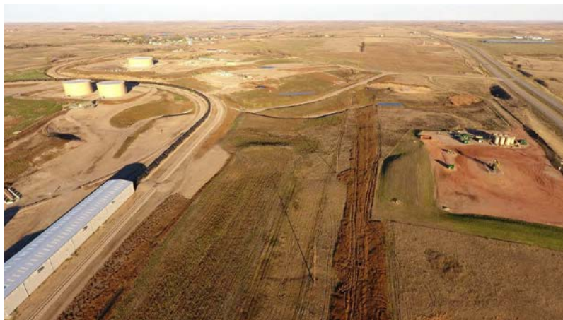
Photo 84: Station 391+05; Latitude: 48.330644667 Longitude: -102.251333
