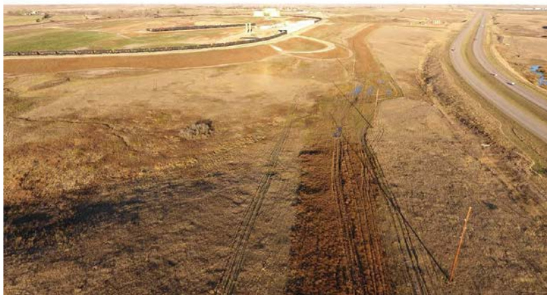
Photo 77: Station: 369+20; Latitude: 48.329699611 Longitude: -102.260198972
