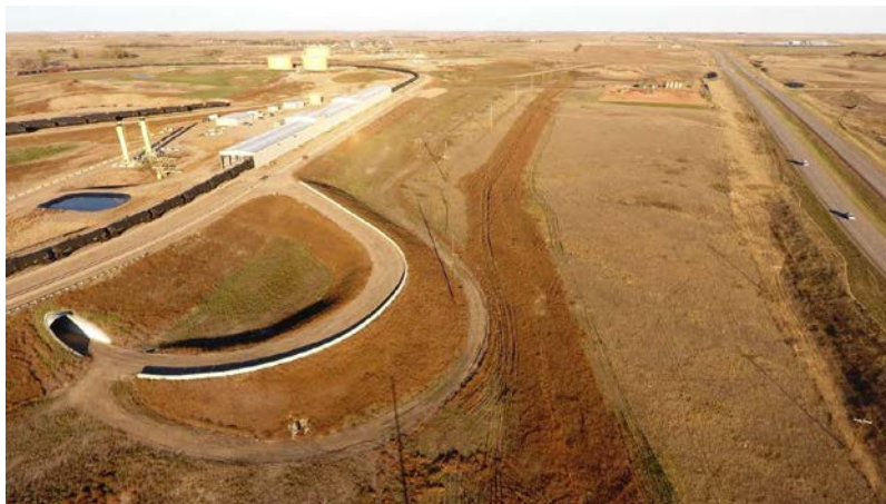
Photo 81: Station 380+00; Latitude: 48.330210944 Longitude: -102.255826028
