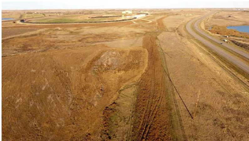
Photo 74: Station 362+00; Latitude: 48.329122778 Longitude: -102.263109028
