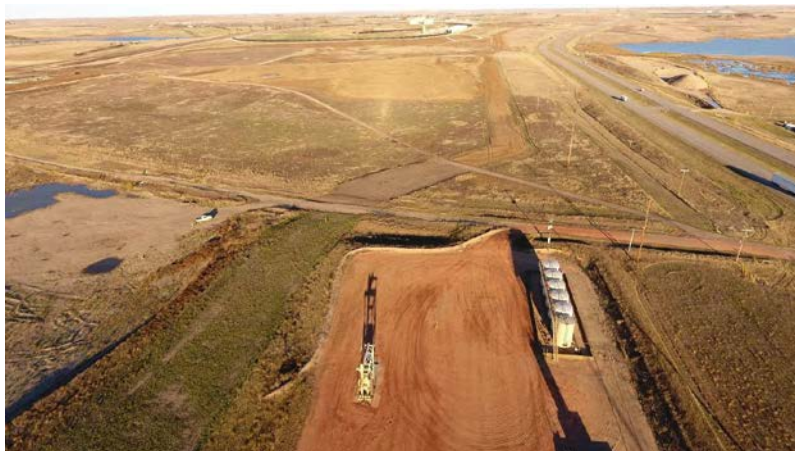
Photo 68: Station 343+00; Latitude: 48.328069694 Longitude: -102.270086556
