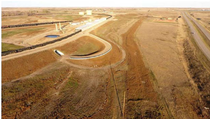
Photo 80: Station 378+10; Latitude: 48.330111611 Longitude: -102.256594861
