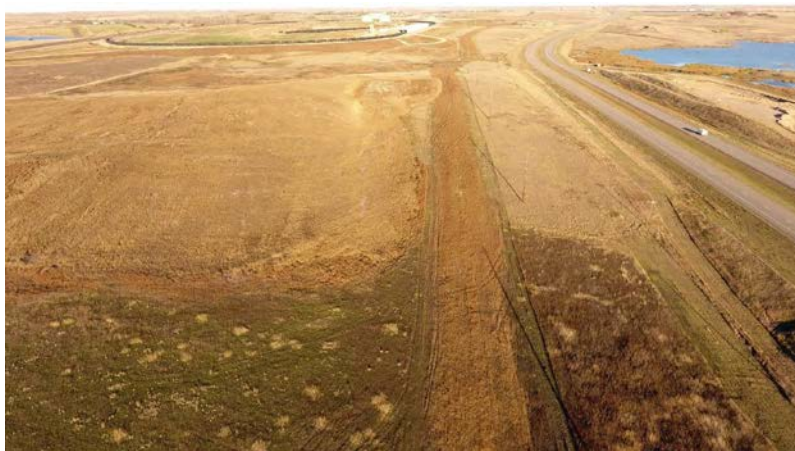
Photo 71: Station 355+20; Latitude: 48.328676083 Longitude: -102.265787667
