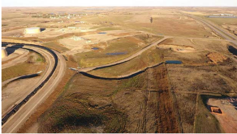
Photo 85: Station 397+50; Latitude: 48.3308205 Longitude: -102.248721833
