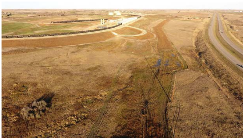
Photo 78: Station 372+15; Latitude: 48.329854722 Longitude: -102.258986056
