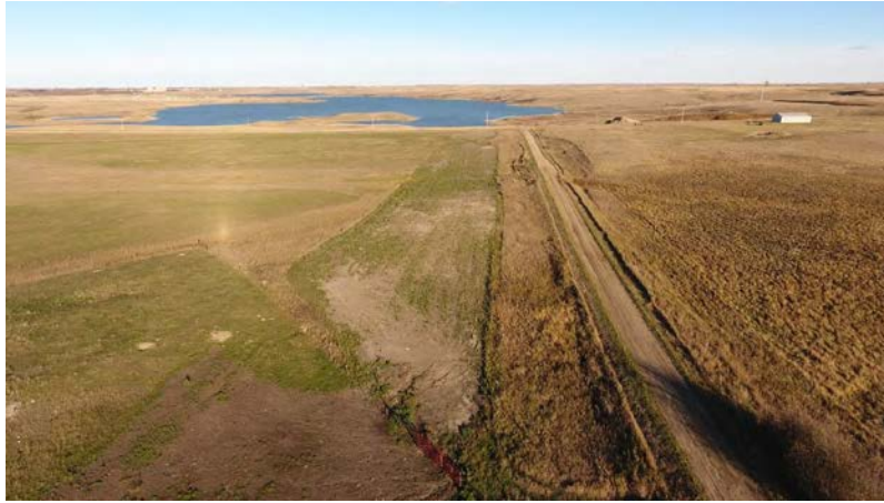
Photo 40: Station 241+10; Latitude: 48.312834167 Longitude: -102.294182278
