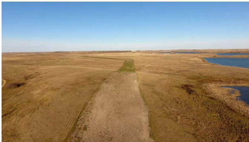
Photo 48: Station 280+50; Latitude: 48.319102194 Longitude: -102.28566225
