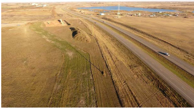
Photo 64: Station 332+10; Latitude: 48.32746350 Longitude: -102.274492694
