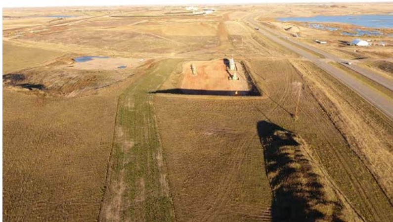
Photo 66: Station 337+95; Latitude: 48.327648939 Longitude: -102.272231806
