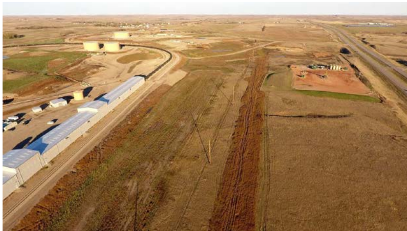
Photo 83: Station 386+95; Latitude: 48.330491028 Longitude: -102.253089889
