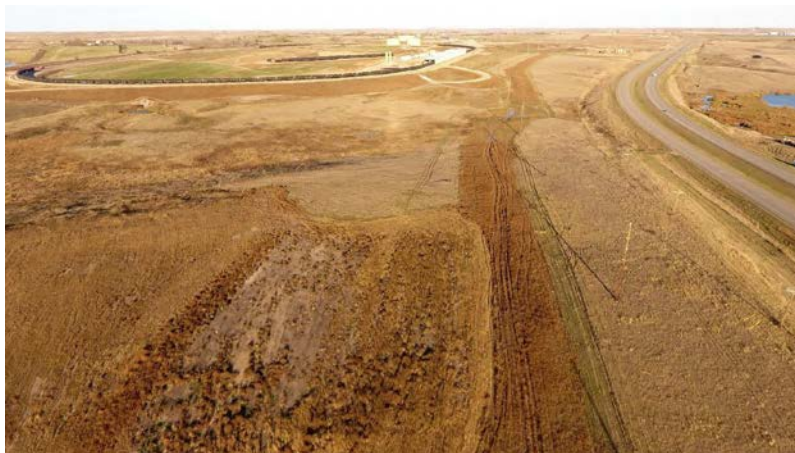
Photo 75: Station 364+45; Latitude: 48.329347833 Longitude: -102.262112472
