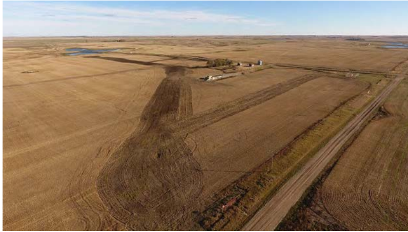
Photo 4: Station 43+80; Latitude: 48.3004863 Longitude: -102.3513947
