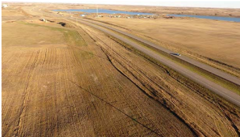
Photo 62: Station 325+95; Latitude: 48.327777472 Longitude: -102.277087417
