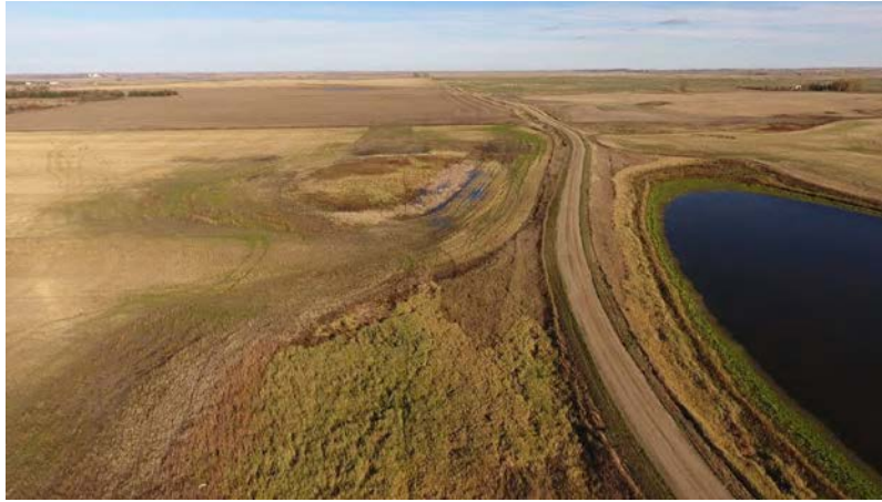
Photo 13: Station 68+90; Latitude: 48.2990770 Longitude: -102.3420824
