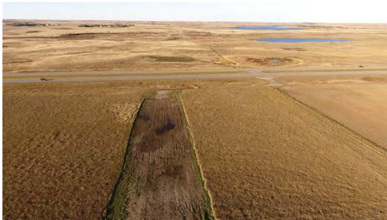
Photo 59: Station 309+53; Latitude: 48.324779389 Longitude: -102.279903639
