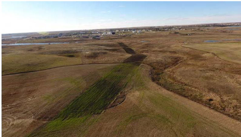
Photo 2: Station 37+00; Latitude: 48.3013947 Longitude: -102.3538208
