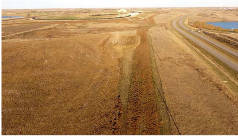
Photo 73: Station 358+90; Latitude: 48.328886056 Longitude: -102.264338278
