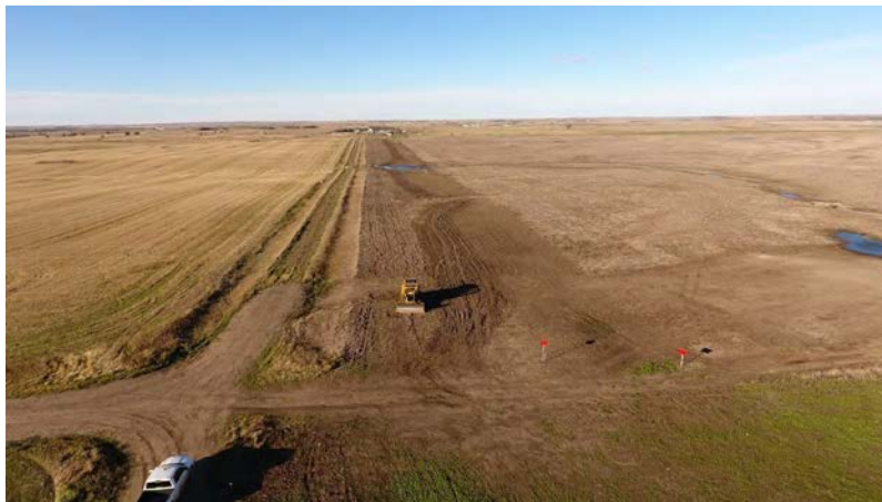
Photo 21: Station 150+90; Latitude: 48.297832028 Longitude: -102.309852722
