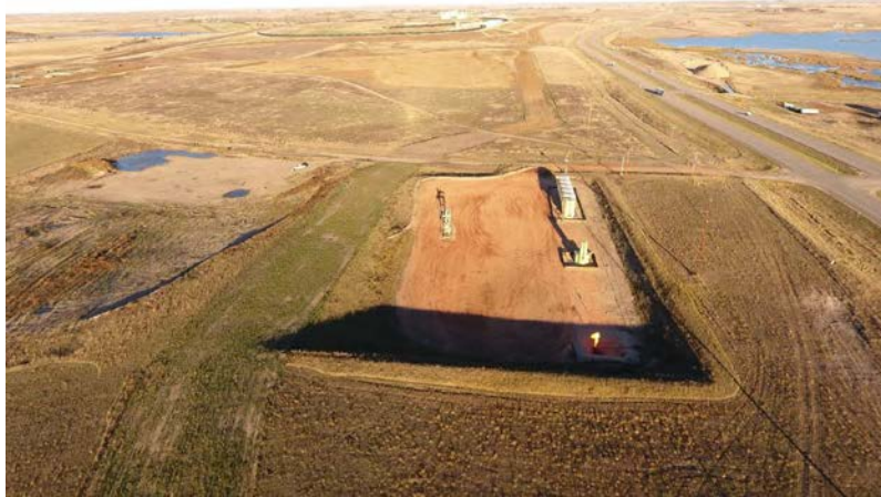
Photo 67: Station 340+85; Latitude: 48.327898444 Longitude: -102.271034717
