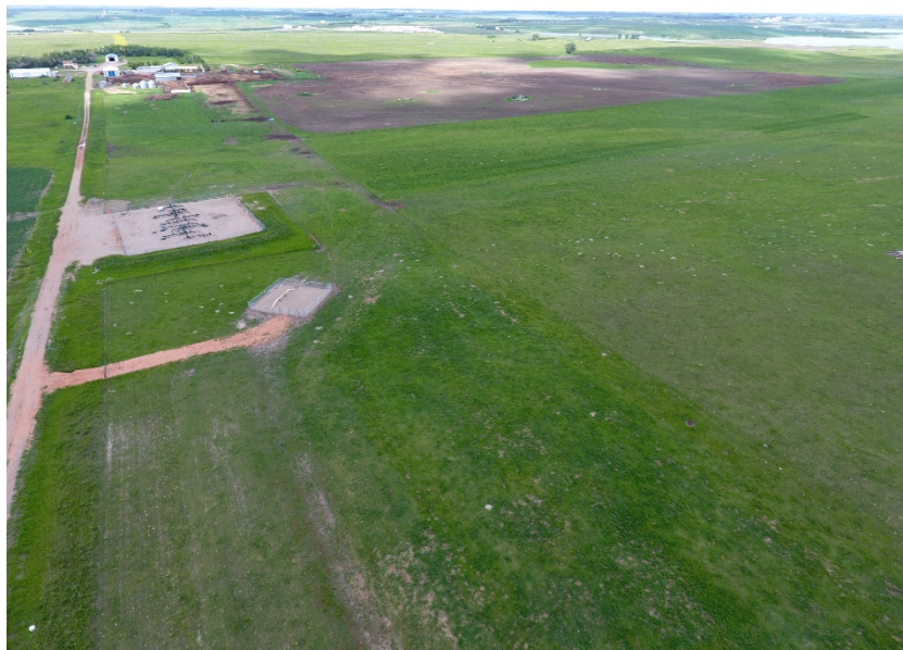
Location 28 (48.306168, -102.309608) Vegetation established to match adjacent conditions
