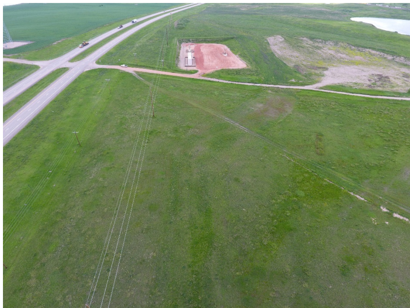
Location 10 (48.32872, -102.265045) Well established and matching existing conditions
