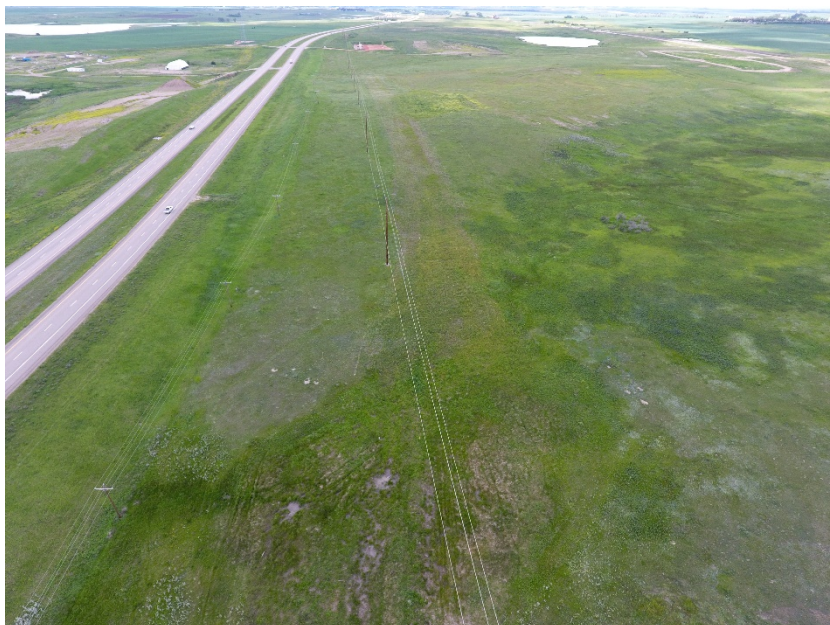
Location 8 (48.330128, -102.255562) Well established and matching existing conditions
