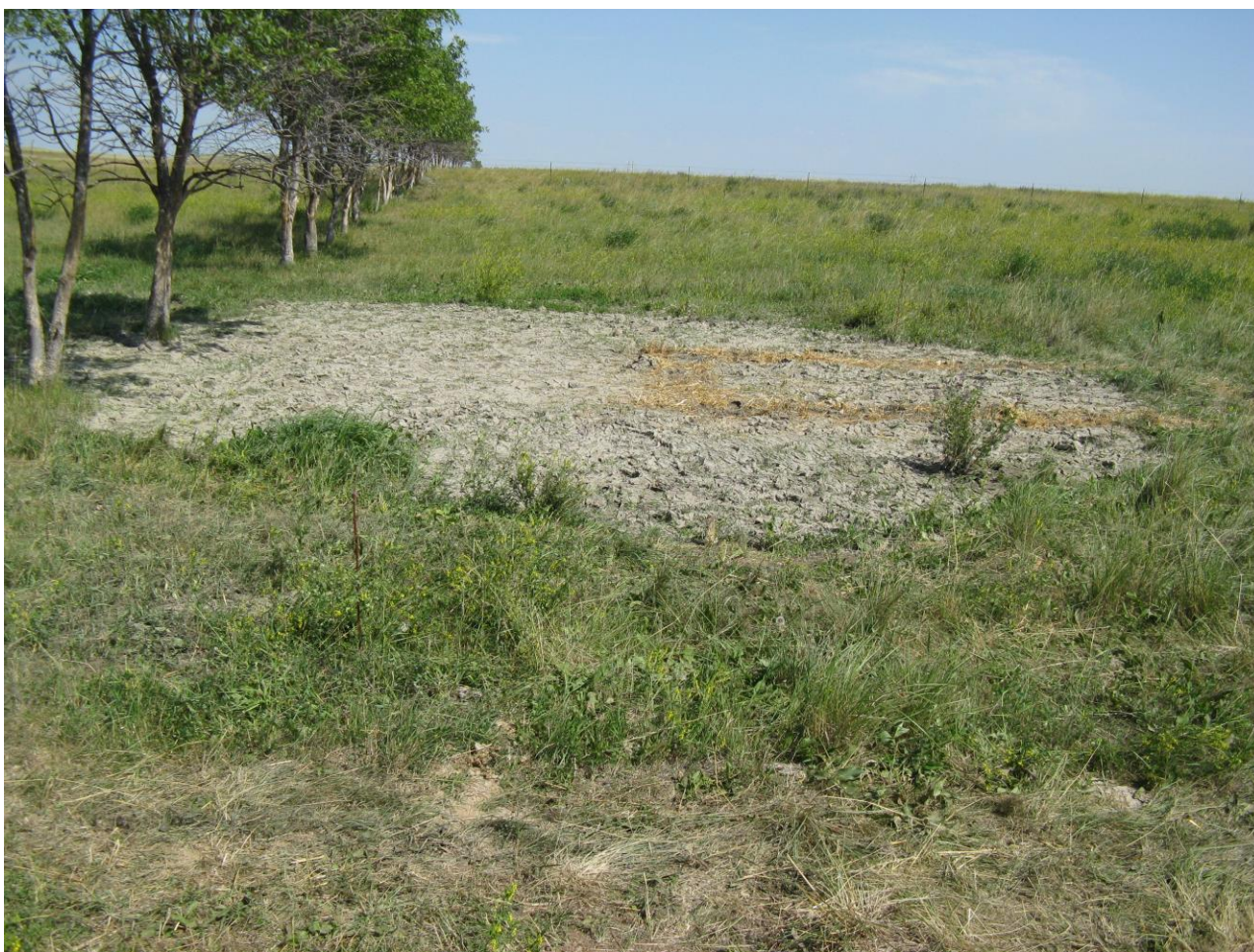
Figure 2. Typical Surface Expression of a Frac-Out
