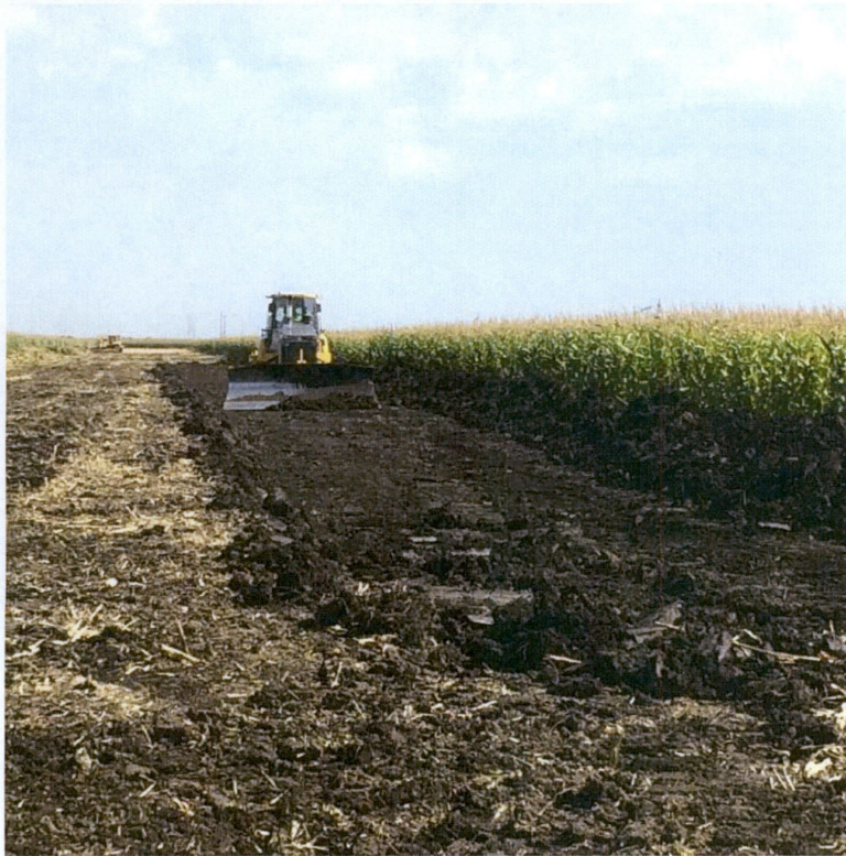
Photo 3: Topsoil scraping and removal depth.
