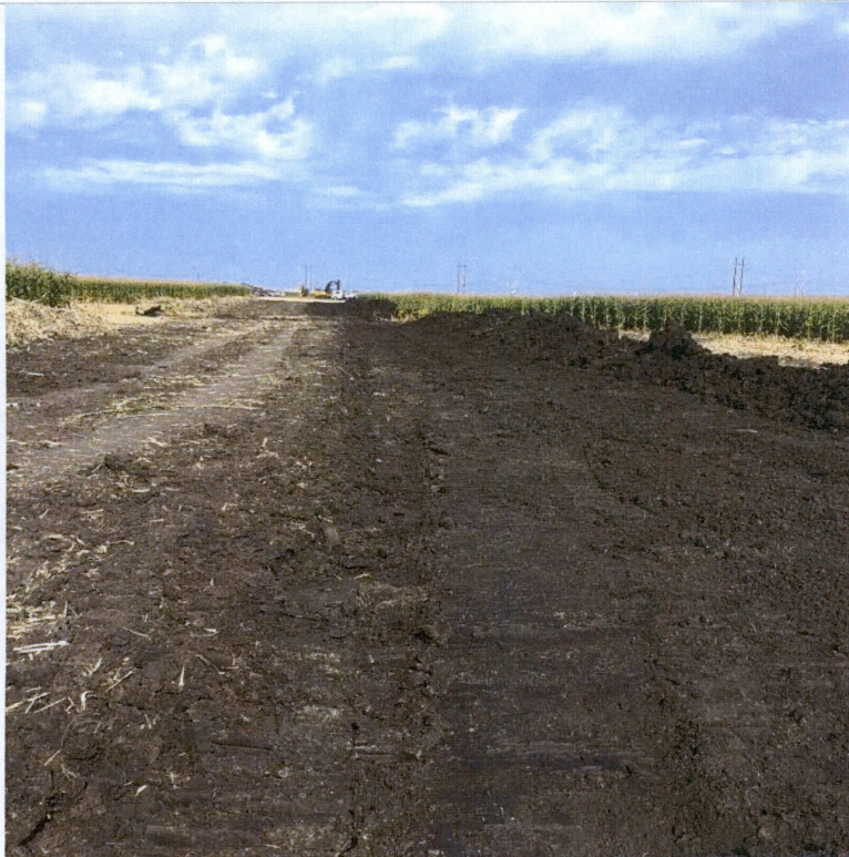
Photo 5: Topsoil placement at construction easement edge.
