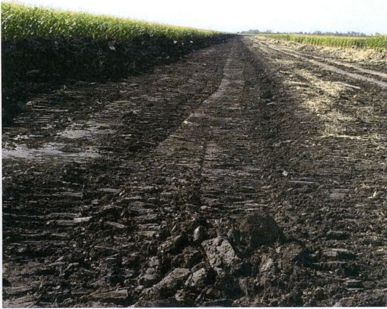
Photo 6: Topsoil placement at construction easement edge.
