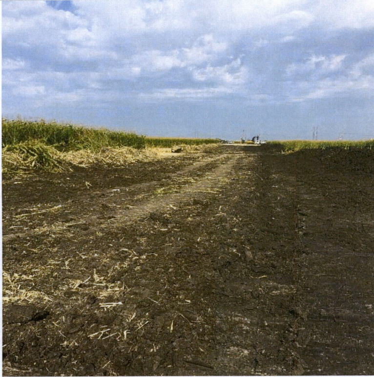
Photo 4: View of easement; topsoil segregation in progress.
