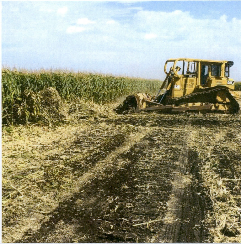
Photo 1: Topsoil scraping to the construction easement edge.
